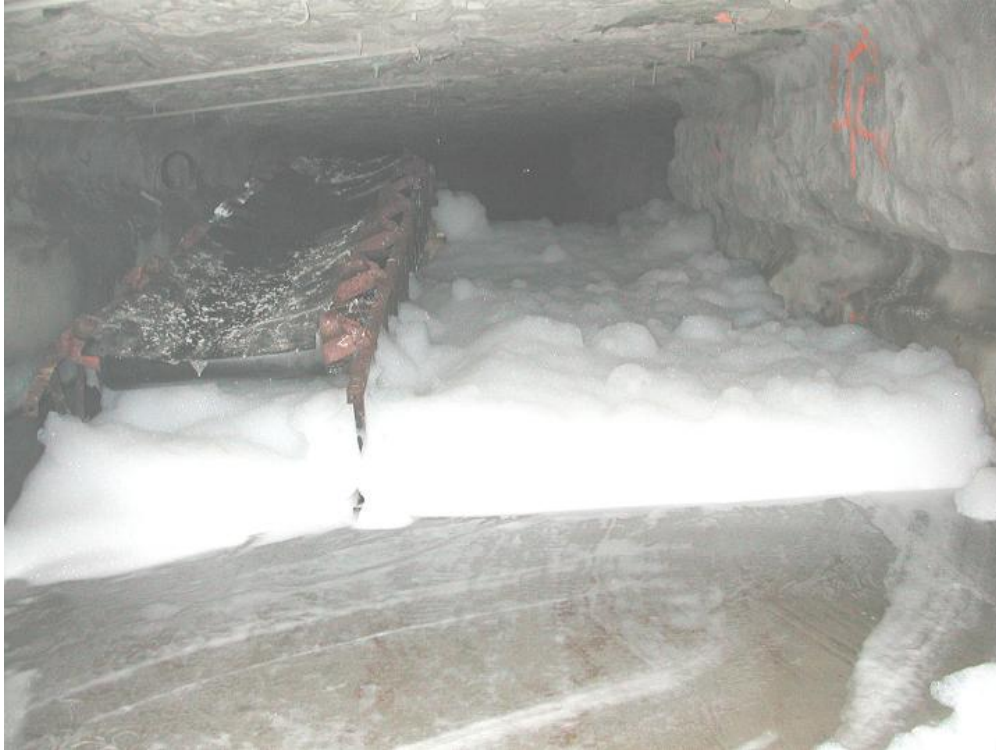
Figure 11. Conveyor belt structure in A drift.
