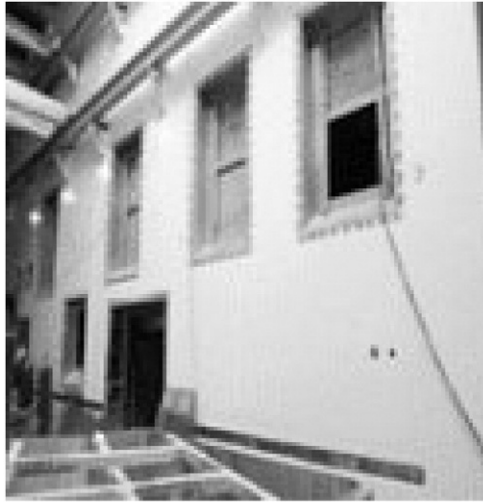
Advanced Mixed Waste Processing Facility Project, January 1, 2002 (Operators' windows): Operators will open waste containers and sort the contents standing behind these finished windows, using remote BROKK robotic arms and overhead power manipulators.
