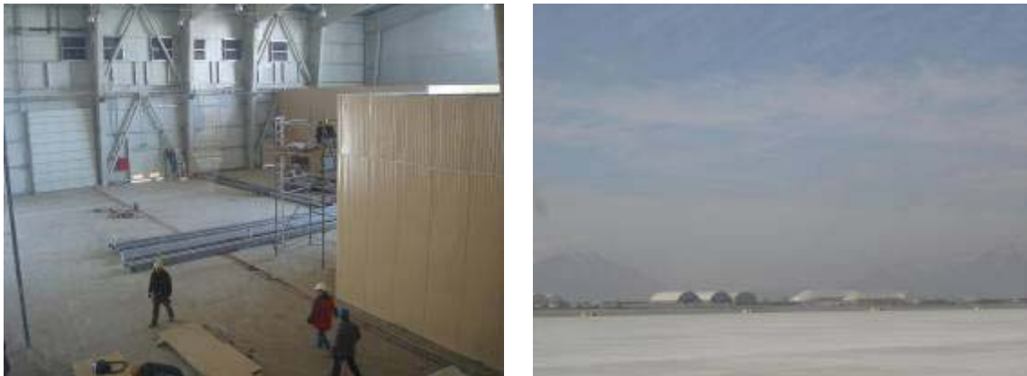
Figure 5. KAIA Hangar (left) and Taxiway (right)
