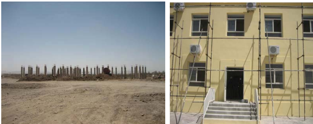
Figure 7. Dining Facility (left) and Operation Group Headquarters (right)
