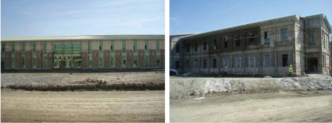
Figure 4. Northside Cantonment Area Office Building (left) and Barracks (right)
