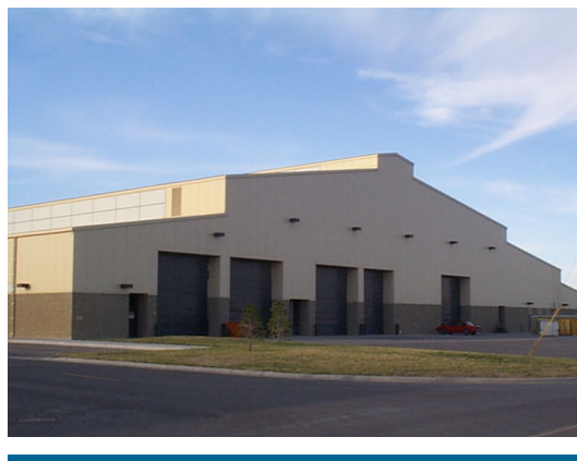
An example of an industrial building in which the visual emphasis has been placed on the service entrances.
