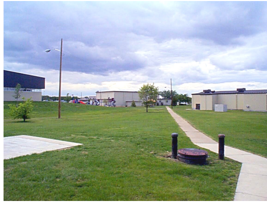
The area behind Buildings 1145, 1150, 1154, and 1156 lacks landscape treatment to help define and create positive outdoor space.
