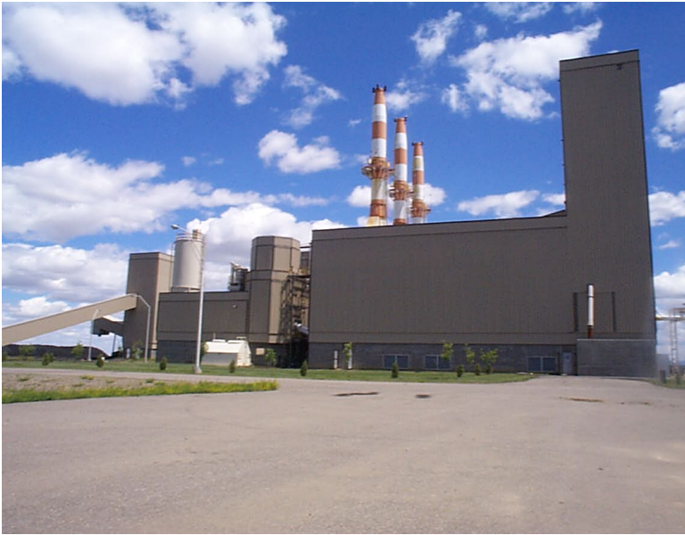
Central Heat Plant
