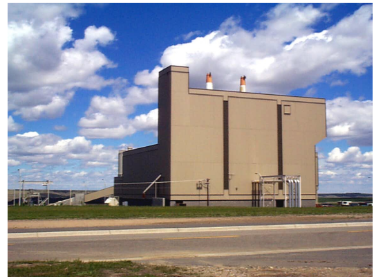
Building 82110, Heat Plant.
