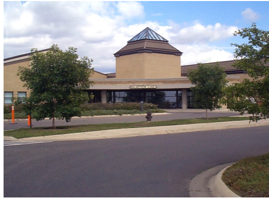
Building 2040, Medical Clinic.
