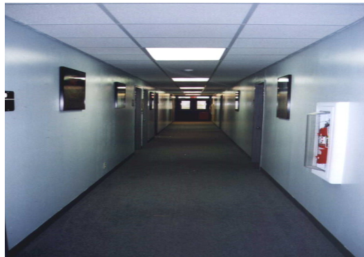
Lights parallel to a long, narrow corridor.
