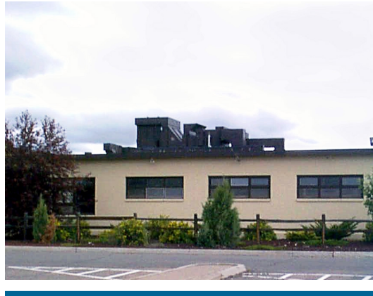
All roof mounted equipment shall be screened with roof materials used elsewhere on the building.
