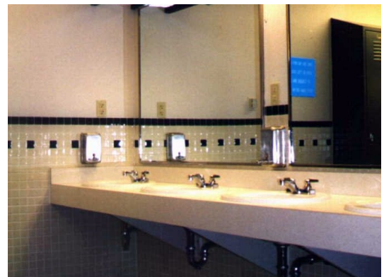
Ceramic tile in restroom.
