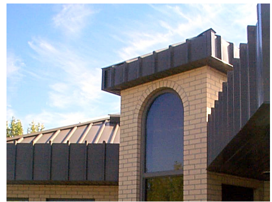
Exterior design theme for the South Gate Visual District should follow the Visitor Center, Building 192.
