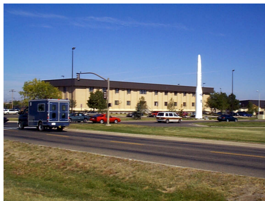
Building 1191, typical of the Administration Visual District.
