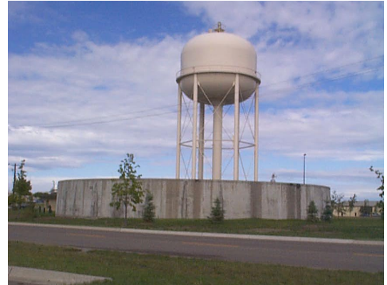
Water Storage Tank.
