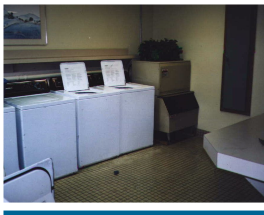
Ceramic tile floor in laundry room.
