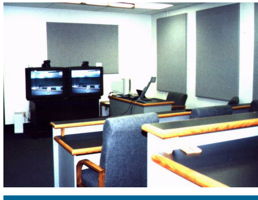
Acoustic fabric panels on walls.
