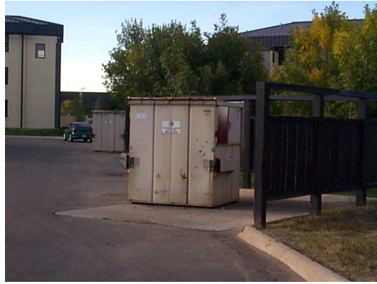
Dumpsters need better screening or relocation.
