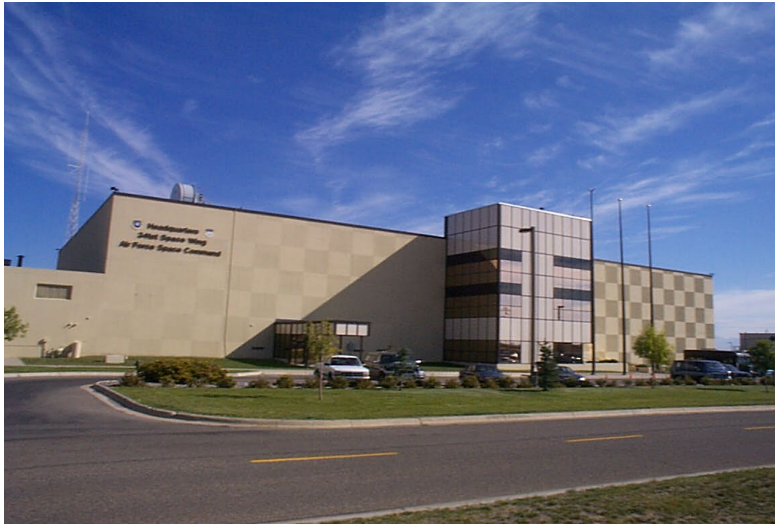
Radio Frequency Transmitters at Building 500
