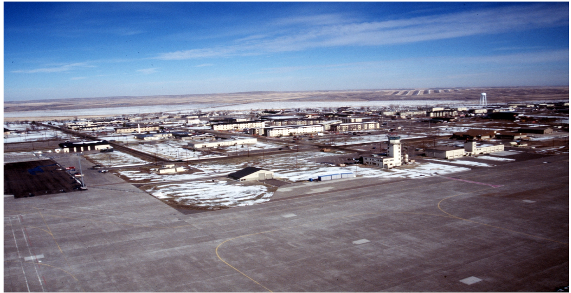
Relatively Flat Terrain on Main Base
