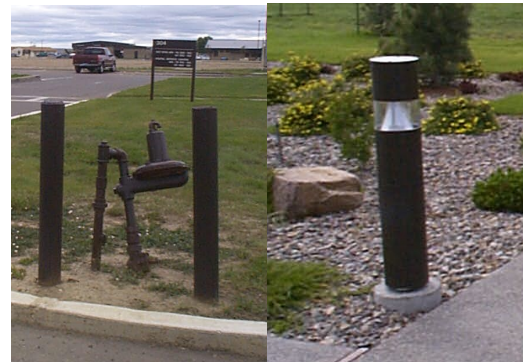
Left: Typical unlit bollards which should be utilized for protecting utility structures.
