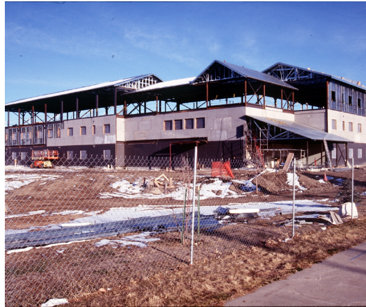
New dormitory construction at Malmstrom AFB.
