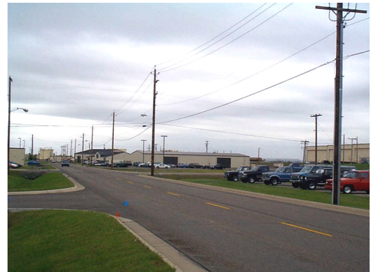
Utility poles along Flightline Drive.
