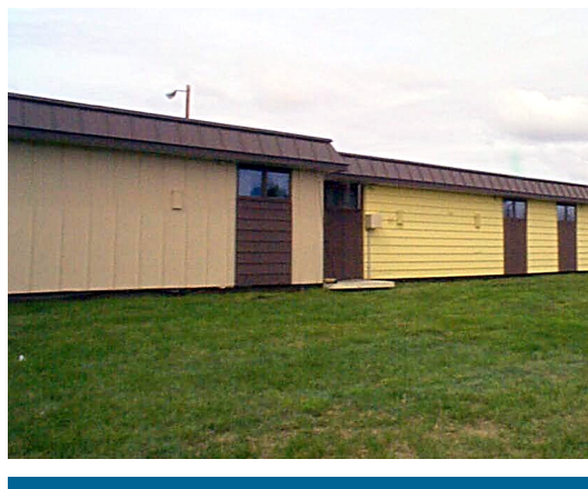
Siding applied vertically and horizontally.
