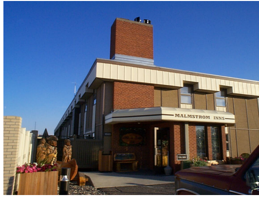
The Malmstrom Inn is not consistent with installation exterior standards.
