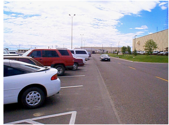
No functional separation of parking and roadway.
