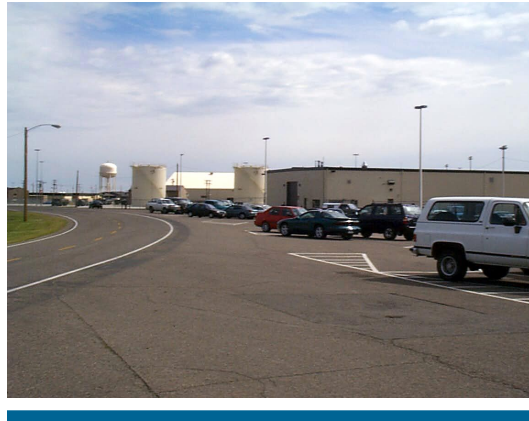
Parking lot which fronts directly onto Perimeter Road.
