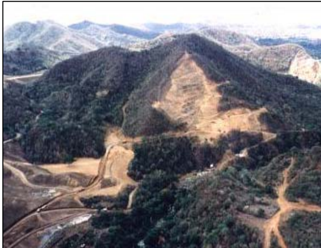
-Portugues Dam (under construction), Puerto Rico
