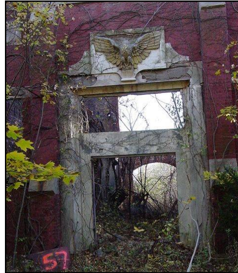
Drill Hall/Gymnasium, built 1909. Credit: Tetra Tech EC, Inc.
