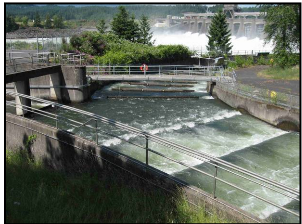
Outlet gates (background) and fish ladder (foreground) at the Bonneville Lock and Dam, Oregon
