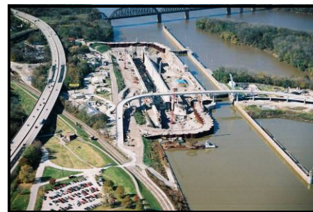
McAlpine Locks and Dam
