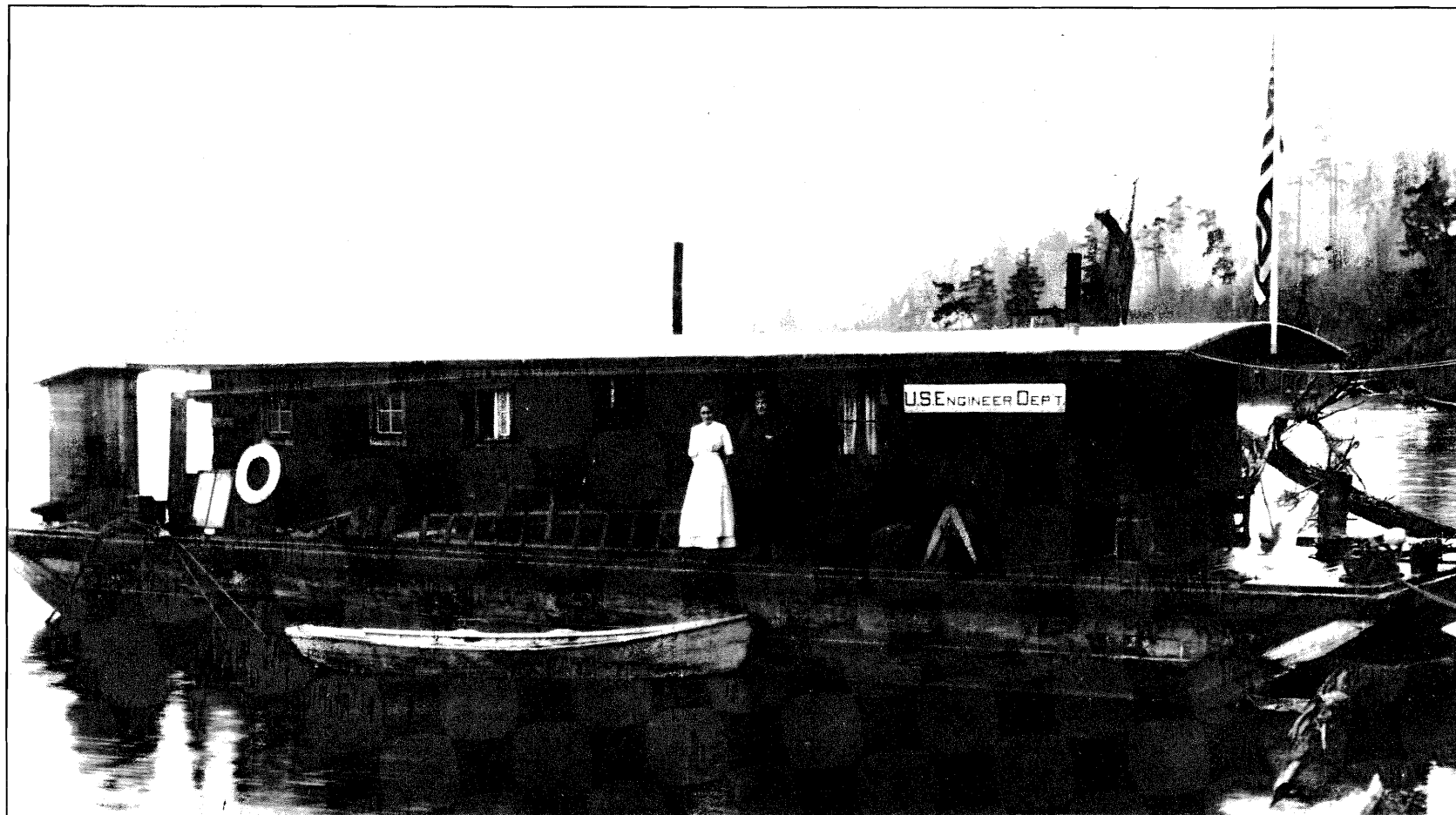
Army Engineer floating plant, Scow "D," 3 December 1914.
