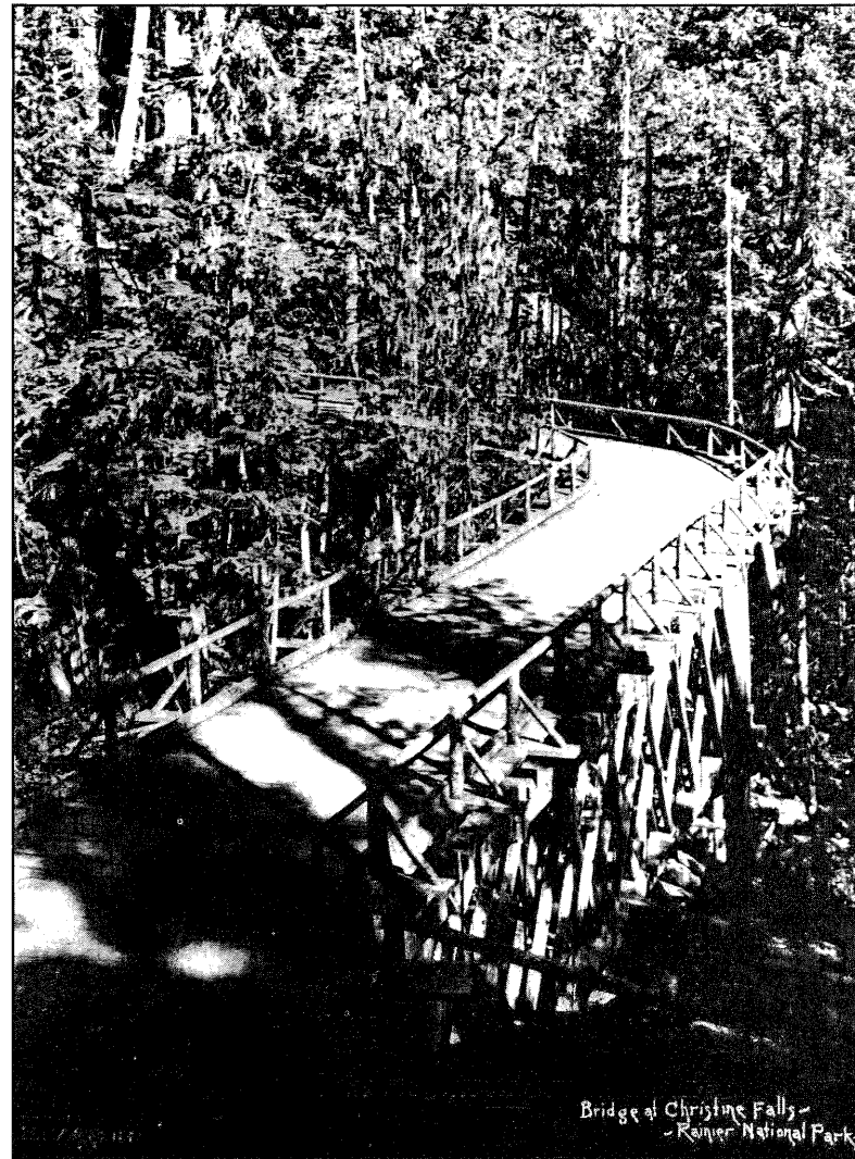
Bridge at Christine Falls - - Rainier National Park One hundred-foot span deck Howe truss bridge across Van Trump Creek, in front of Christine Falls, Mount Rainier National Park. One hundred feet to bottom of canyon. Photograph from Annual Report, June 30, 1909.
