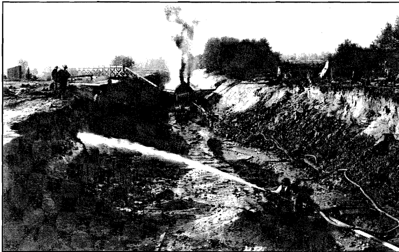
Excavation by water blasting, Lake Washington Ship Canal. Asahel Curtis photo, ca. 1914.
