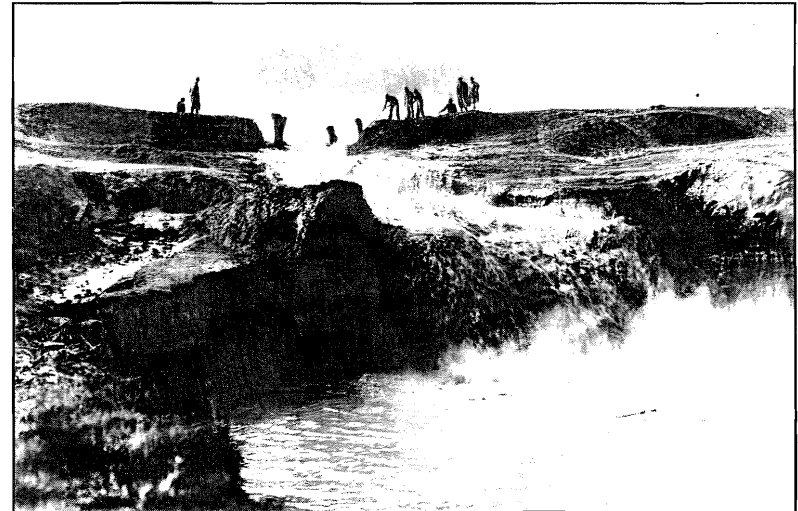
"...the waters ate their way into the earthen cofferdam, and in a few minutes the flow was roaring with the sound of a cataract." Breaching the cofferdam, Lake Washington Ship Canal, ca. 1916.
