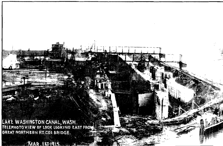
Looking east from Great Northern Railroad bridge
