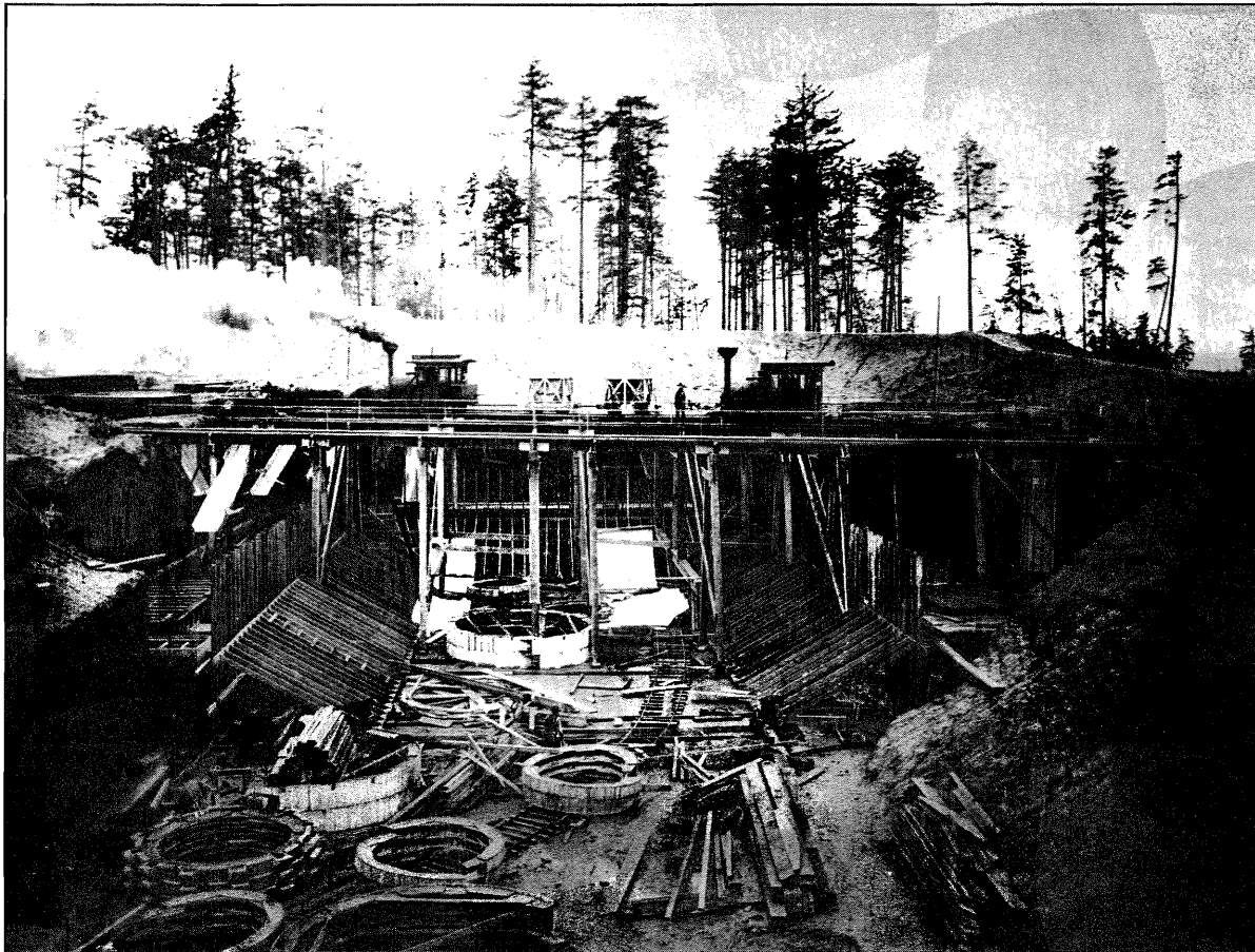
Construction of 12-inch mortar battery, Fort Worden.
