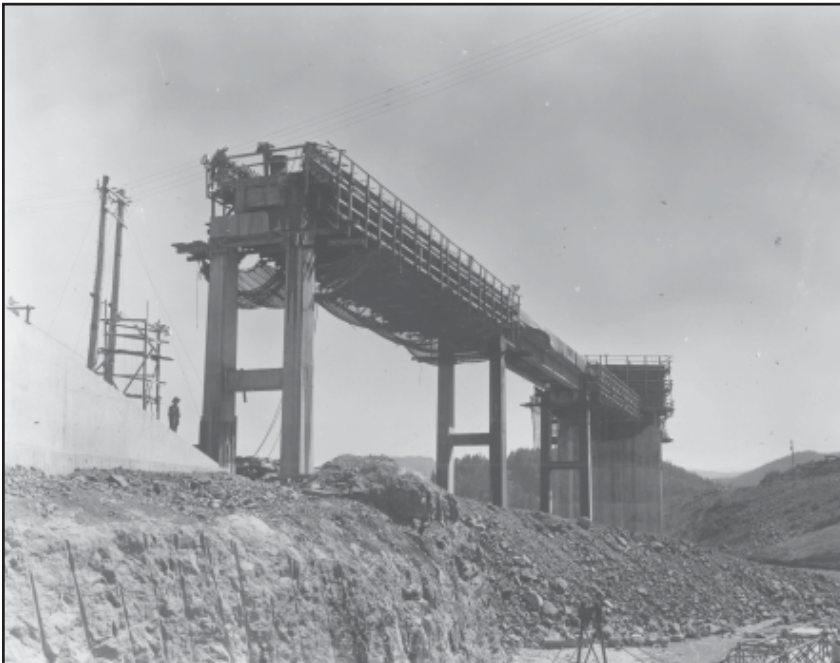
Howard Hanson Dam Construction
