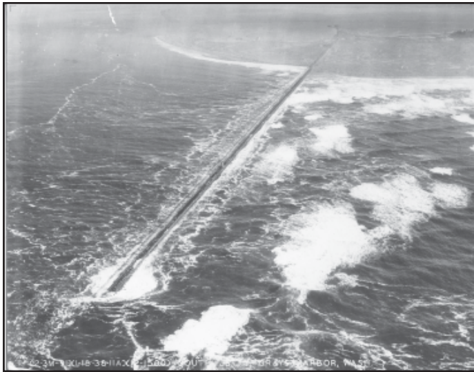
Grays Harbor, South Jetty
