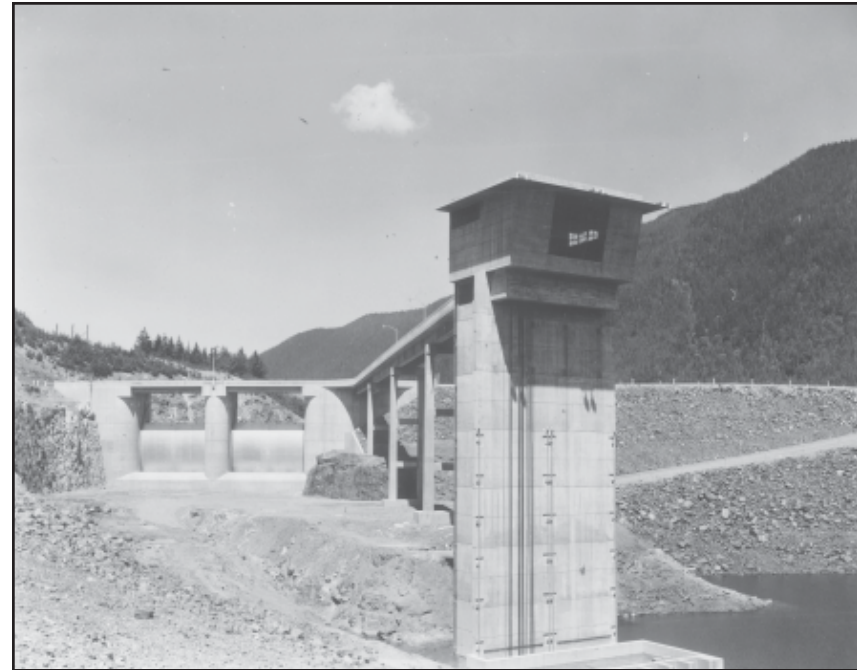
Howard Hanson Dam Construction
