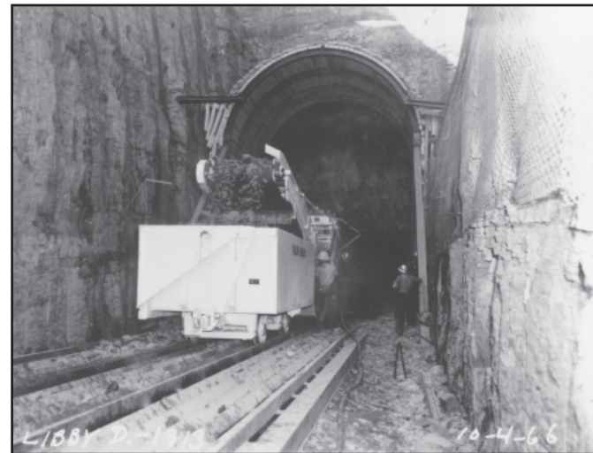
Great Northern Railway Tunnel Construction
