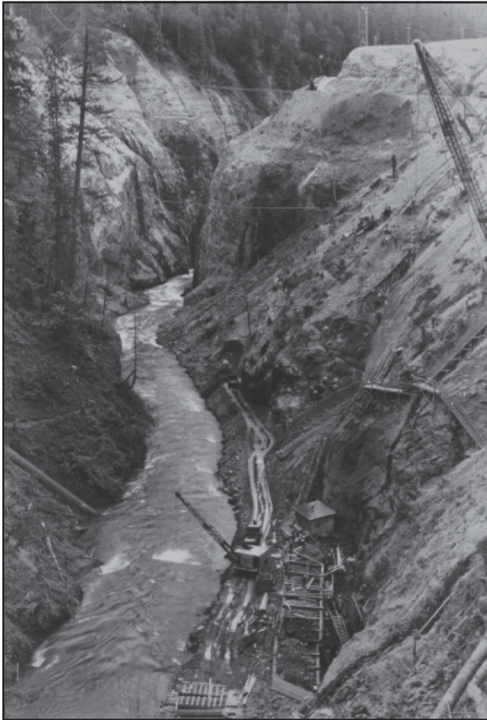
Mud Mountain Dam - Canyon Damsite 15 May 1940
