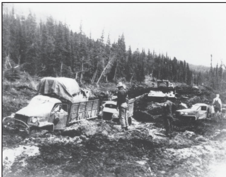
Alaska Canada Highway Construction, 1942
