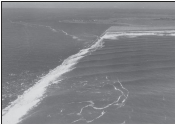
Grays Harbor, South Jetty Deterioration 30 January 1962
