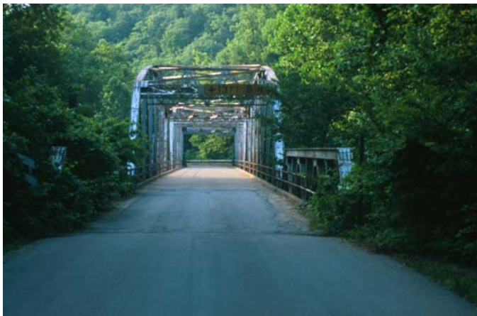
The Devil's Elbow Bridge across the Big Piney River attracts approximately 145,000 visitors a year. As part of the rehabilitation project, the county will locate signage to help direct visitors to the bridge.
