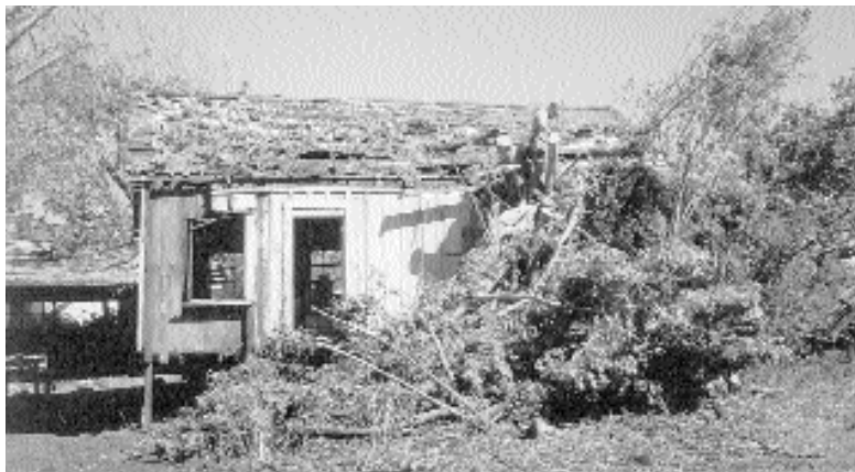
Bay View, Kalaupapa National Historical Park. National Park Service crew removing overgrown vegetation at the beginning of the rehabilitation project. Photo by Hunter Glidewell.
