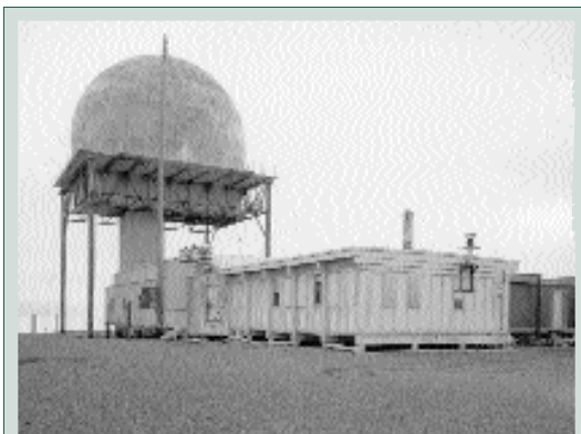
The Distant Early Warning Line Station, Bullen Point, AK, is one in a series of stations of the late 1950s and 1960s located across Alaska and Canada. These stations monitored enemy planes over the North Pole by providing for radar equipment to be located in the radome, which opened and scanned the skies. The Alaska State Historic Preservation Office worked with the Department of Defense in documenting and evaluating these important historic places from the Cold War period. Historic American Buildings Survey photo.
