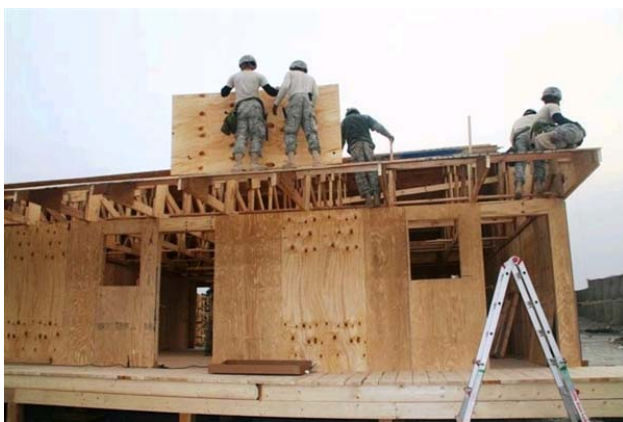
Soldiers from 1st Platoon, 76th Engineer Company, Fort Knox, KY, build a hut in Jalalabad, Afghanistan. ( Army photo )
