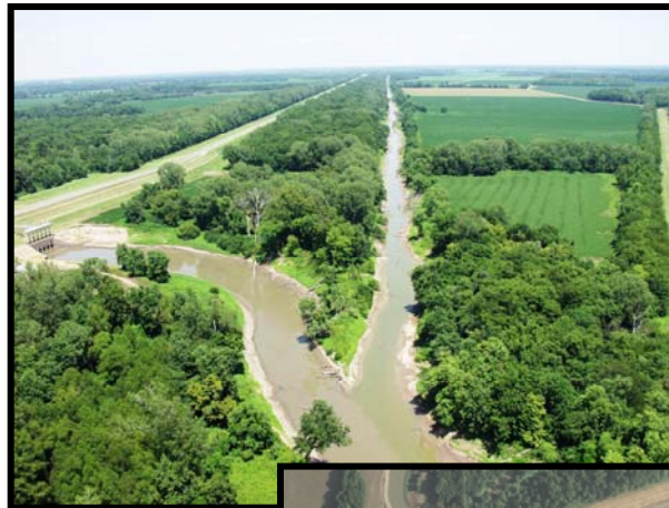
New Madrid, MO Floodway Outlet
