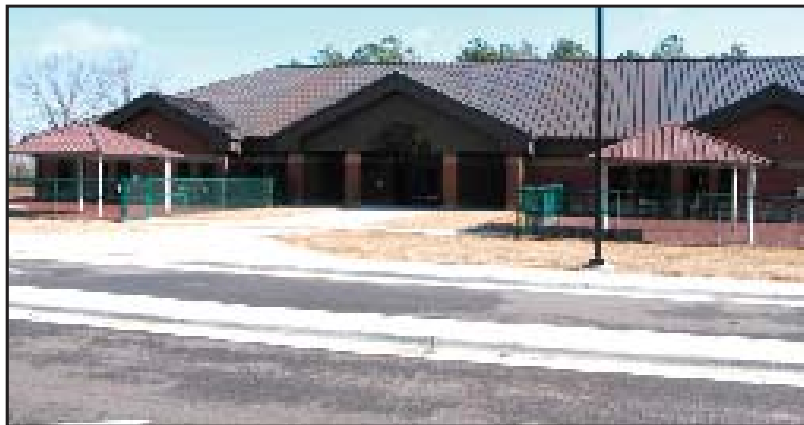
The completed Child Development Center at Little Rock Air Force Base in February.
