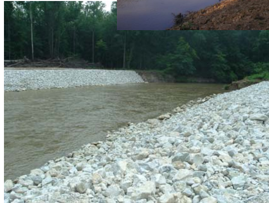
Completion of Channel Stabilization Weir CW-6
