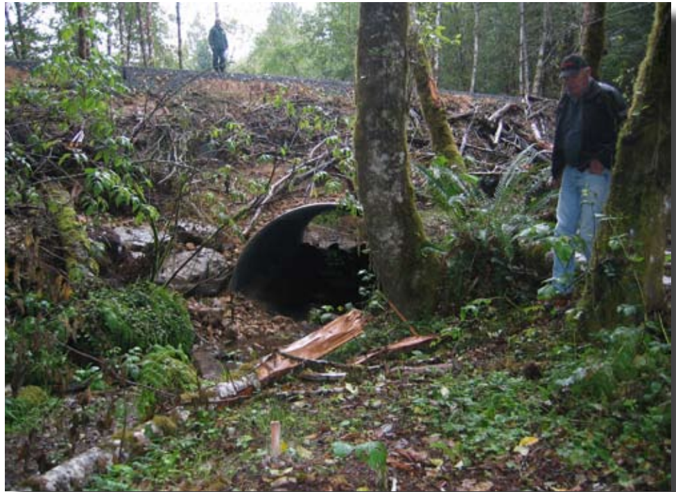
Figure 7.11—Clearing debris scattered for erosion control.
