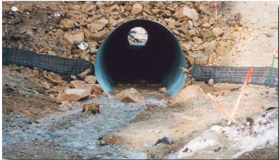
Figure 7.22—Typical silt-fence installation.
