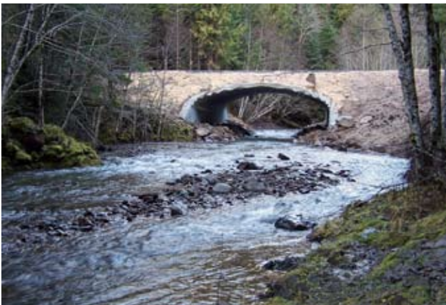
Figure 7.6—Multiplate open-bottom box.
