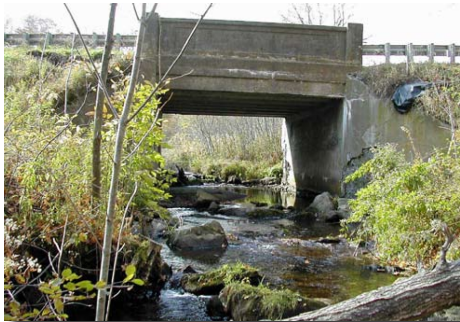
Figure 1.22—This box culvert has a concrete floor and no shallow edges for crawling-species passage. Photo: Scott Jackson, University of Massachusetts.
