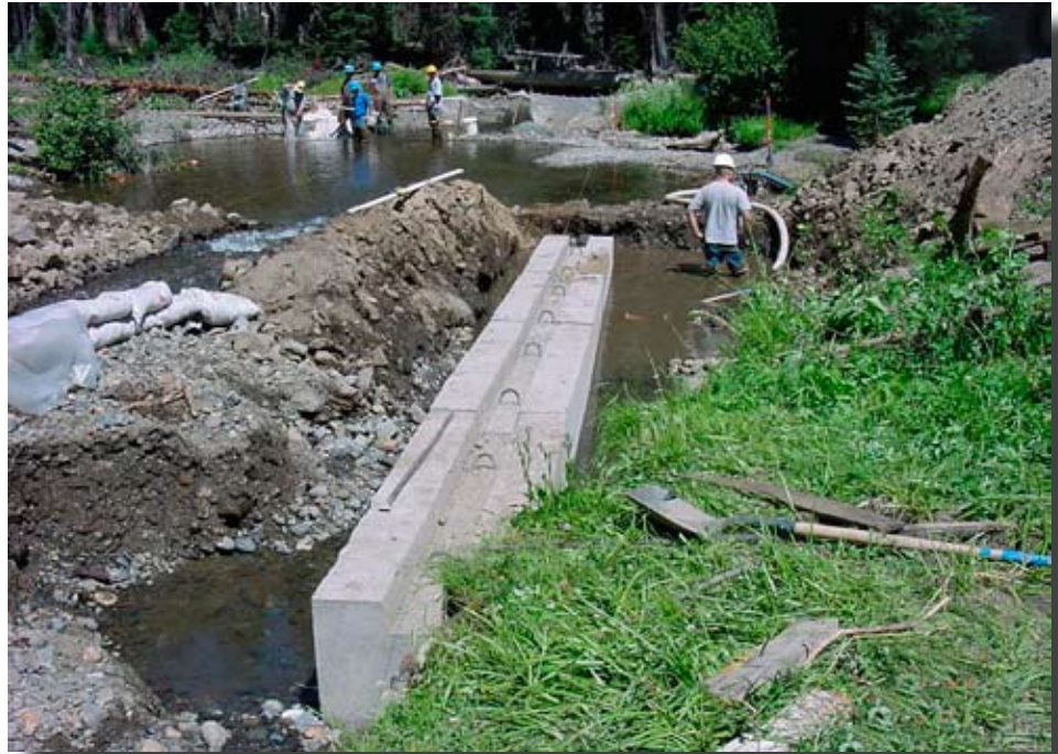
Figure G.10—South Fork Desolation Creek looking upstream. The crew captured fish trapped within the construction area as the foundation trenches were dewatered.
