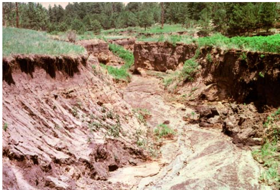
Figure 4.6—Channel widening after recent incision, eastern Colorado.
