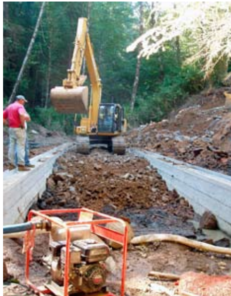
Figure 8.13—Machine placing stream-simulation material. It took 4 days to place 600-cubic yards.
