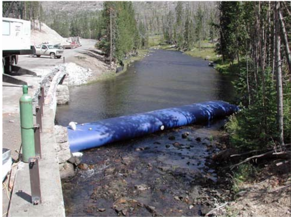
Figure 2.6—Isolating the construction area at a bridge reconstruction site in Yellowstone National Park. Photo: Dan Rhodes, National Park Service.
