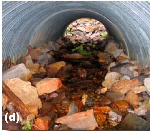
Figure 6.18—(a) Design site plan.(b) Design longitudinal profile.(c) Realigned channel at outlet.(d) Looking downstream through the finished stream simulation culvert. (Design by Robert Gubernick, Tongass National Forest, and Chinook Engineering.)
