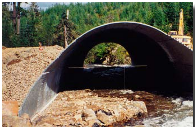
Figure 7.5—Multiplate open-bottom pipe arch.
