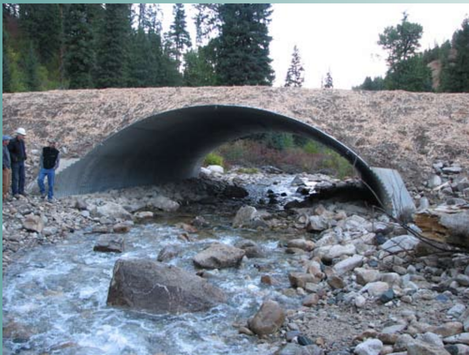
Figure 3.1—Roaring River crossing site before-and-after culvert replacement in 2007, Boise National Forest, Idaho.
