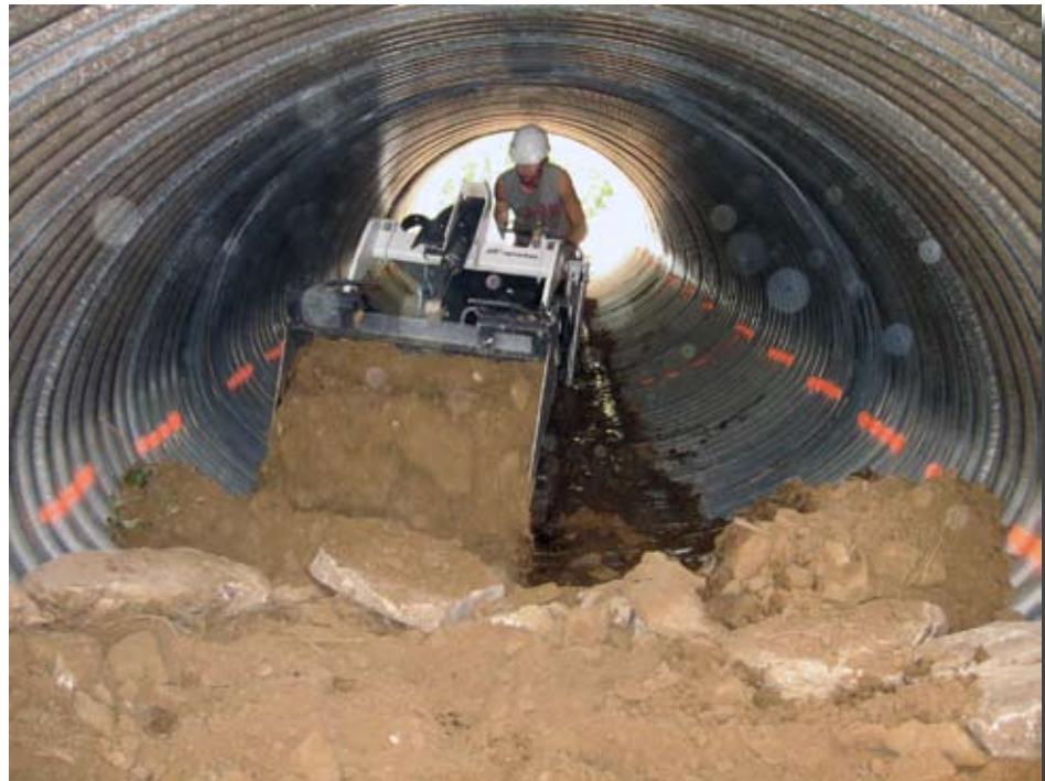
Figure 8.15—Bobcat placing bed material to marked elevation.
