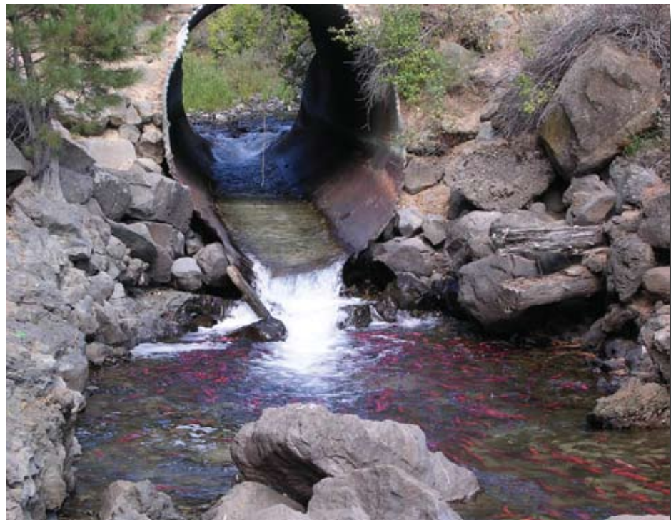
Figure 3. Culvert on the Boise National Forest prevents migration of kokanee salmon.
