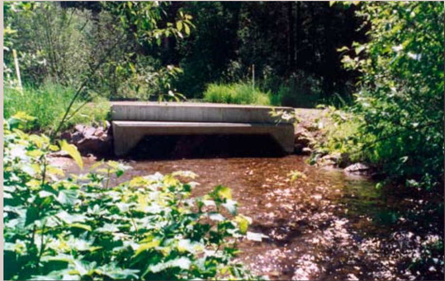
Figure 4.8—Brewster Creek road replacement box culvert, filled to 85 percent of its rise after 1 year.
