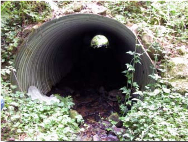
Figure 7.2—1-piece corrugated metal pipe (embedded).
