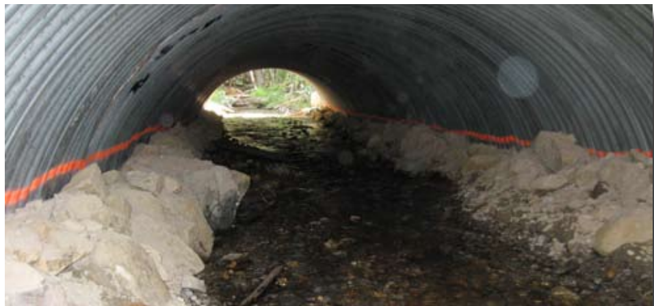
Figure 7.16—Newly constructed (2006) stream-simulation channel and banks, Surveyor Creek, Lolo National Forest, ID. The top of the bank is at bankfull elevation, indicated by the painted line. Note the transition between natural banks outside and constructed banks inside the culvert.
