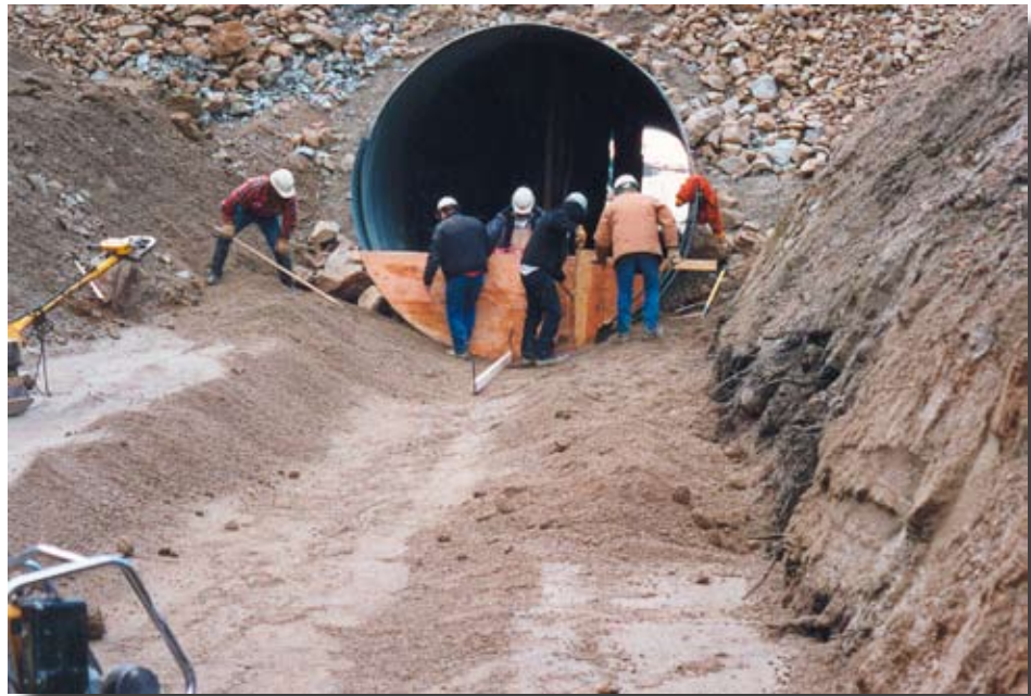
Figure 7.9—Shaping culvert bedding.
