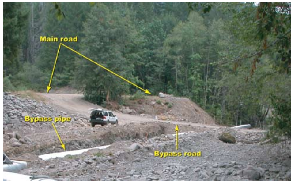
Figure 7.12—Typical construction site traffic bypass.
