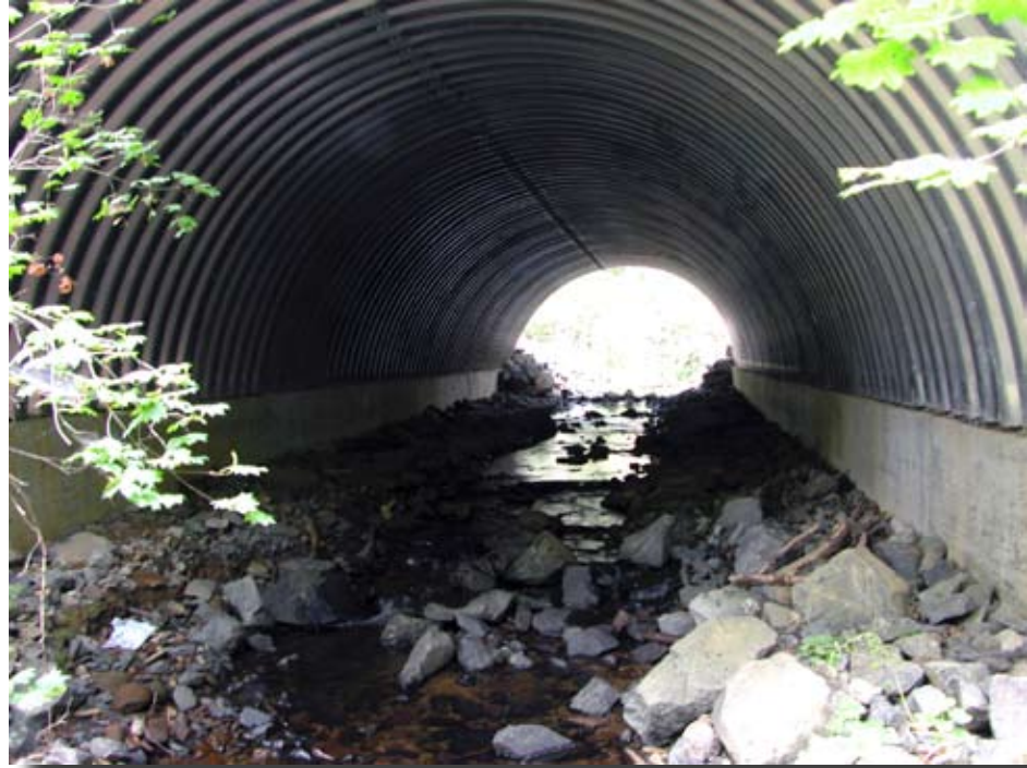
Figure 8.3—Results of a survey error. Footings were constructed 2 feet higher than the designed location because of a construction survey error. Always doublecheck surveys!
