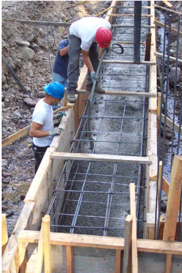
Figure 8.10—Concrete forms and reinforcing during concrete pour.
