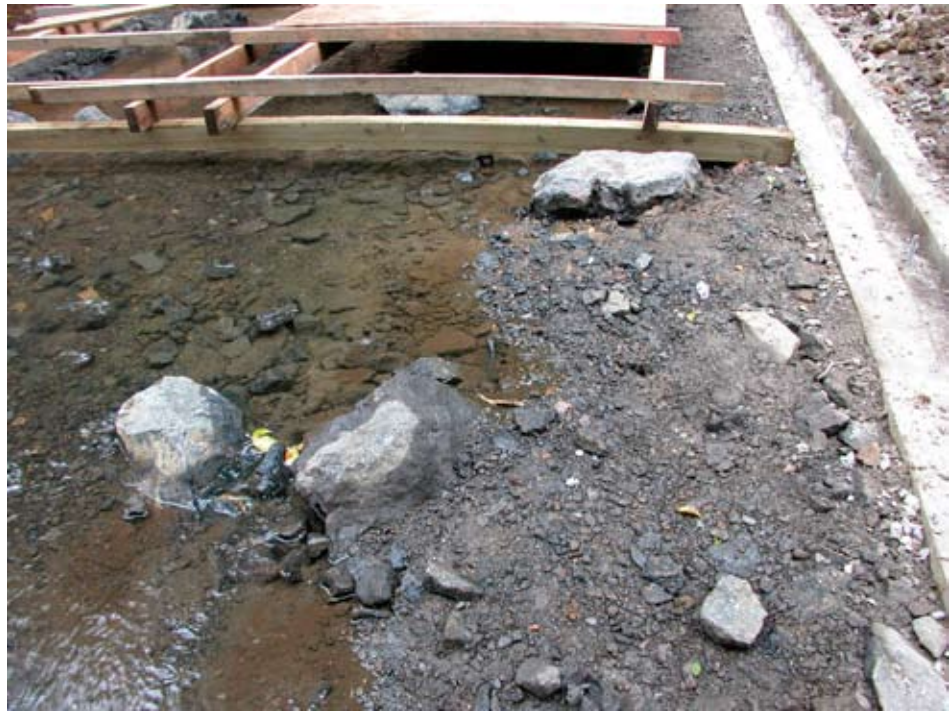
Figure 8.14—Newly constructed stream-simulation bed for a bottomless arch. The stream-simulation bed material is manufactured rock from a commercial source. Footing backfill and stream-simulation bed material were backfilled and compacted at the same time. Placing the stream-simulation bed is much easier before the structure is in place.
