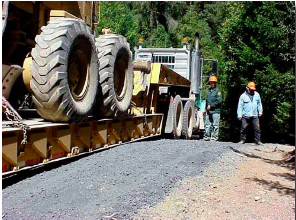
Figure 8.19—The grade change at this dip is too severe to accommodate a lowboy, which has high-centered on top of the dip..
