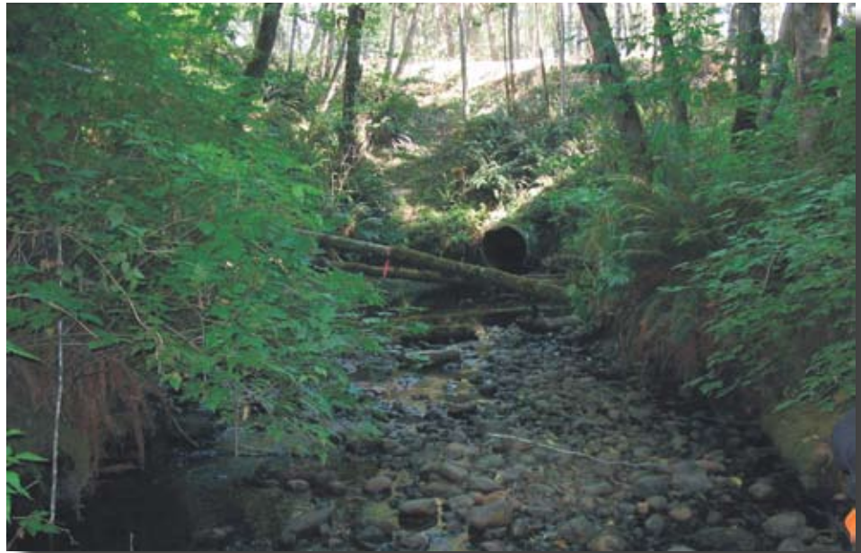
Figure E.6—The culvert outlet and the upper segment of the reference-reach channel at the Schafer Creek tributary. Note the perch of the culvert outlet and its size relative to the channel.
