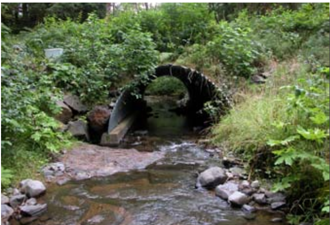
Figure 7.4—1-piece open-bottom arch.
