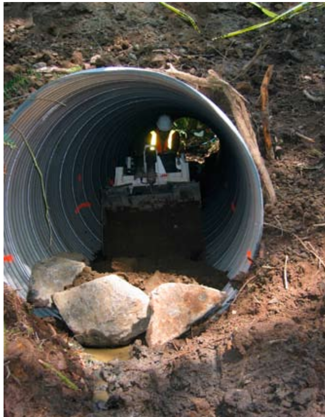
Figure 7.13—Hand labor walk-behind equipment.
