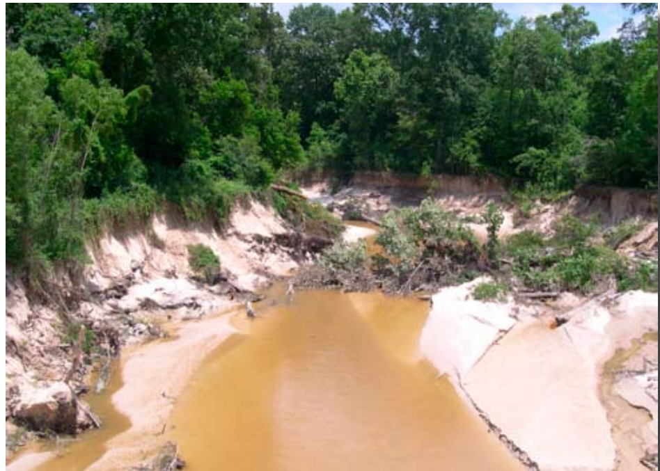
Figure 5.18—Major channel instability occurring on the Homochitto River, MS. Bank erosion and widening follow channel incision on this fine-grained channel.
