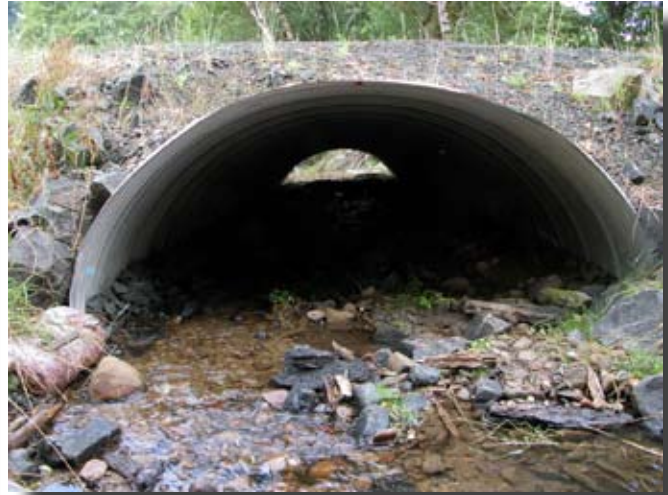
Figure 7.3—1-piece corrugated metal pipe arch (embedded).
