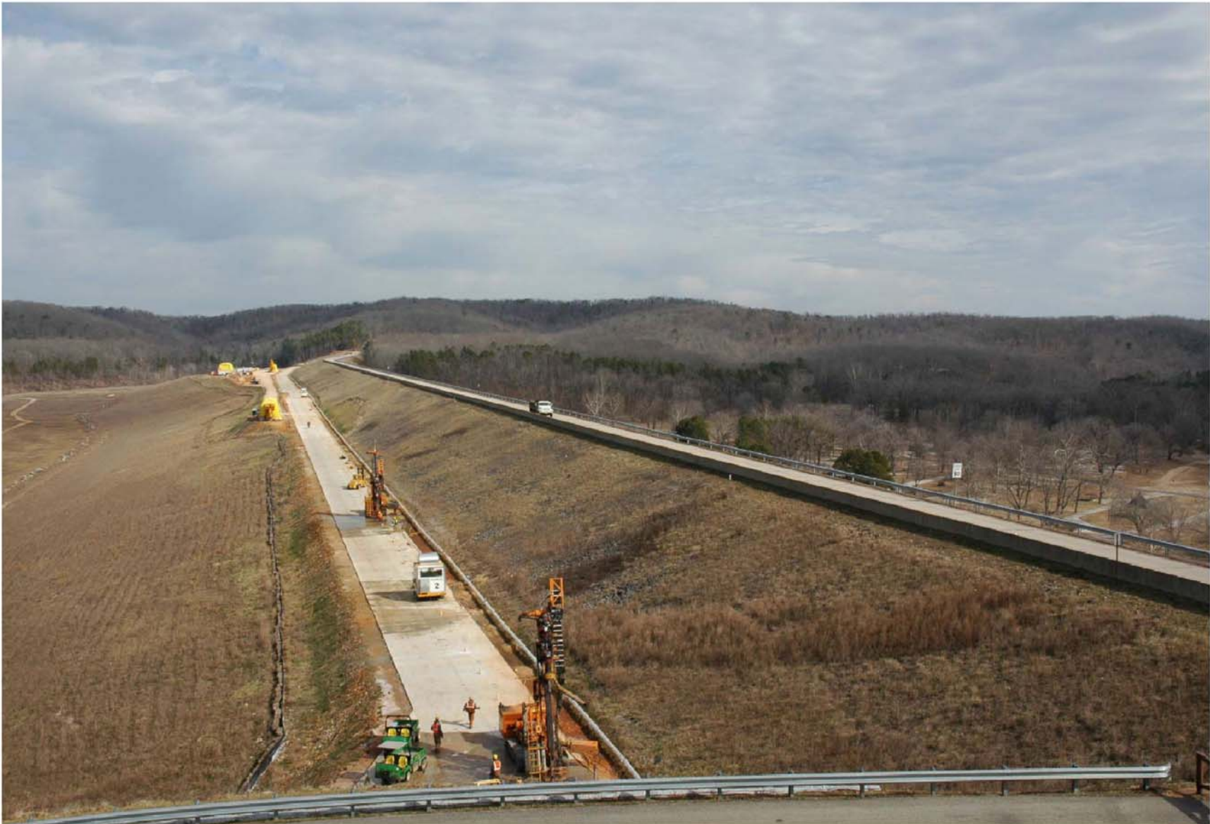
Figure 8. Parapet Wall and Berm
