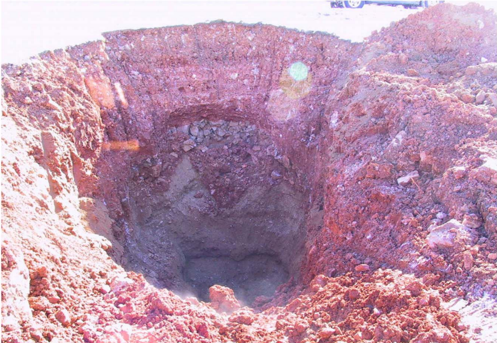
Figure 11. Sinkhole After Excavation
