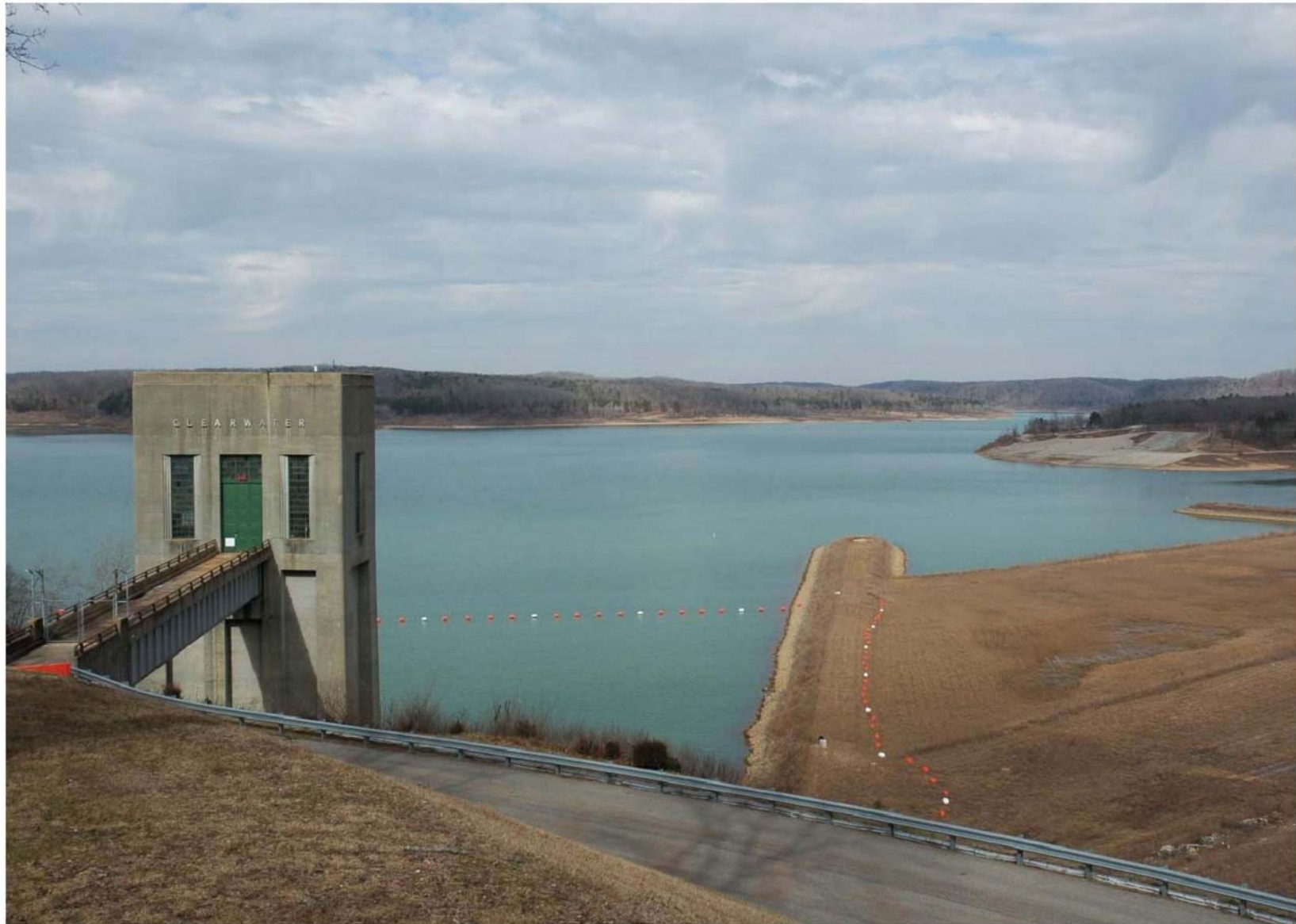
Figure 9. Low Level Outlet Control Tower
