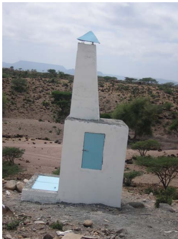
The project initiated this kind of incinerator s in the rural health post which did not exist before
