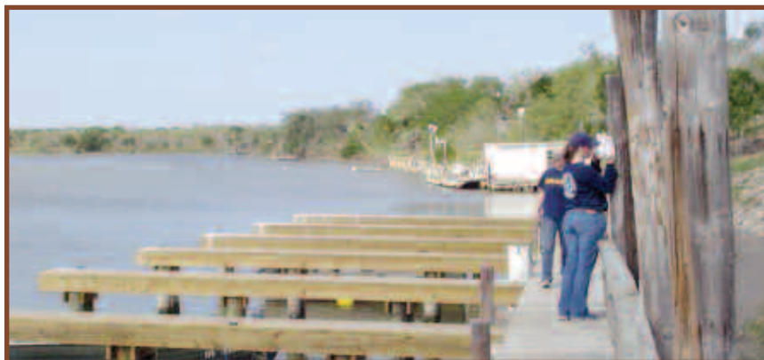
Land Office personnel inspecting a structure on state-owned submerged land.
