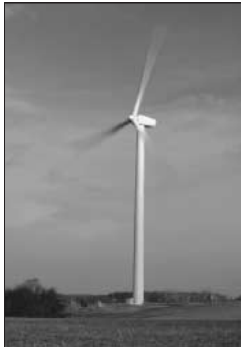
FIGURE 6.1 SOMERSET WIND TOWER
