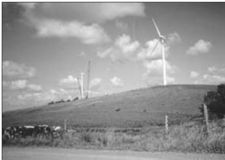
Figure 2.1 View of Fenner wind farm.
