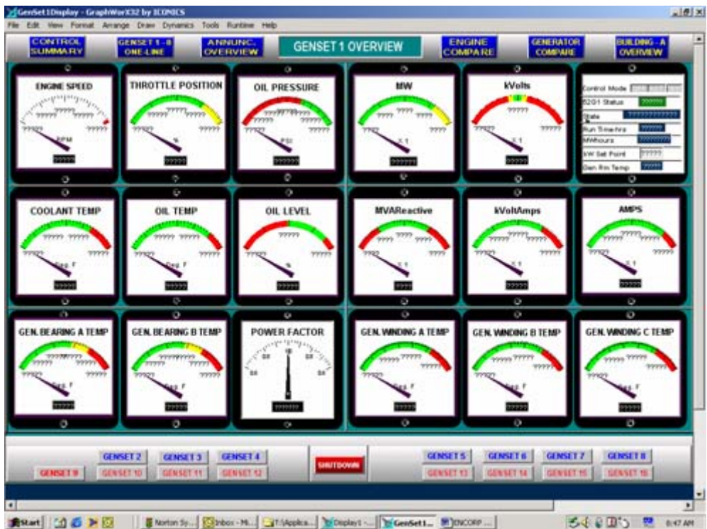
Figure 29: Generator Metering Screen
