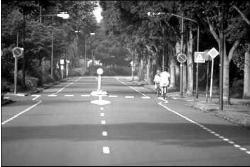
Roadway narrowing increases safety of the drivers and the pedestrians and provides an opportunity to redistribute space to pedestrians
