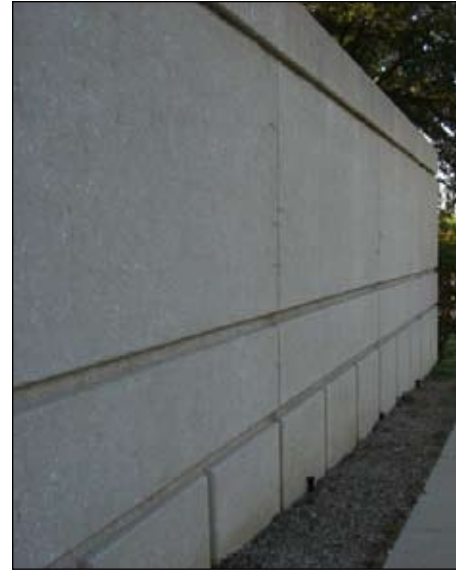
Retaining walls frame existing landscaping
