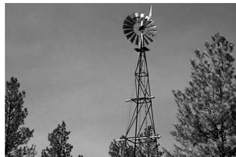
Power generation equipment
