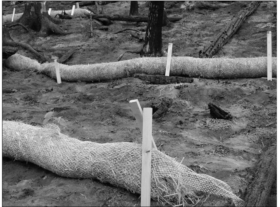
Figure 4: Straw Wattles Used to Help Retain Soils and Reduce Erosion
