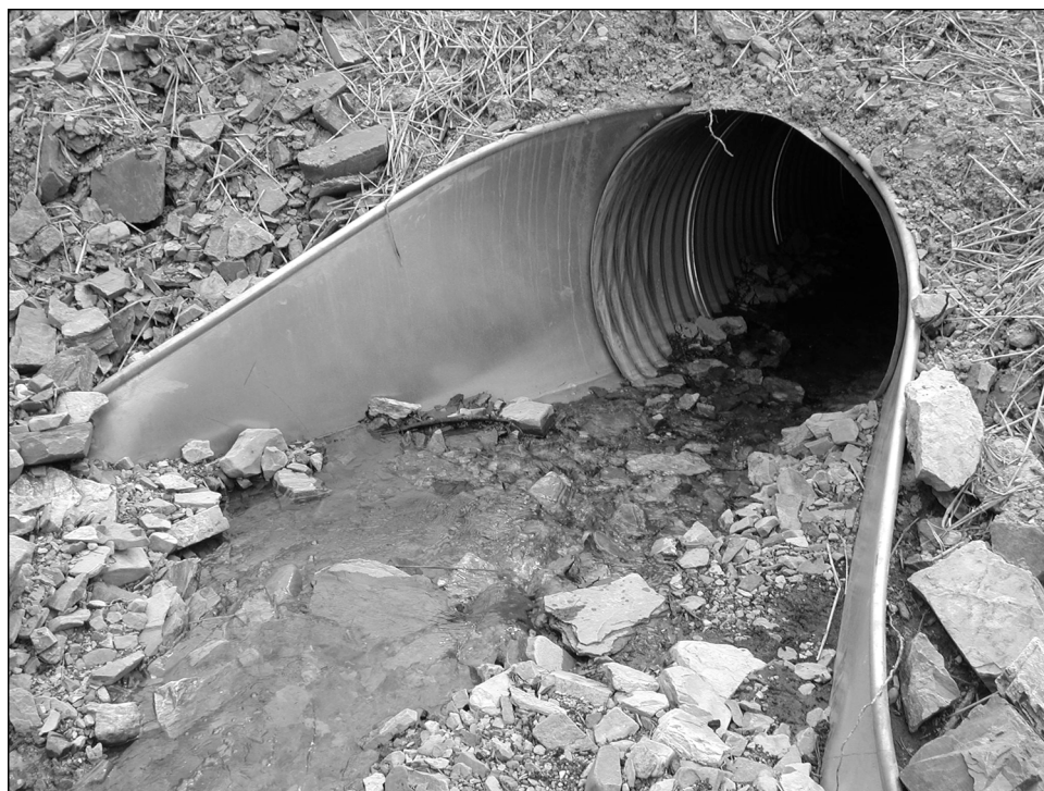
Figure 6: Upgraded Culvert to Withstand Increased Storm Runoff
