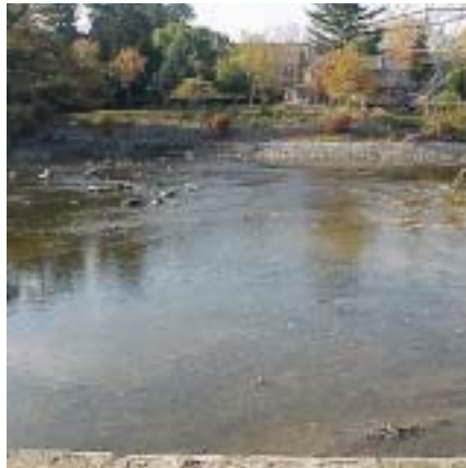
Good Hope dam after removal
