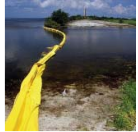
Turbidity barrier crossing the south breach of the impoundment
