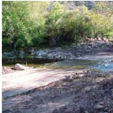
Completed road crossing restoration project
