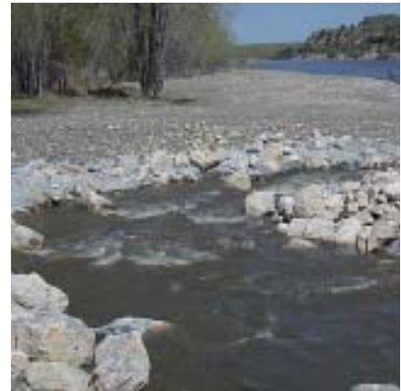
Fish passage channel, looking downstream
