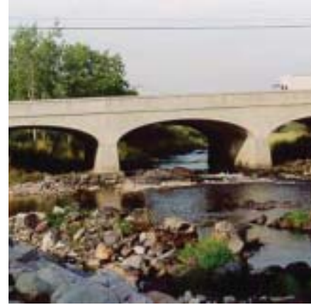
East Machias dam after removal
