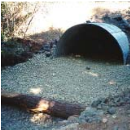
Culvert on Buffin Creek after renovation.
