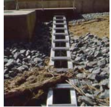
Fish ladder installed at Pleasant Pond dam
