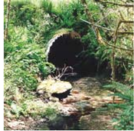
Culvert on unnamed stream before renovation
