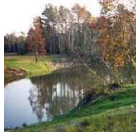
Stream site after dam removal
