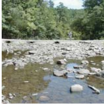
Honobia Creek at Bridge Three before renovation
