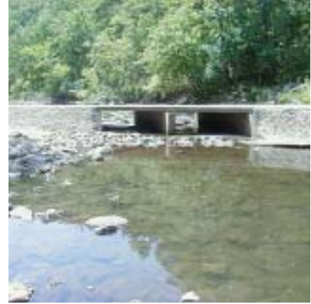
Honobia Creek at Bridge Three after renovation
