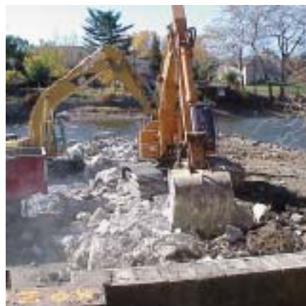
Dam removal on Conodoguinet Creek, PA.
