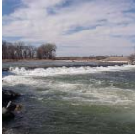
Huntley irrigation diversion dam on the Yellowstone River
