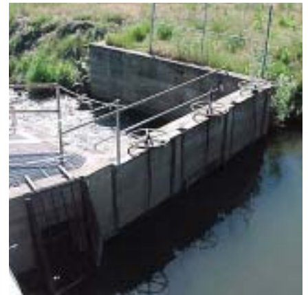
Upstream view of the headgate at East Canal/Blitzen River
