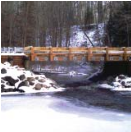
Bridge reconstruction on the North Branch Manistee River at Sharon Road.
