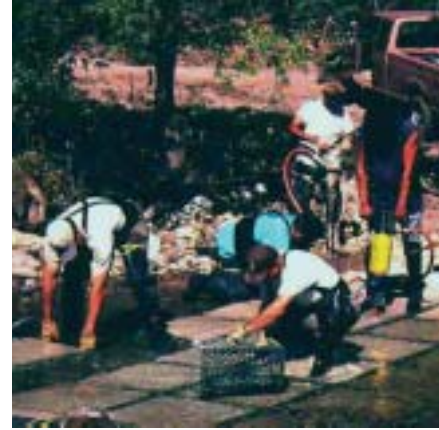
Hand-placing precast slabs
