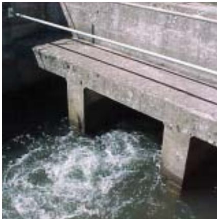
Downstream view of the headgate at East Canal/Blitzen River
