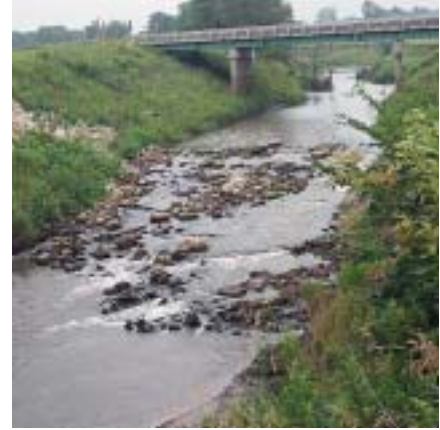
Renovated streambed providing fish passage
