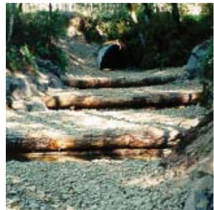
Step pools installed after renovation
