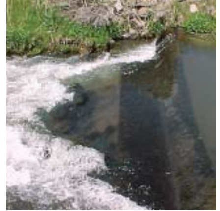
Bridge Creek gaging station creates passage barrier during low flows
