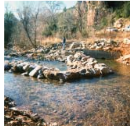
The new design of the Geronimo's Cave irrigation diversion
