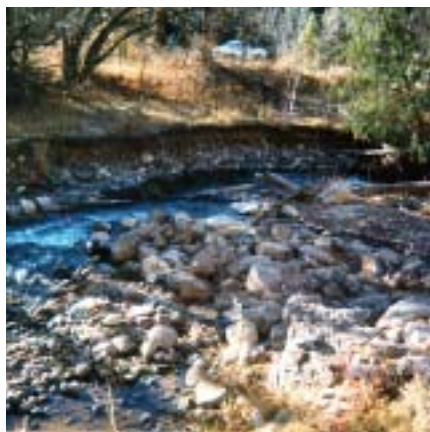
Eroding banks at Geronimo's Cave irrigation diversion
