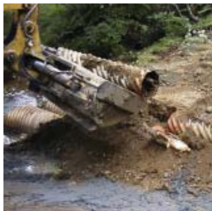
Culvert renovation on Duck Creek, AK.
