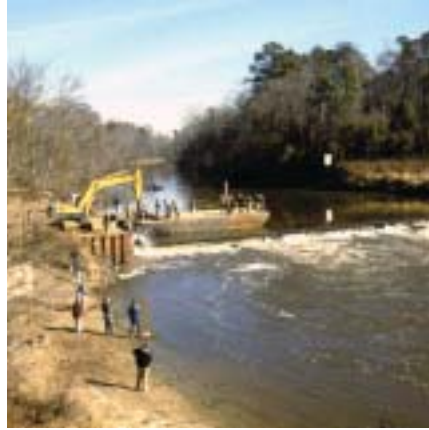
Stream site during dam removal
