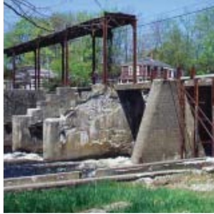
East Machias dam before removal (see road bridge behind dam)
