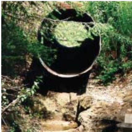
Culvert on Buffin Creek before renovation.
