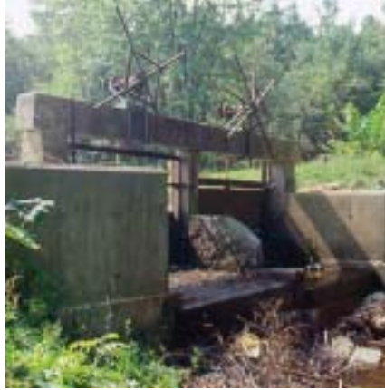
Pleasant Pond dam before fish passage was provided
