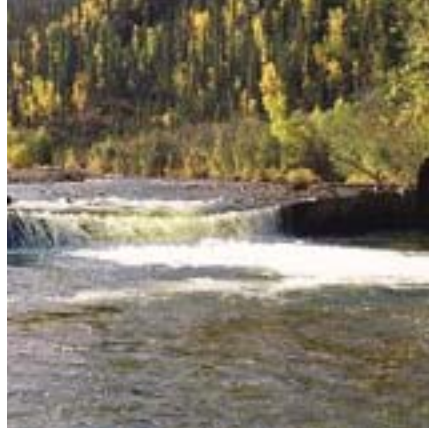
Chatanika dam before removal
