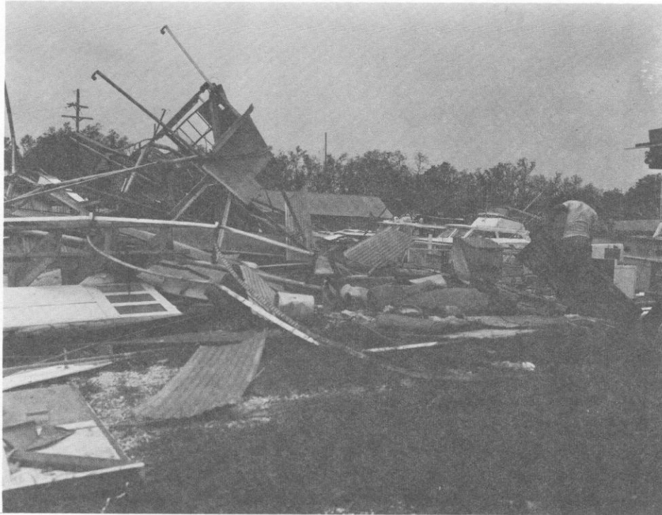
WIND DAMAGE, ORLEANS MARINA NEW ORLEANS, LA., 11 SEPTEMBER 1965
