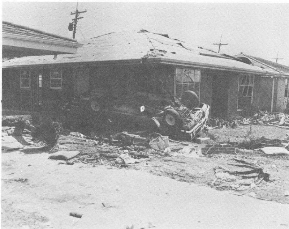
WATER AND WIND DAMAGE NEW ORLEANS, LA.
