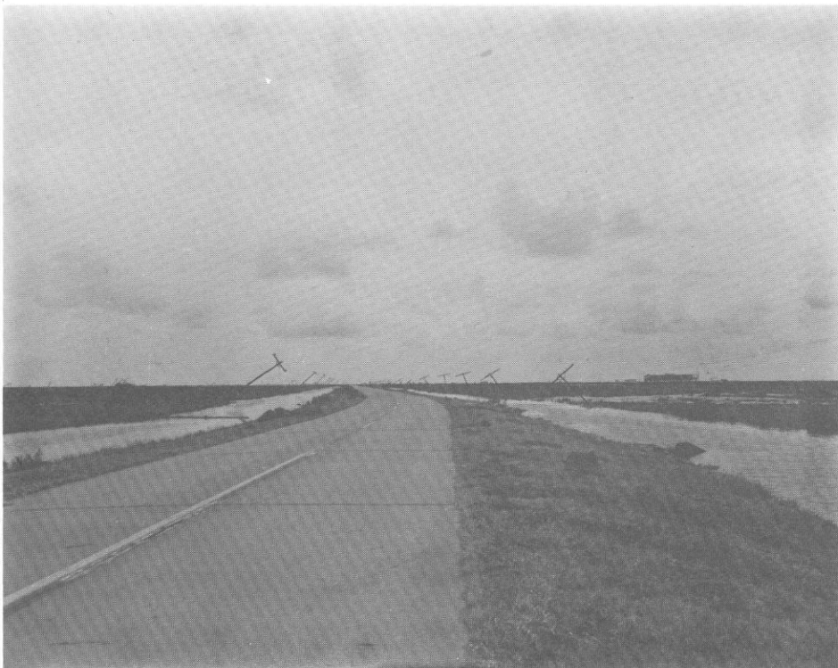
POWER AND TELEPHONE LINE DAMAGES BELOW LEEVILLE, LA.
