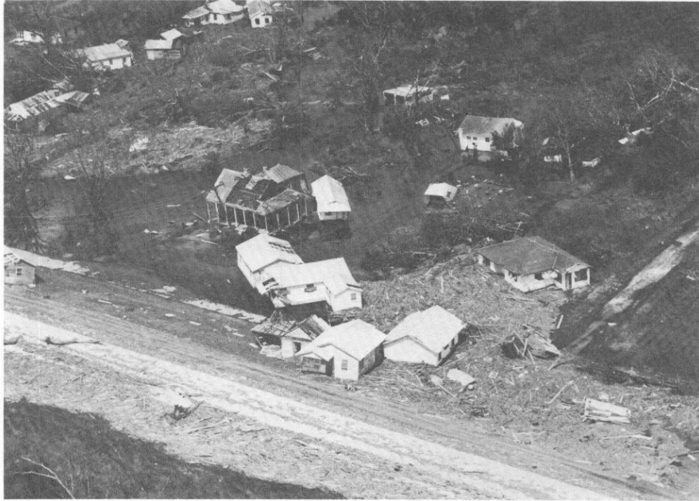
HIGH TIDE, WIND, AND RIVER, POINTE A LA HACHE, LA. 13 SEPTEMBER 1965
