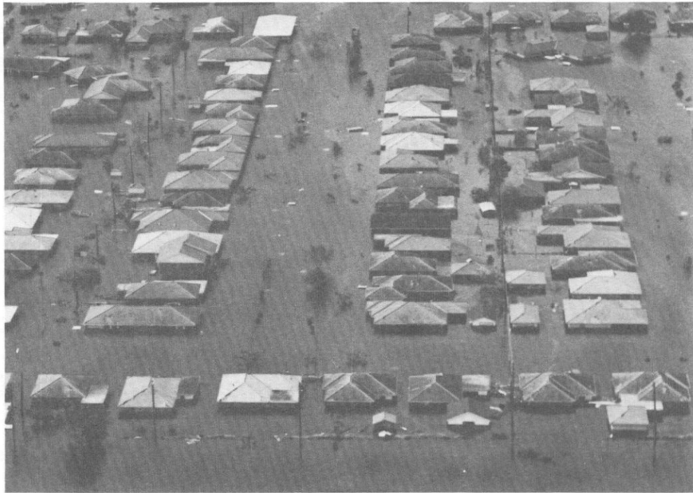
ARABI AREA FLOODED, ST. BERNARD PARISH, LA. 11 SEPTEMBER 1965
