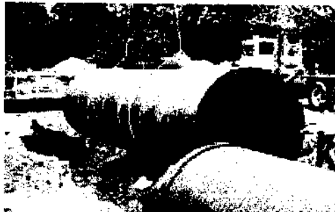
96" Weholite used for water management on a golf course.
