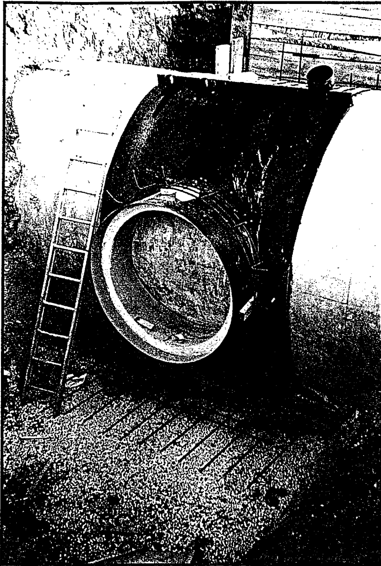
A specially manufactured 54-inch (1350 mm) diameter tapping saddle assembly was installed on the existing cast-in-place concrete aqueduct to provide for the interconnection with the new reservoir cells.
