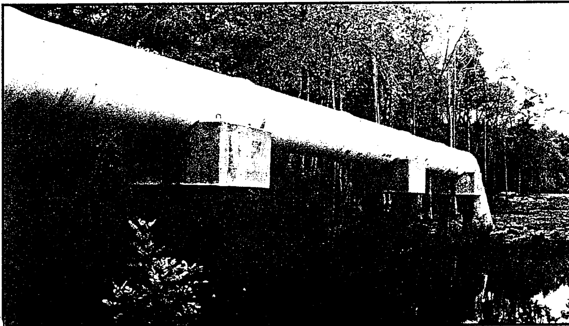
48-inch diameter Concrete Pressure Pipe supported by pile bents with concrete pipe cap.
