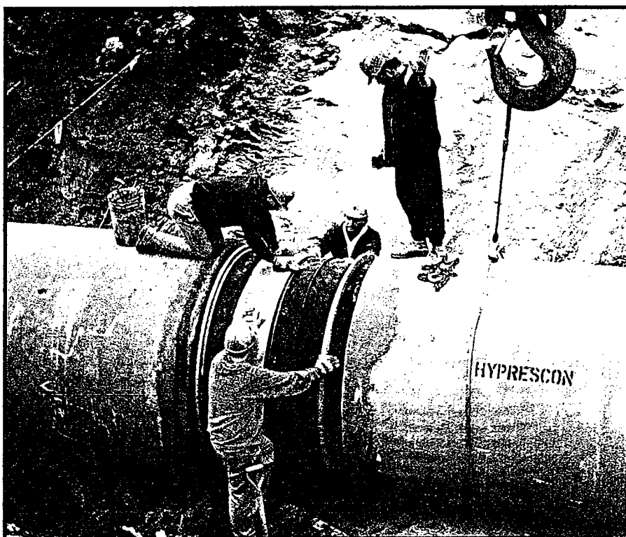
Winnipeg's construction contractor, Nelson River Construction, Inc., prepares to install a 54-inch (1350 mm) diameter closure section for the inlet pipe.
