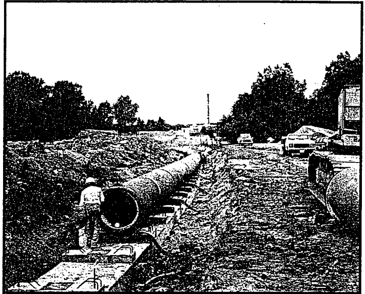
36-inch Concrete Pressure Pipe installation on a grade support beam built atop a pile foundation crossing a land-fill site
