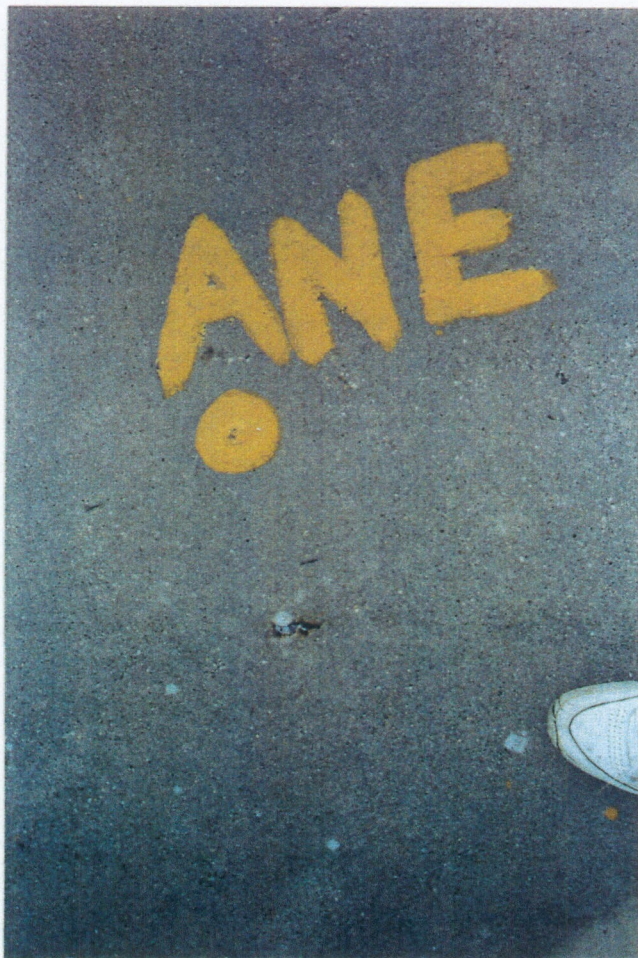
PHOTO 8: EXPOSED PIECE OF METAL ON TOP SURFACE OF EAST GATE MONOLITH. NO CHANGE OR DETRIMENTAL ACTION TO THE CONCRETE SINCE INSPECTION NO. 4.
