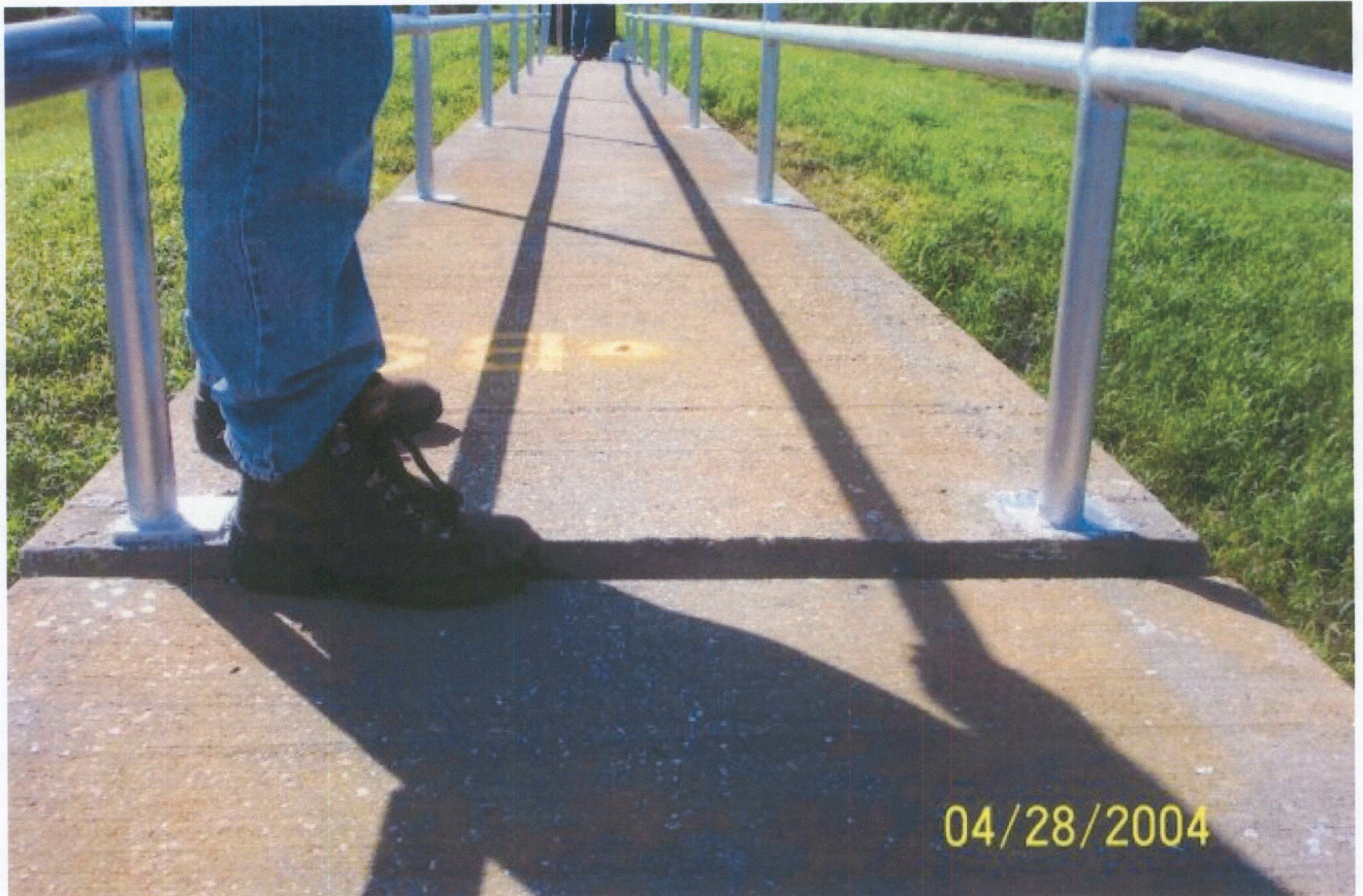
Photo No. 35 – Settlement reference markers (SRM) noted atop the “T” Floodwall.
