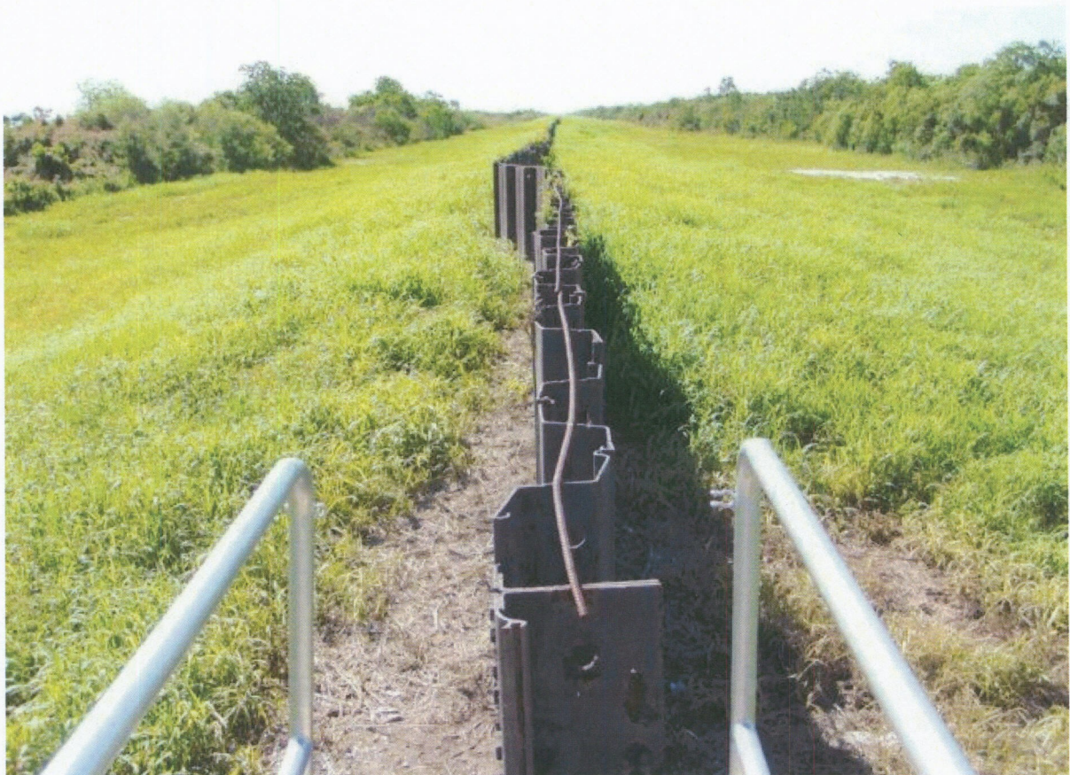
Photo No. 27 – East side steel sheetpile “I” floodwall.
