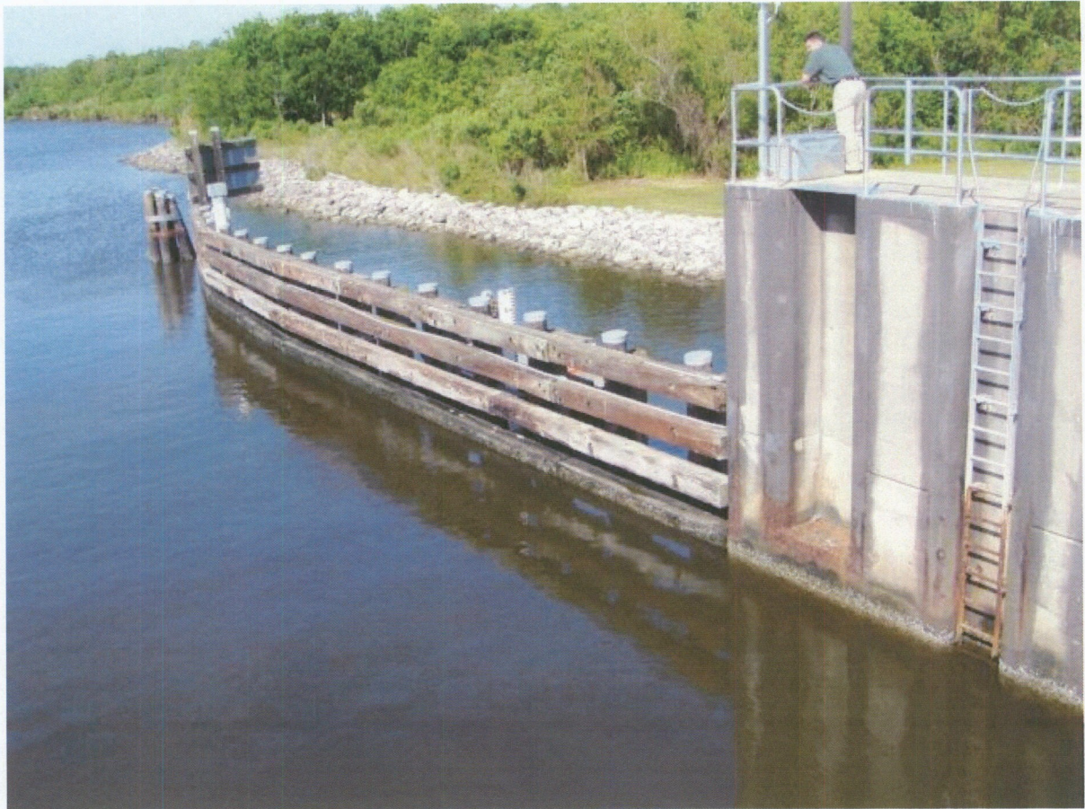
Photo No. 29 – Southwest guidewall noted in good condition.
