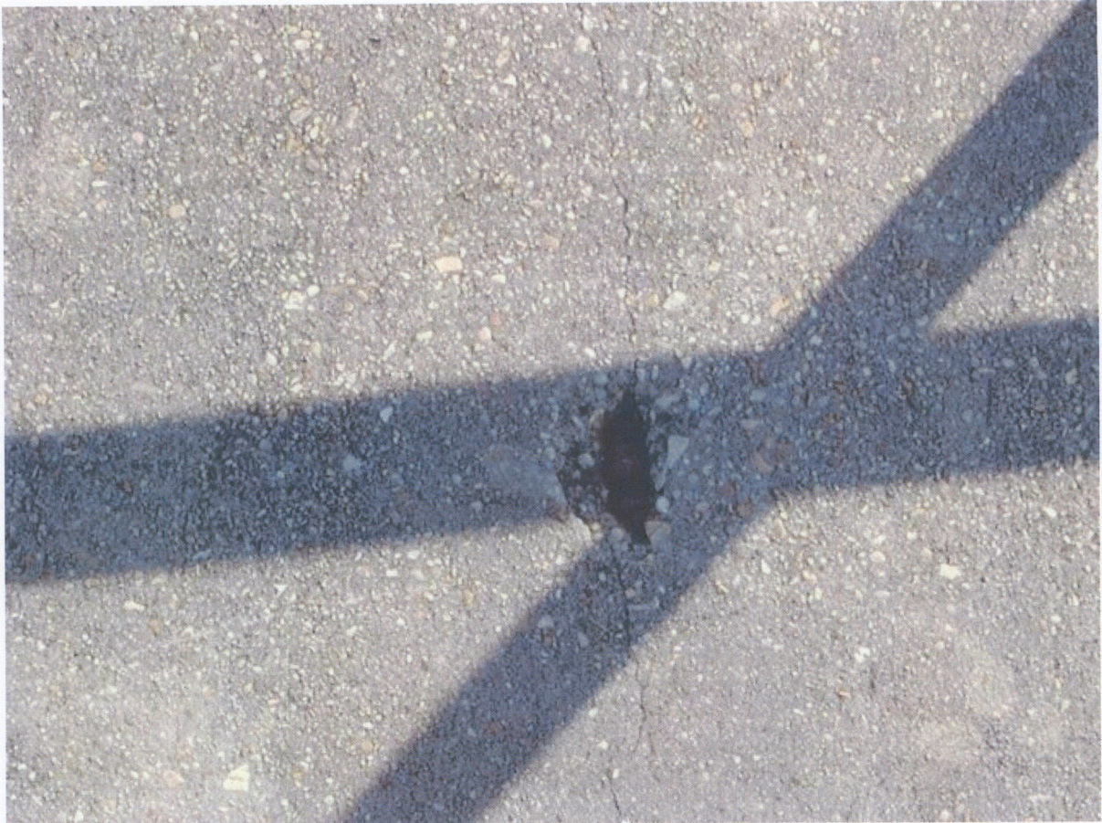
Photo No. 19 - Exposed rebar on the walkway atop the inverted west "T" floodwall.
