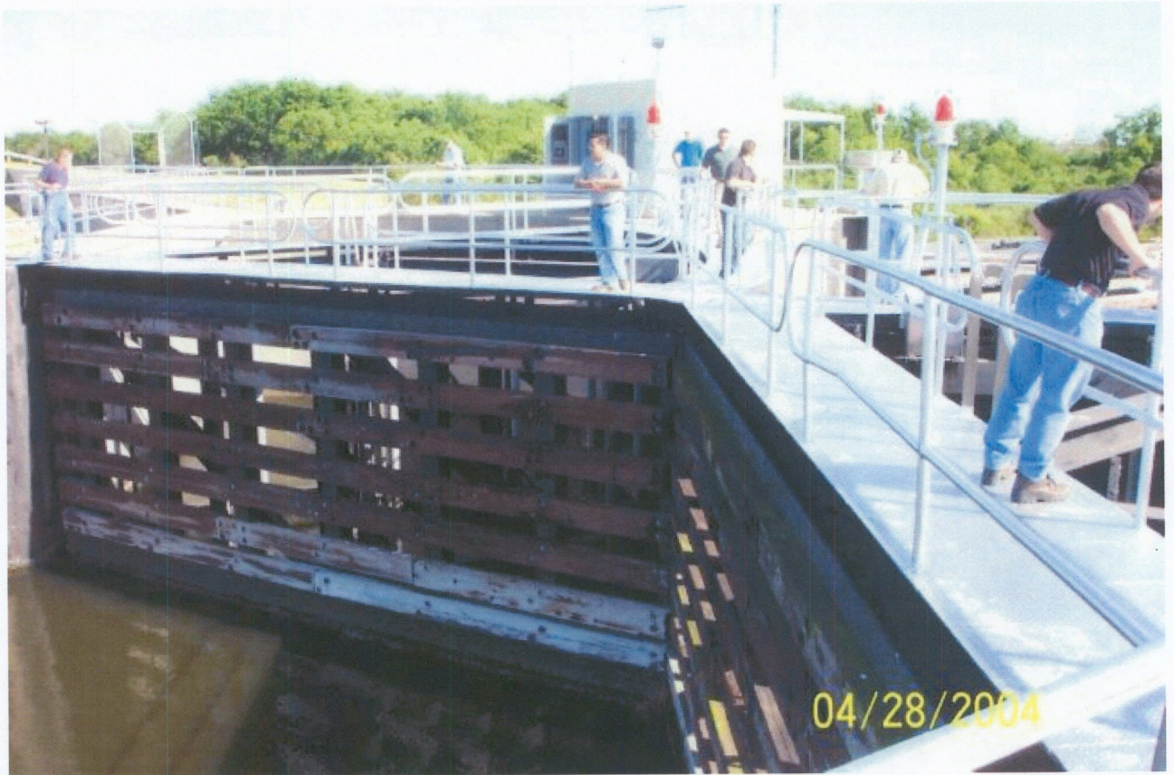
Photo No. 5 – Steel walkways and handrails noted in excellent condition
