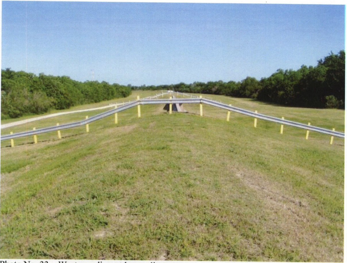
Photo No. 33 – Western adjacent levee alignment.
