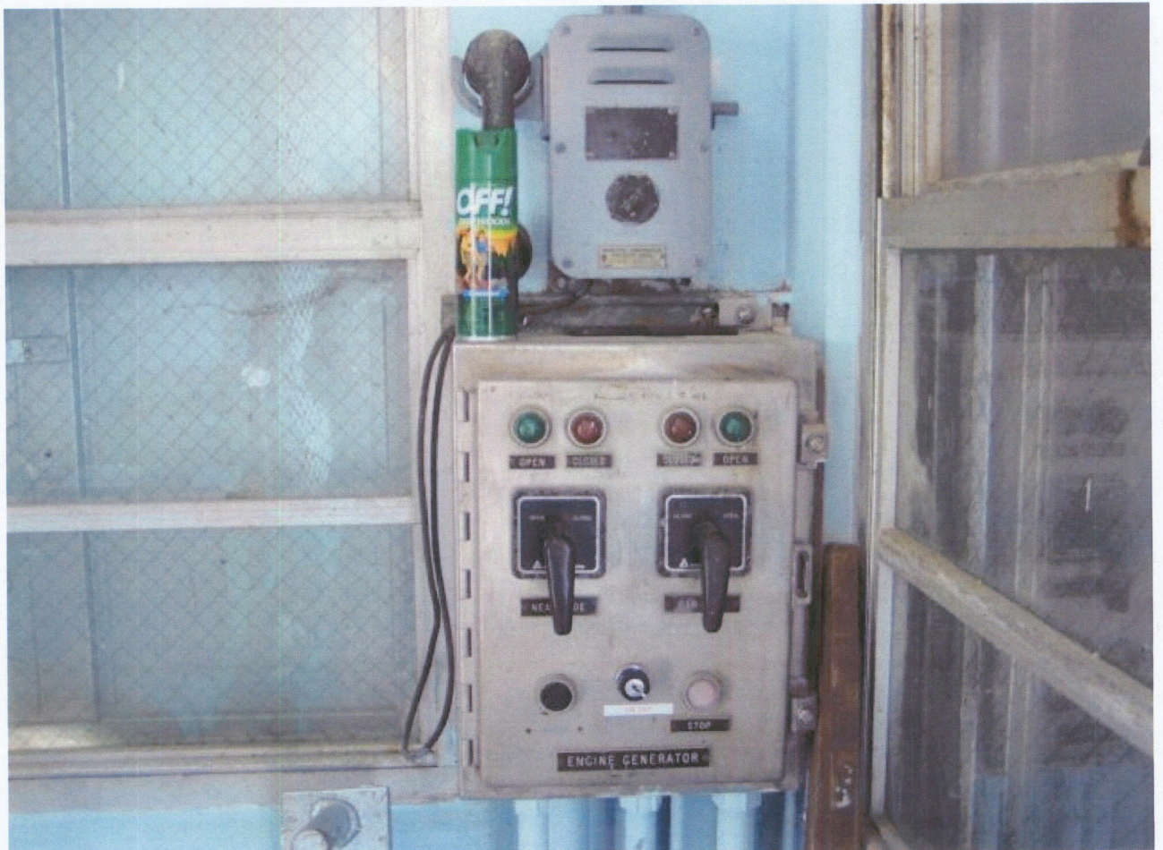
Photo No. 6 – Original controls for the gate operating machinery.
