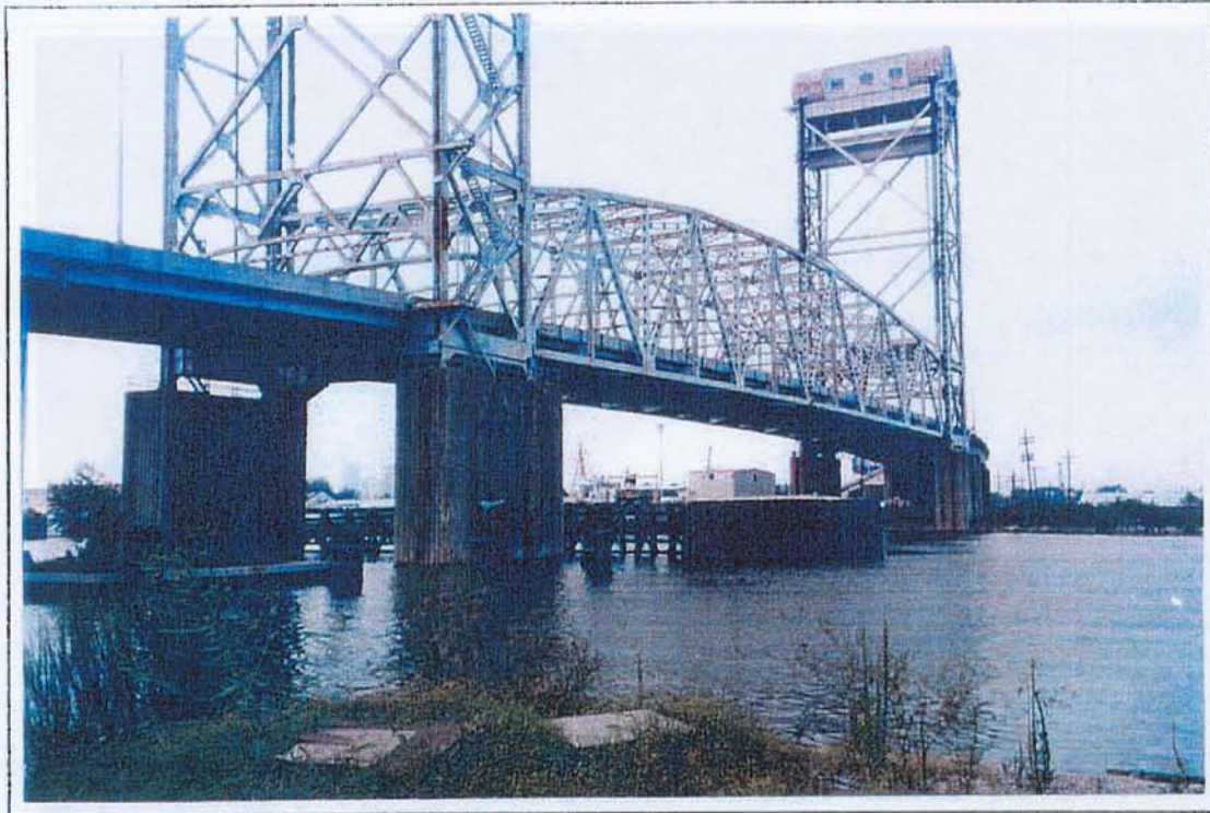
13. A view to the south-southwest of the Clairborne Avenue Bridge and the collection area for the background sediment sample associated with this project. Sampling Location IEBS-22.
