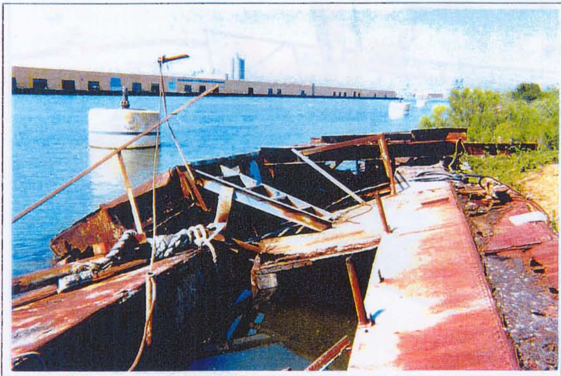
32. A view to the north of Barge 36-039
