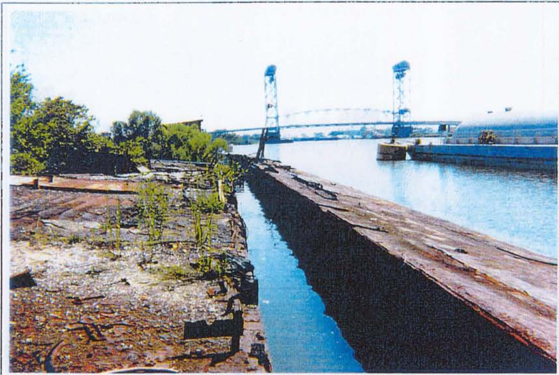
16. A view to the south-southwest of abandoned barges along the waterfront of Saucer Marine. Sampling Location IEBS-05.
