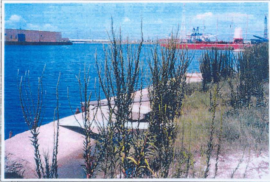
7. A view to the north-northeast along the waterfront of Mayer Yacht-Distributor's Oil. Sampling Location IEBS-10.
