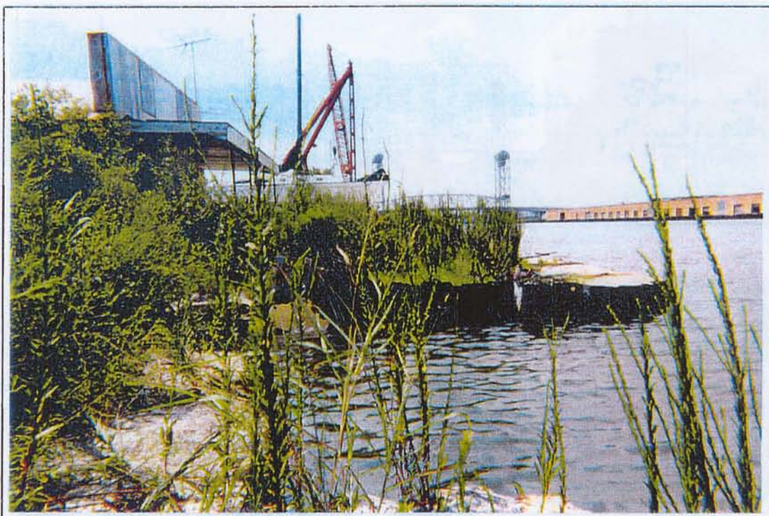
6 A view to the south-southwest along the waterfront of Mayer Yacht-Distributor's Oil. Sampling Location IEBS-11.
