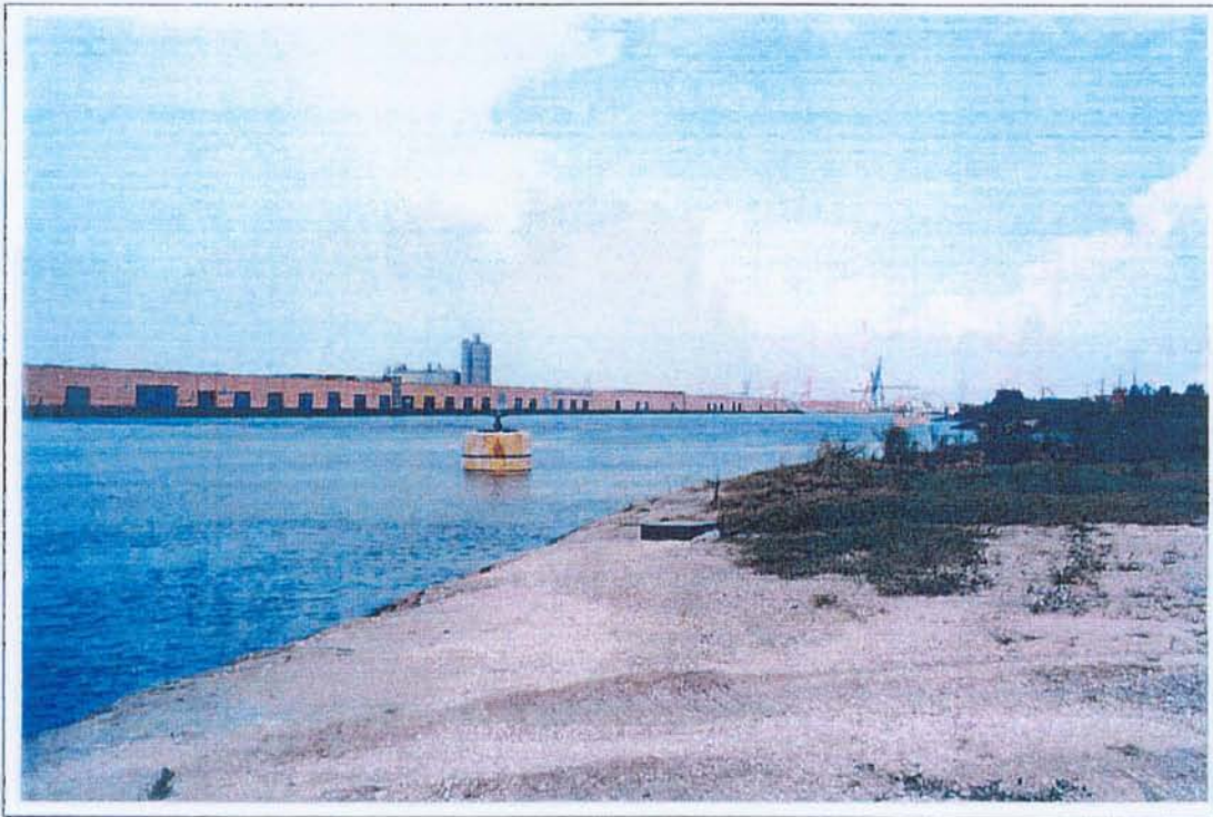
A view to the north-northeast along the waterfront of International Tank Terminal.
