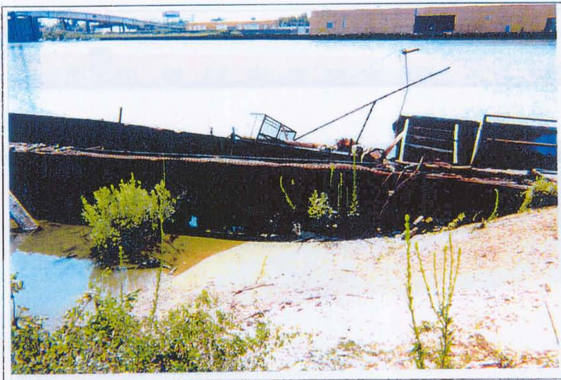
34. A view to the west of Barge 36-039.
