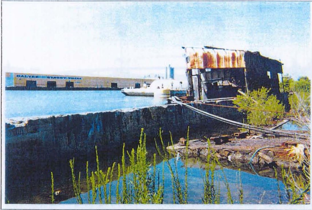
39. A view to the north of Barge 36-042.
