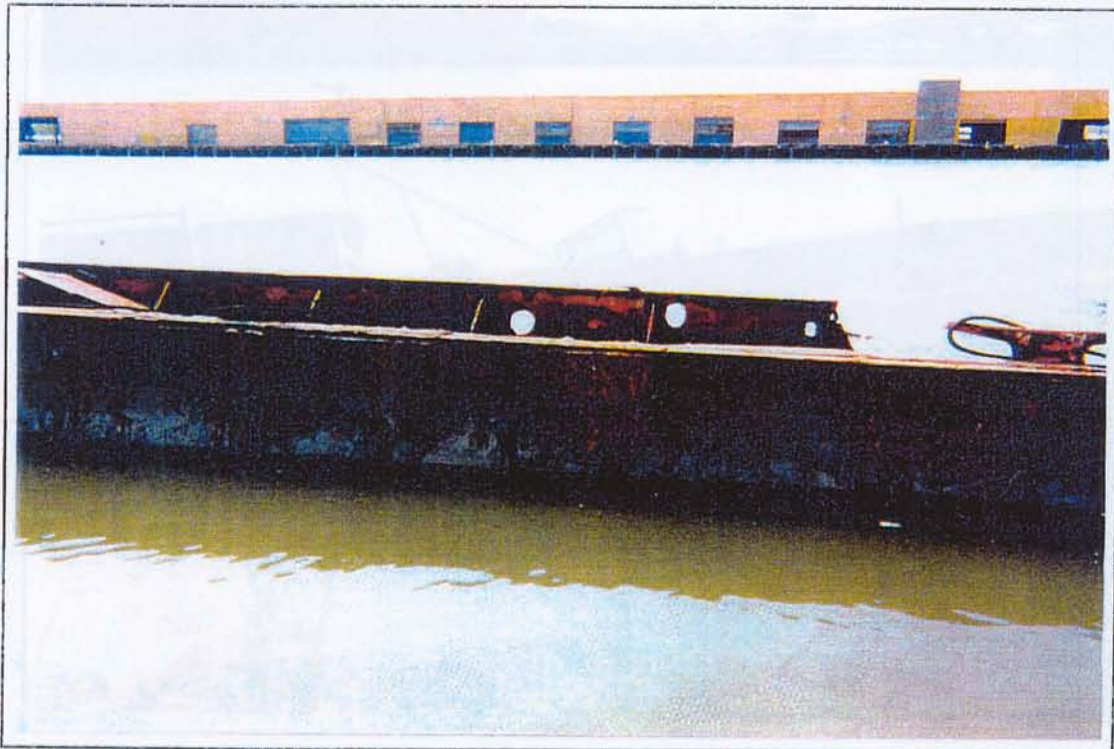
36. A view to the west of Barge 36-040.
