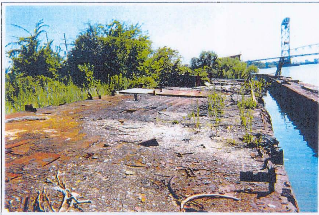
46. A view to the south-southwest of Barge 36-045.
