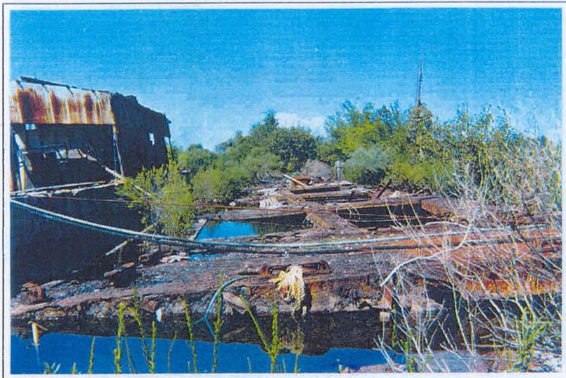
42. A view to the north of Barge 36-043.
