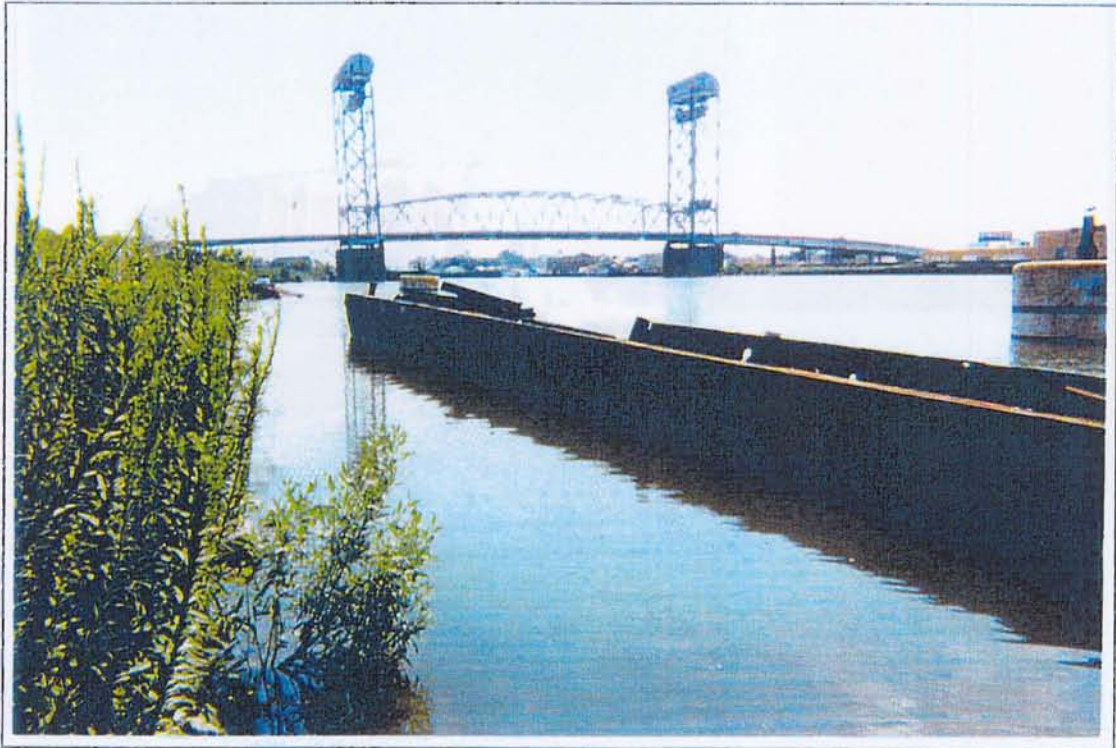
37. A view to the south-southwest of Barge 36-040.
