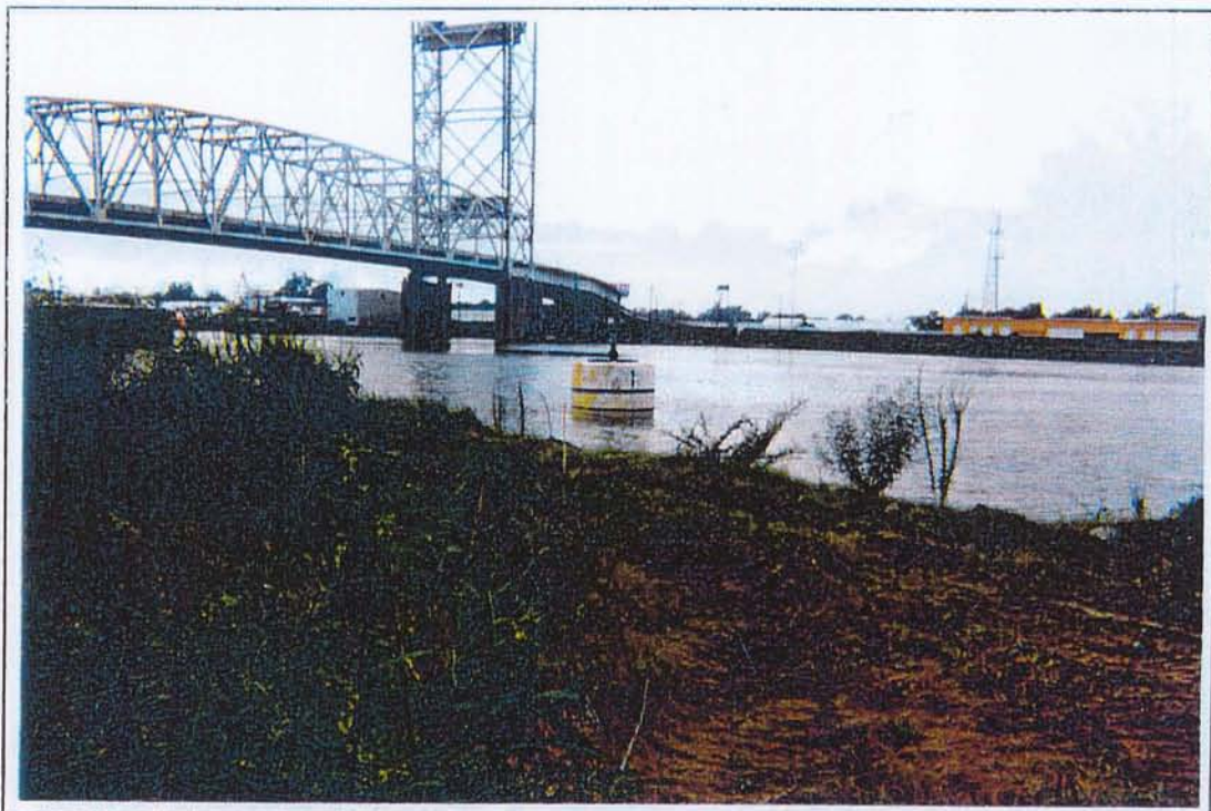
12. A view to the south-southwest along the waterfront of International Tank Terminal. The Claiborne Avenue Bridge is located in the background of the photograph.
