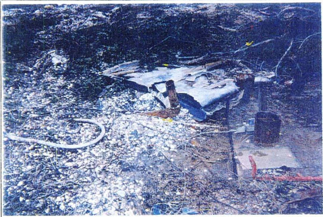
25 View to the north of the west end of the concrete pad (former AST pad). Four inch metal piping on the west end of the pad runs to the west toward the piping observed at Test Pit 120-60-1.
