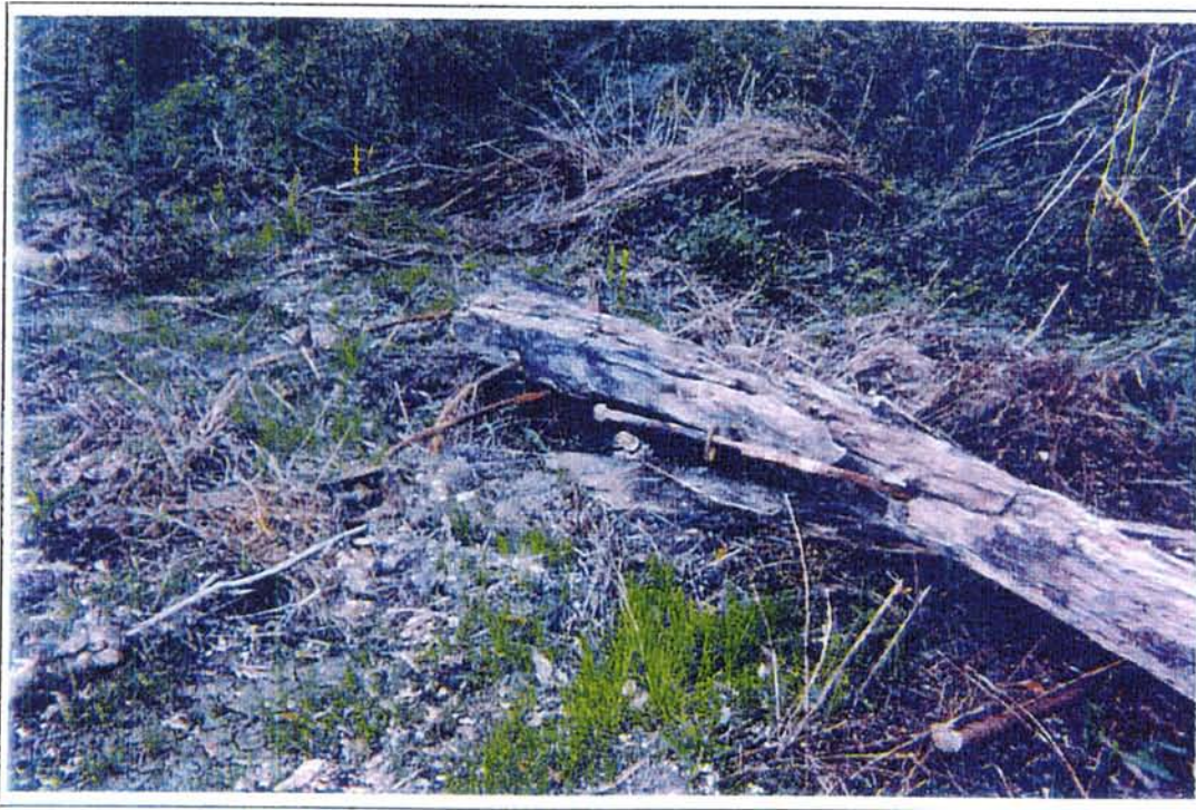
20. View to the northwest of timbers with large metal bolts.
