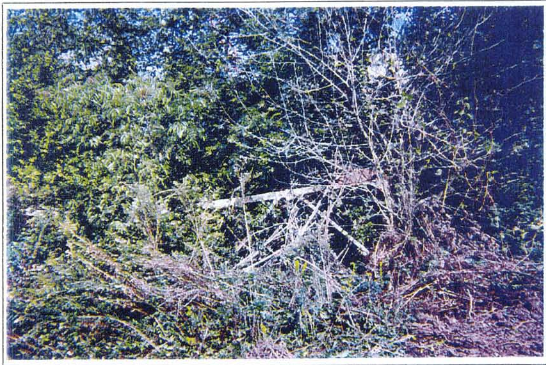
14. View to the north of a metal structure covered with dense vegetation.
