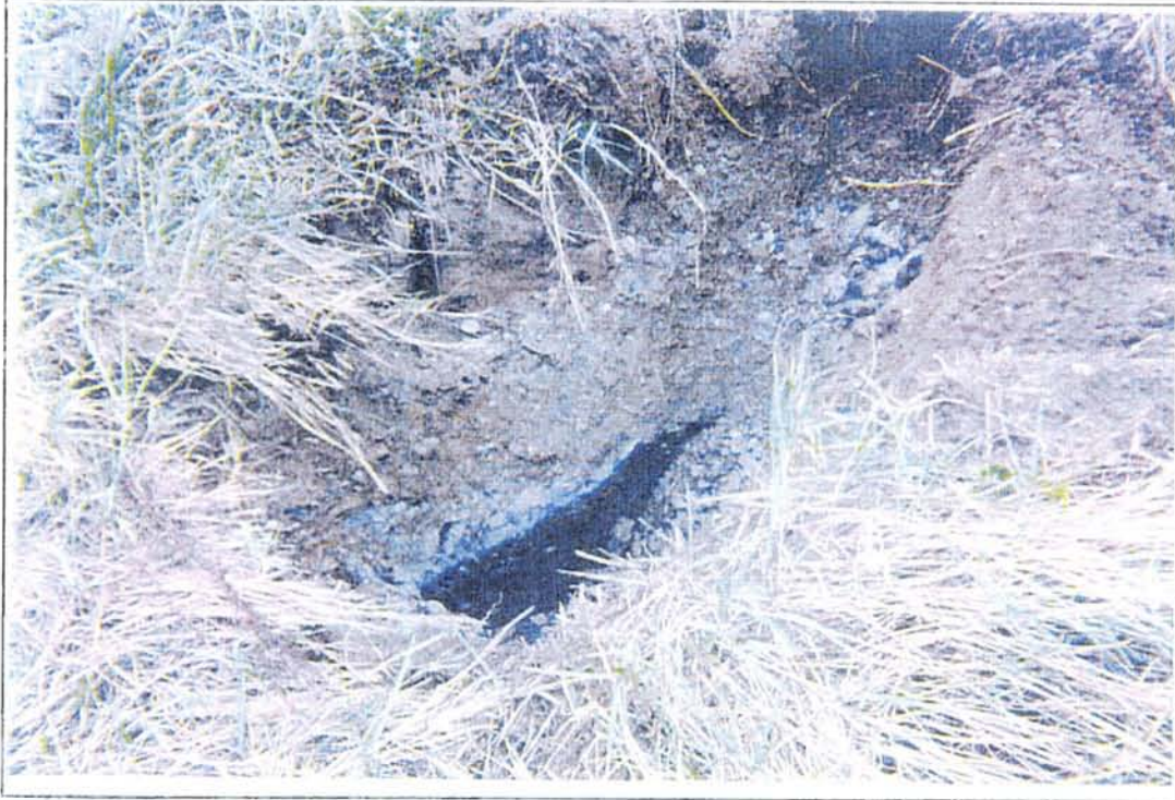
35 View to the northwest of petroleum impacted soil observed along the six-inch piping observed in the vicinity of Test Pit TP-120-60-17
