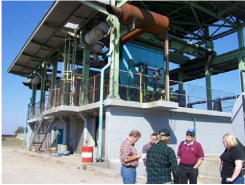
Pump Station No. 1 Building
