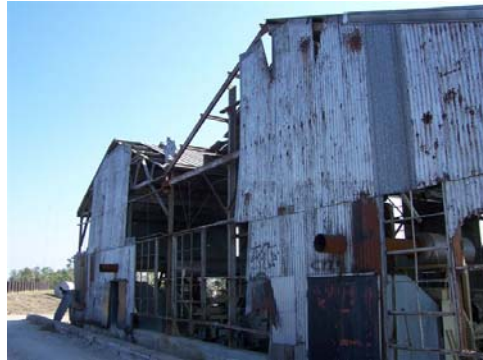
Pump Station No. 2 Building
