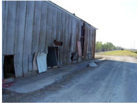
Pump Station No. 3 Building
