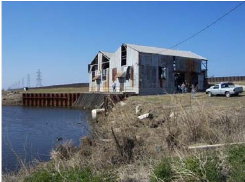
Pump Station No. 2 Building
