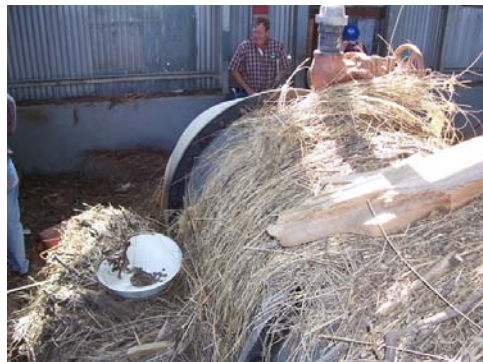
Flood Damaged Engine and Pump
