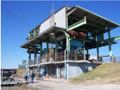
Pump Station No. 4 Building
