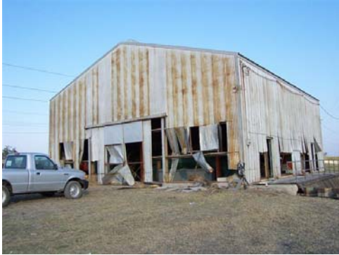
Pump Station No. 3 Building
