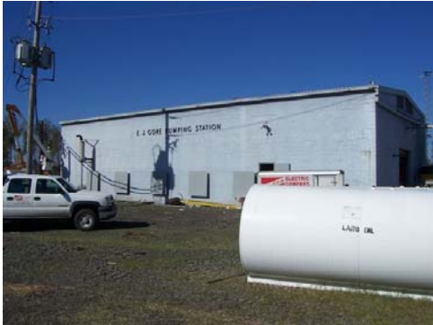
Pump Station No. 5 Building
