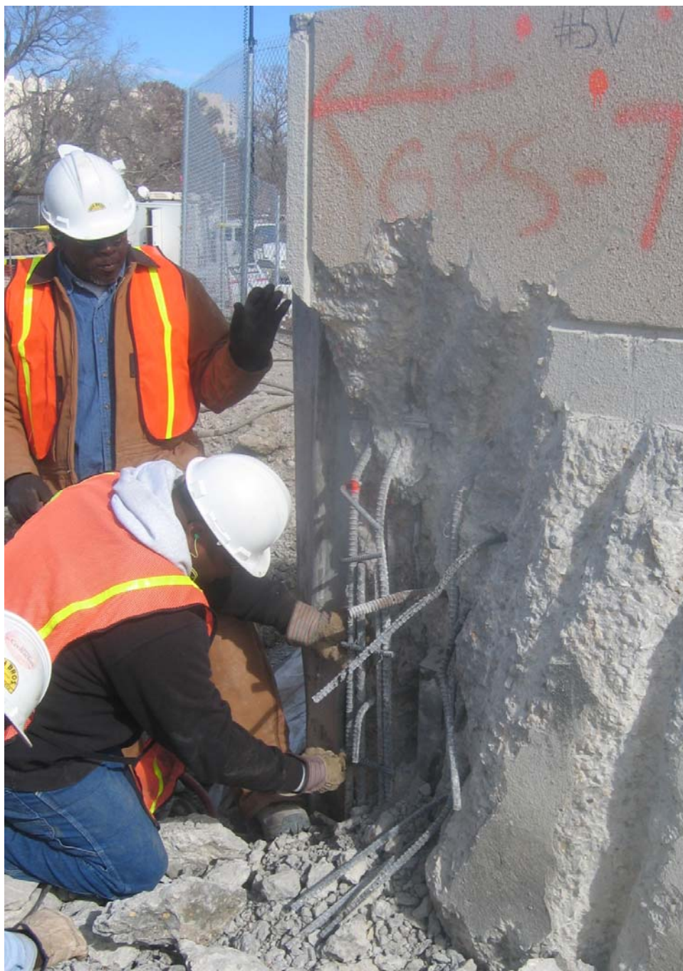
Figure K4-15. Number 6 rebar sample being taken from panel H38
