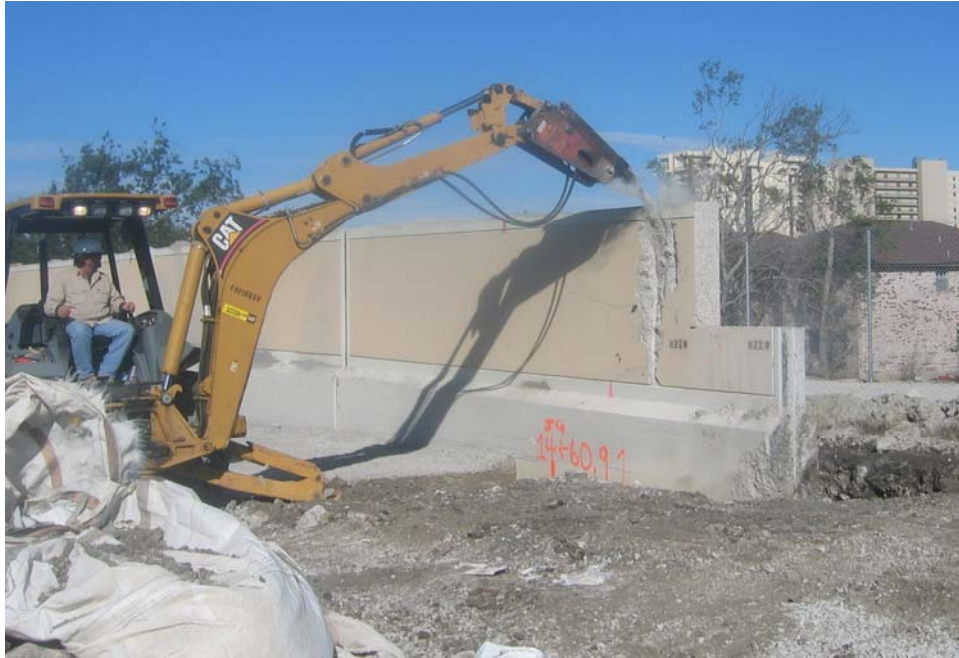
Figure K4-12. Demolition of concrete for rebar sampling at panel H22
