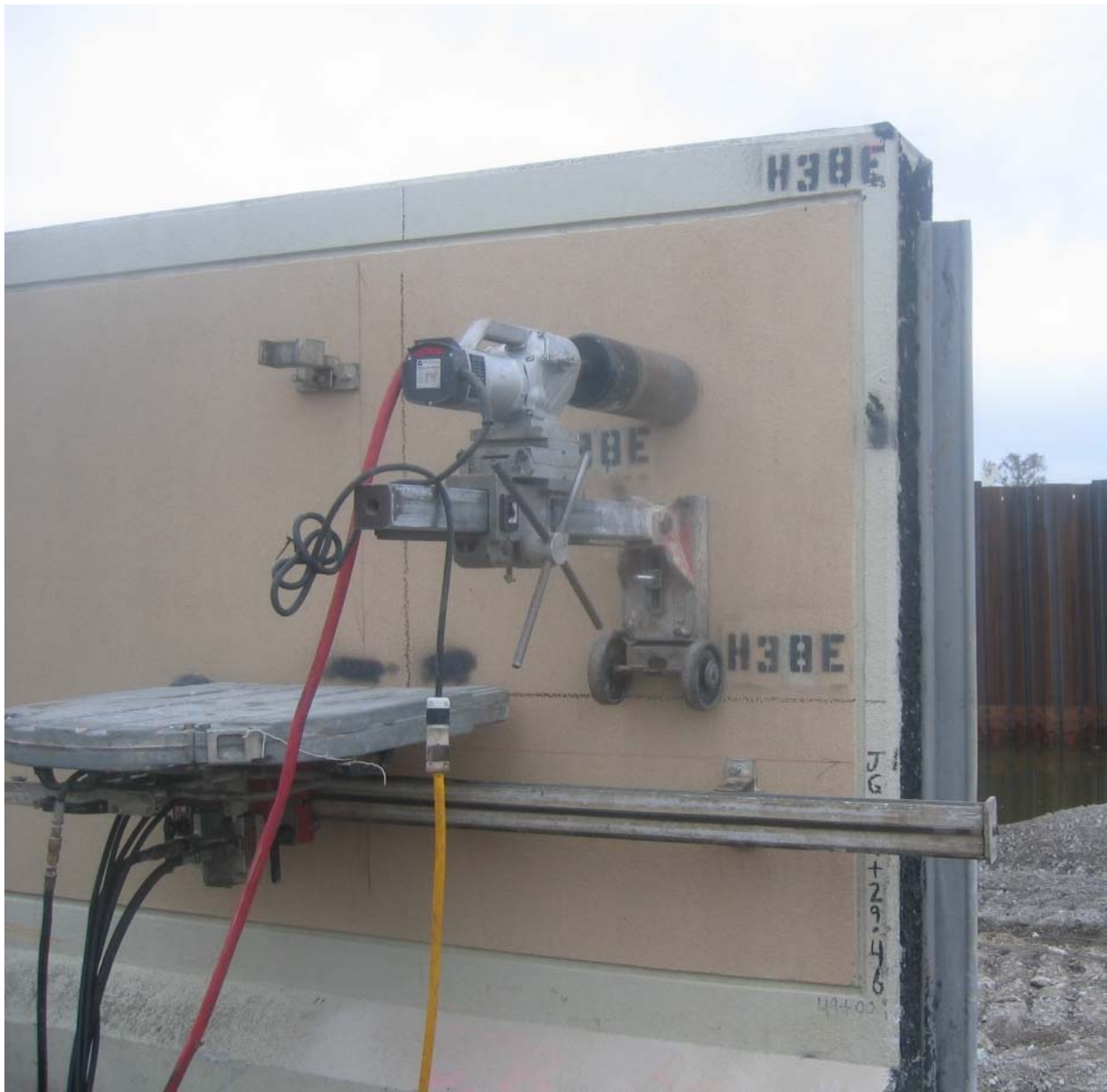
Figure K4-3. Core drill and saw mounted to wall panel H38
