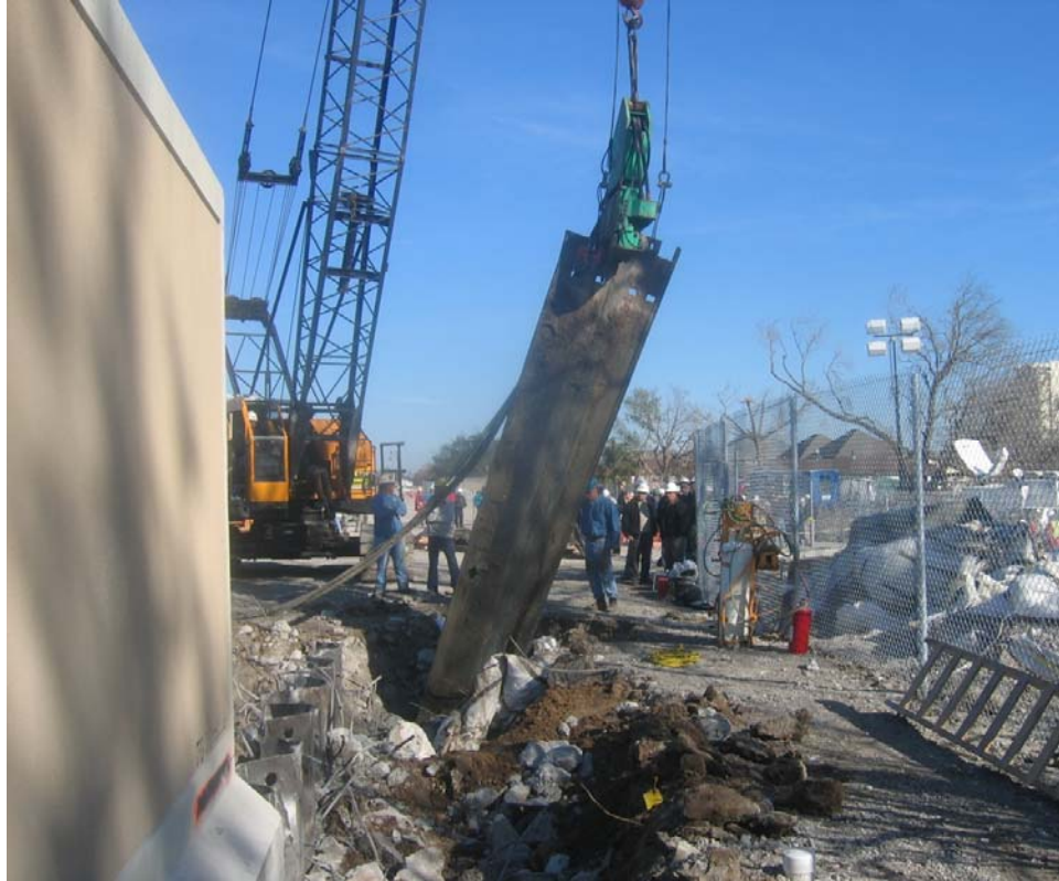
Figure K4-21. Extraction of sheet piles MH37SP1 and MH37SP0
