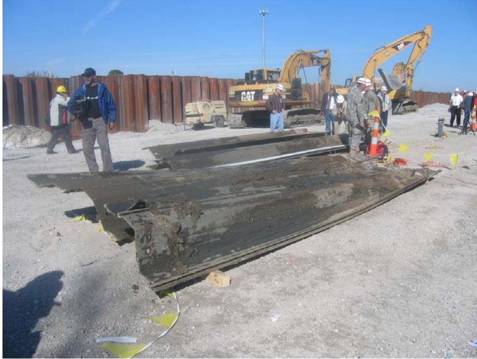
Figure K4-24. Sheet piling extracted from south end of breach
