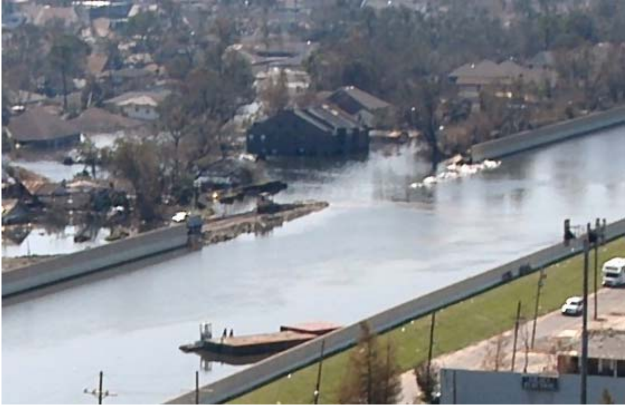
Figure K4-1. 17th Street canal breach
