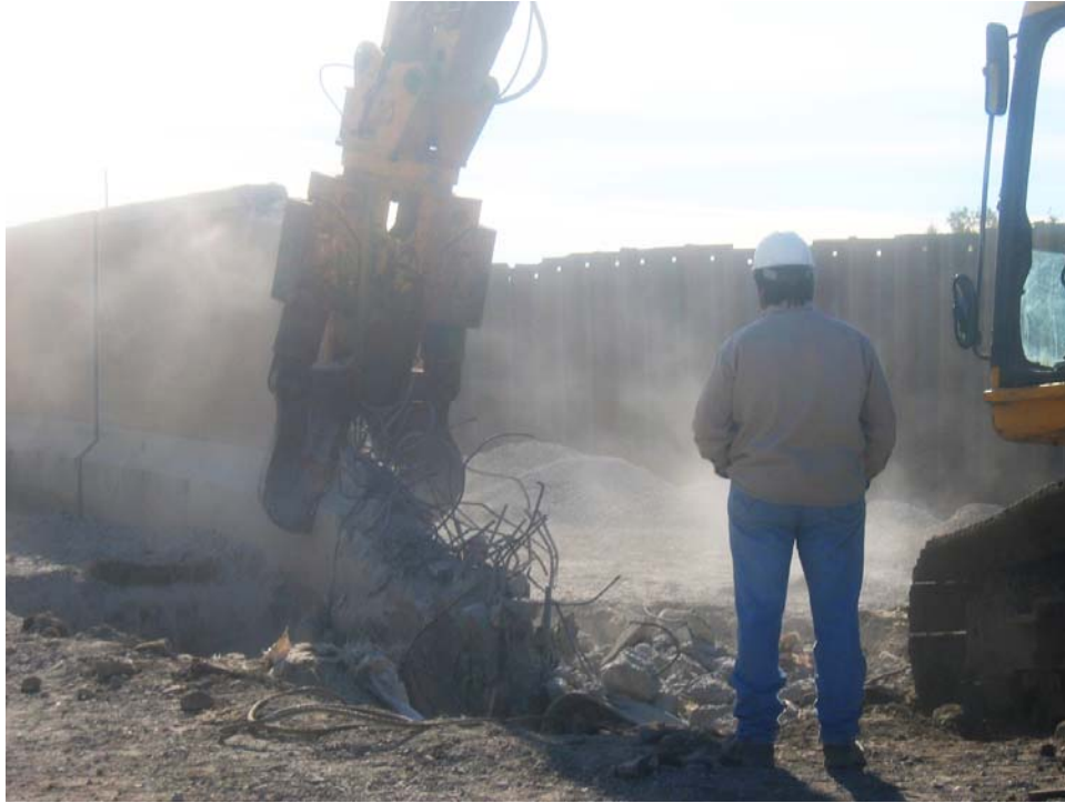
Figure K4-17. Demolition of top portion of wall panel H38
