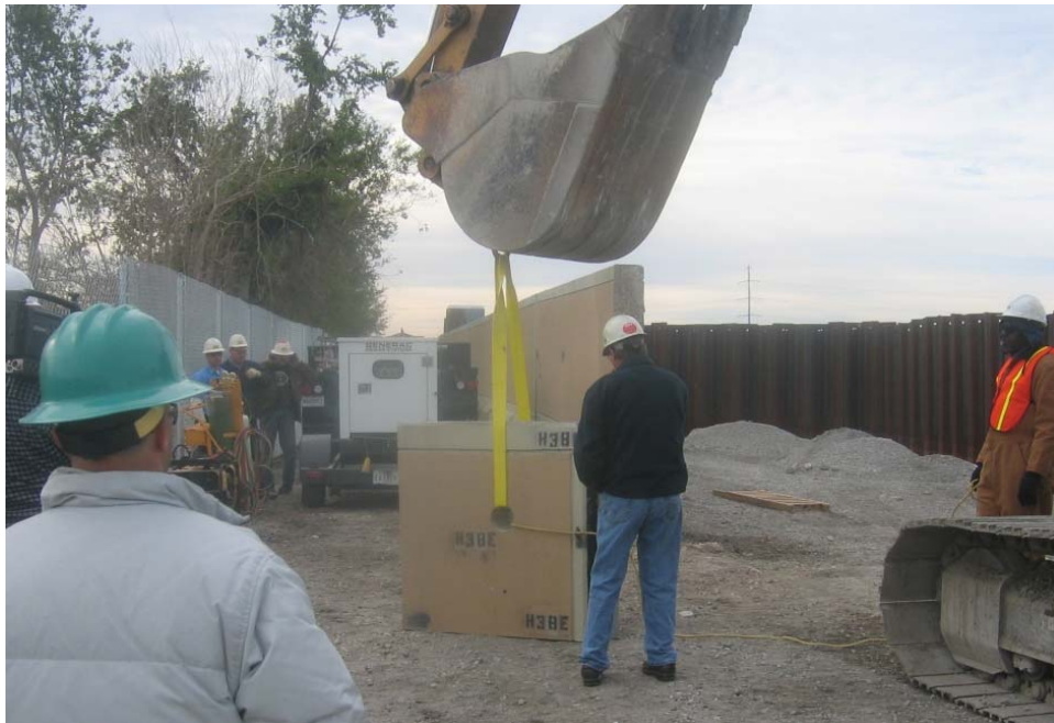
Figure K4-7. Removal of sample from wall panel H38
