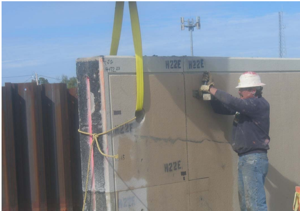
Figure K4-9. Sample being removed from wall panel H22
