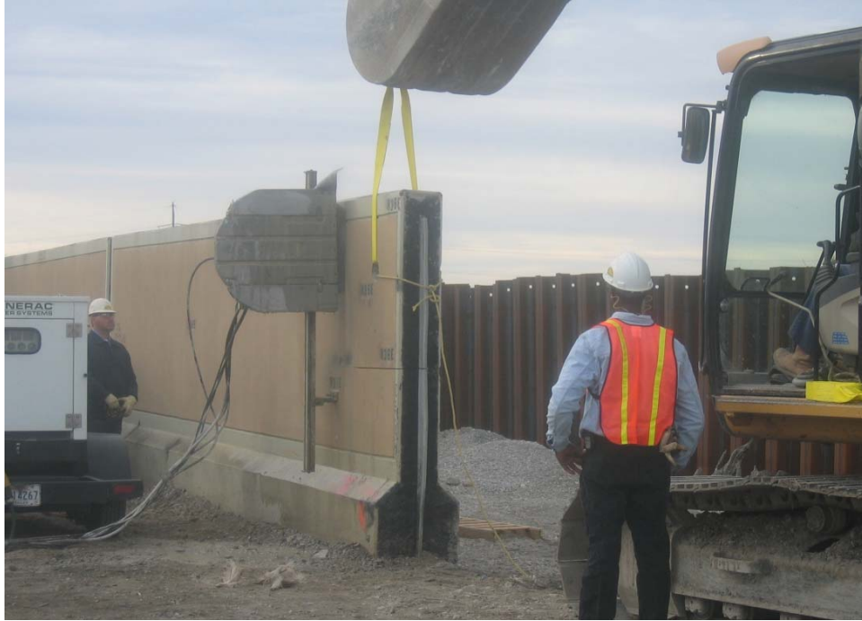
Figure K4-6. Sawing of sample from wall panel H38
