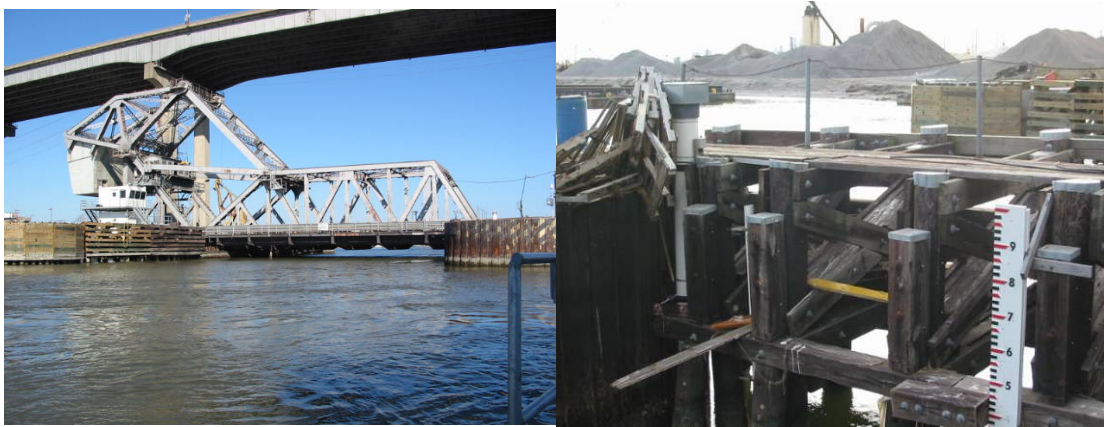
Figure III-26. (Left) IHNC Almonaster Bridge—low chord elevation 3.51 ft NAVD88 (2004.65). (Right) Leveling to USGS recording gage and Orleans Levee District staff gage on I-10 bridge over IHNC
