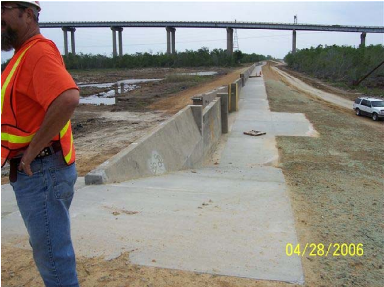
Figure STB 32. TFG repairs to Paris Road floodwall
