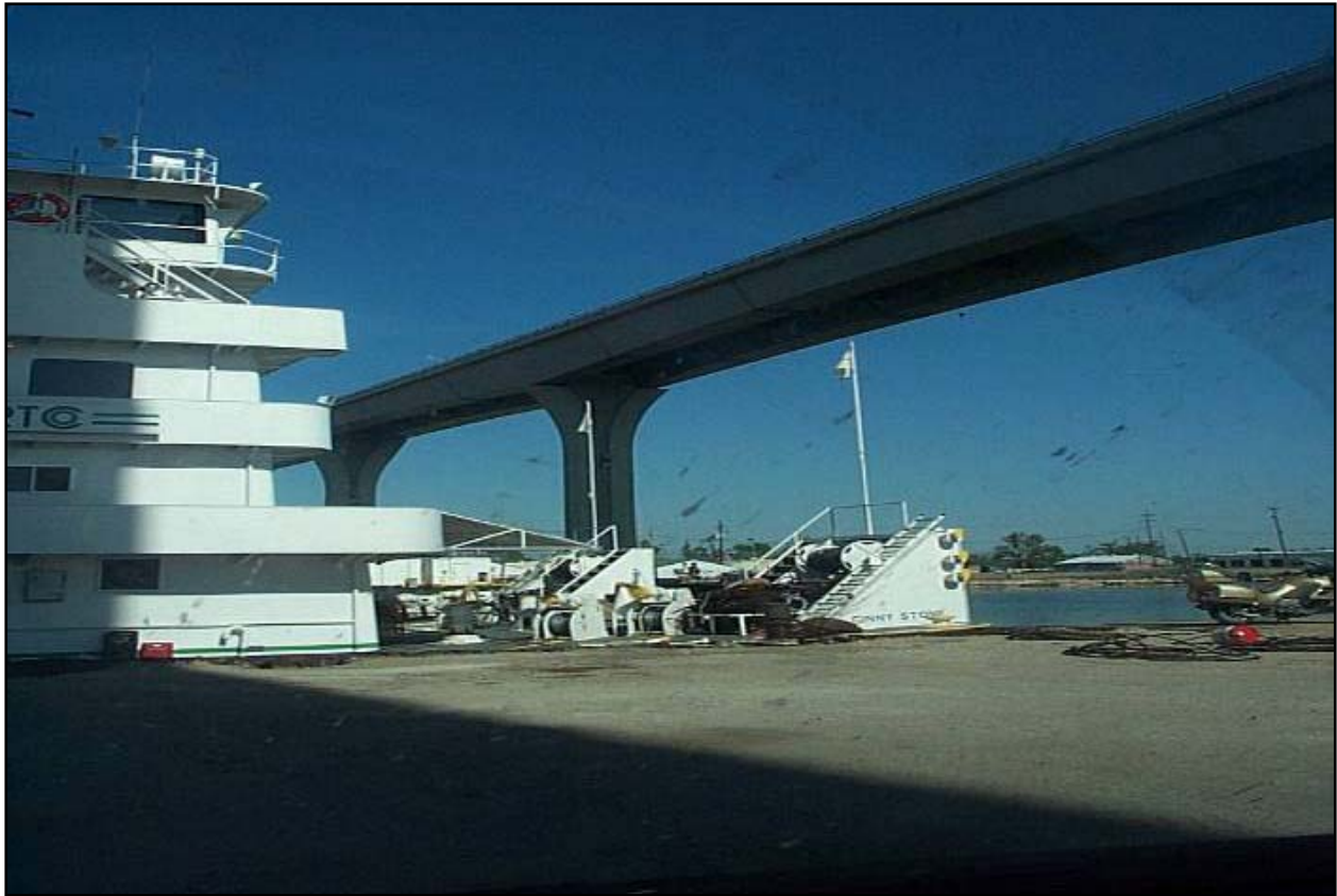
US 90 Bridge over Harvey Canal near Harvey Lock
