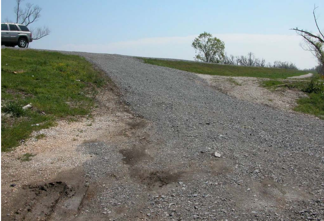
The Back Levee intersects the MRL after it crosses Hwy 23
