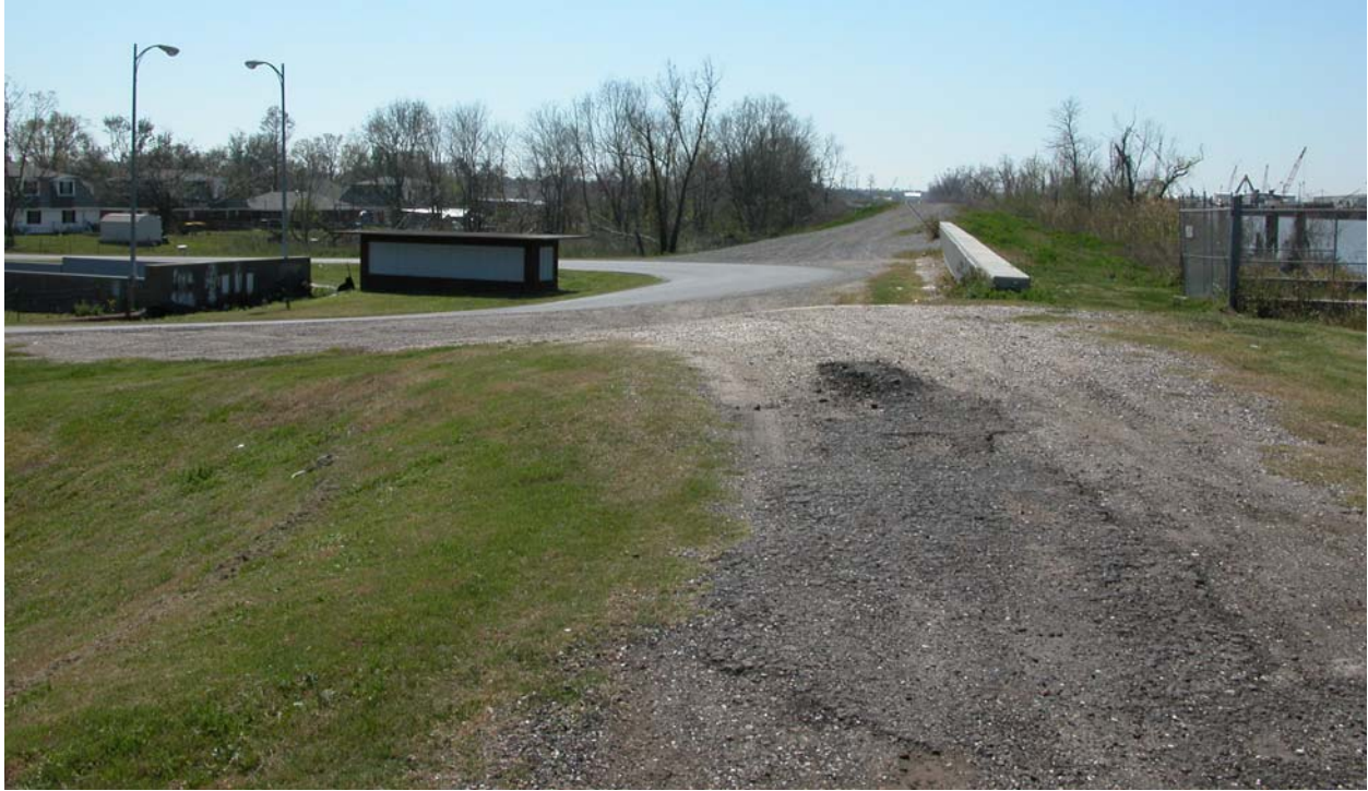
Highway 23 Tunnel under the GIWW
