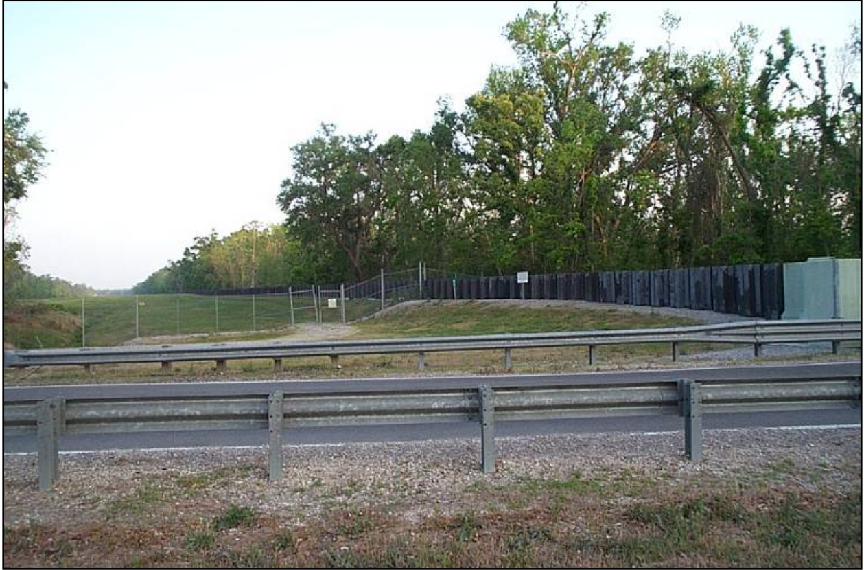
V-line levee continues south of LA Hwy 45 closure
