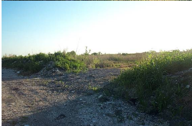
Local levee along site of proposed HPS levee
