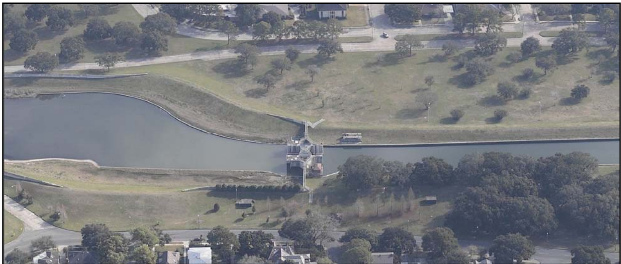
Protection Gate Structure at Bayou St. John
