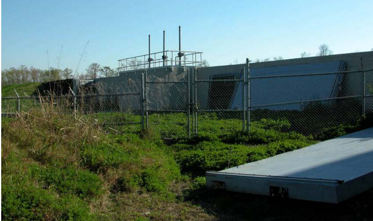
Trepagnier Drainage Structure
