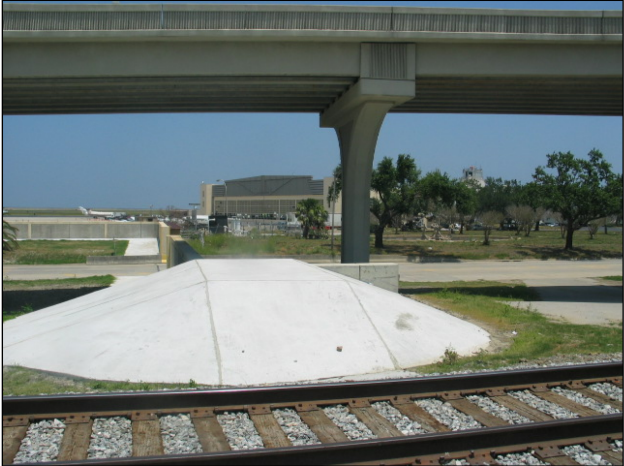
Figure NOE 23. Transition Improvements Between Reaches NOE 1&2 (Note: refer back to Figure NOE 5 taken from same location)
