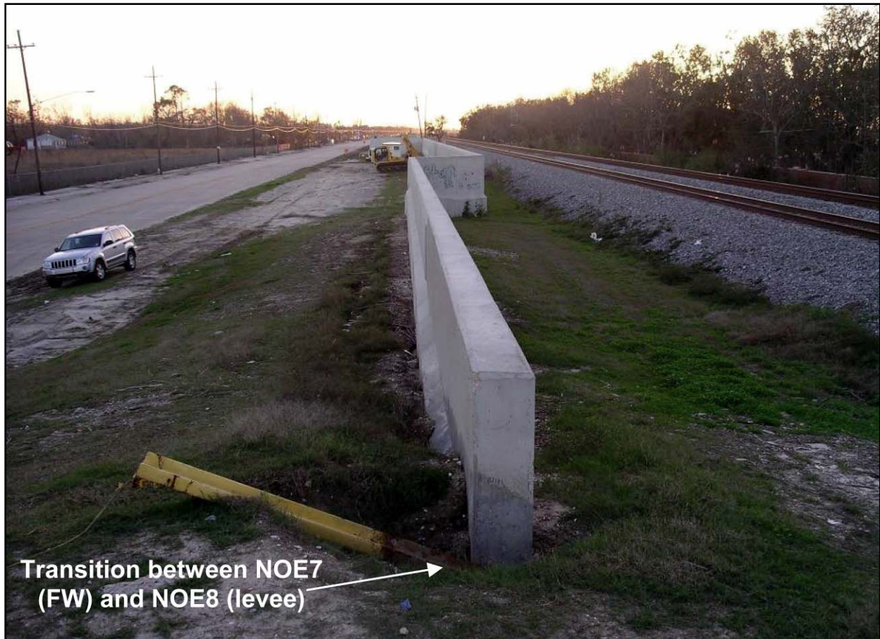
Figure NOE 8. Lincoln Beach Floodwall (Reach NOE7) (Looking west from Reach NOE8)
