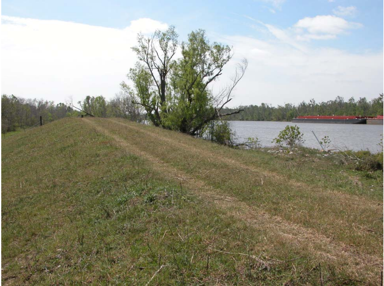
Typical levee section along the GIWW
