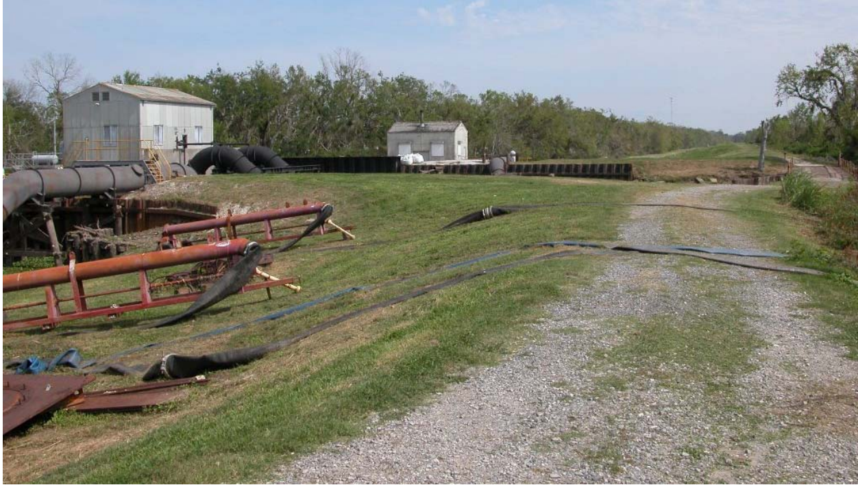
Ollie Pump Station
