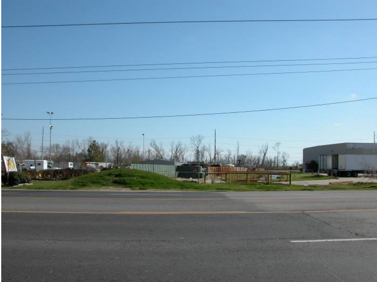
St. Charles – Jefferson Parish Boundary Levee South of US 61 Highway – no closure at this crossing
