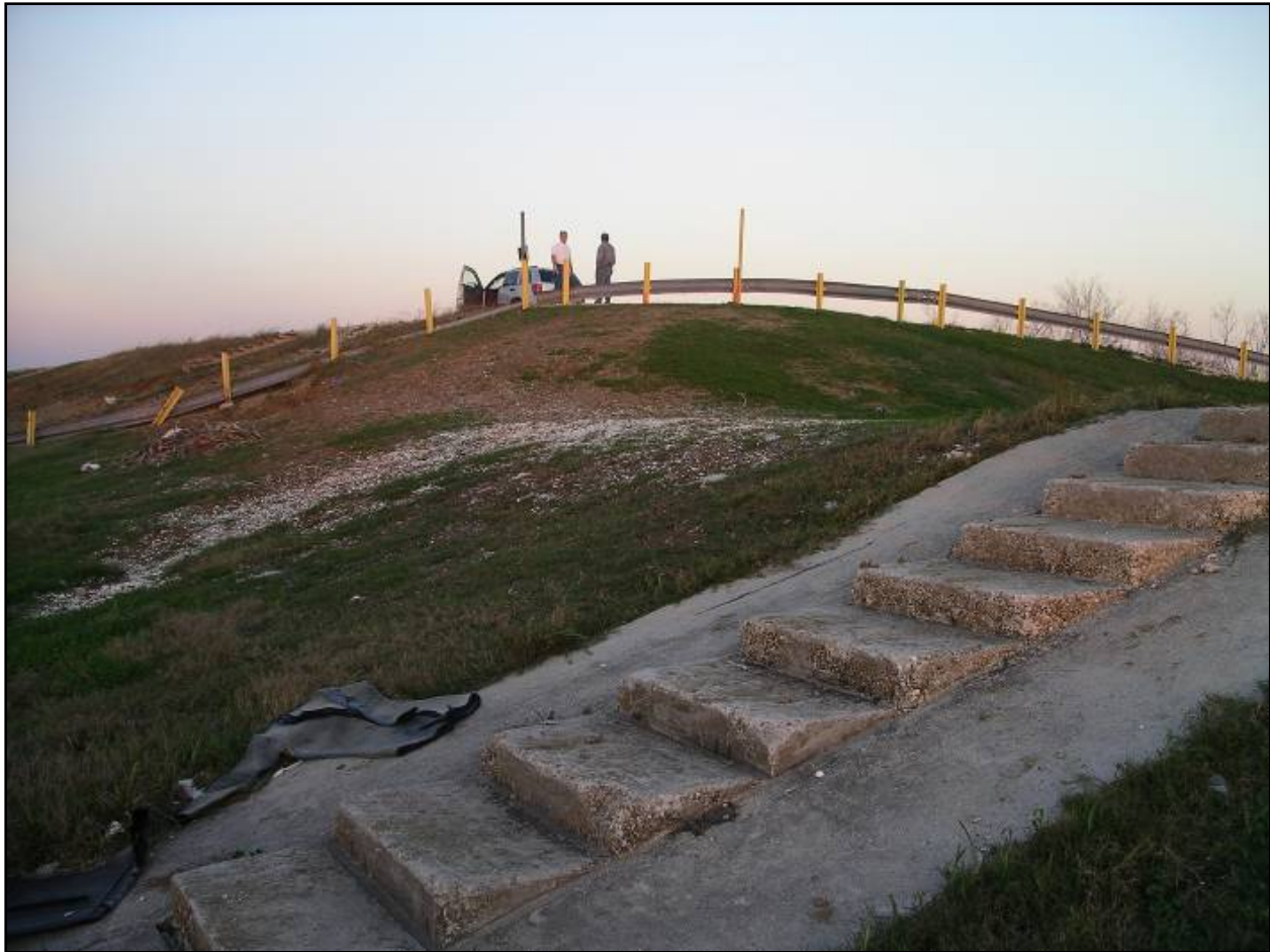
Figure NOE 9. Begin Lakefront Levee at Citrus Lakefront and Paris Road (Lakefront Levee @ El. 18.6 +/- and Citrus Lakefront Levee @ 12.6+/-)
