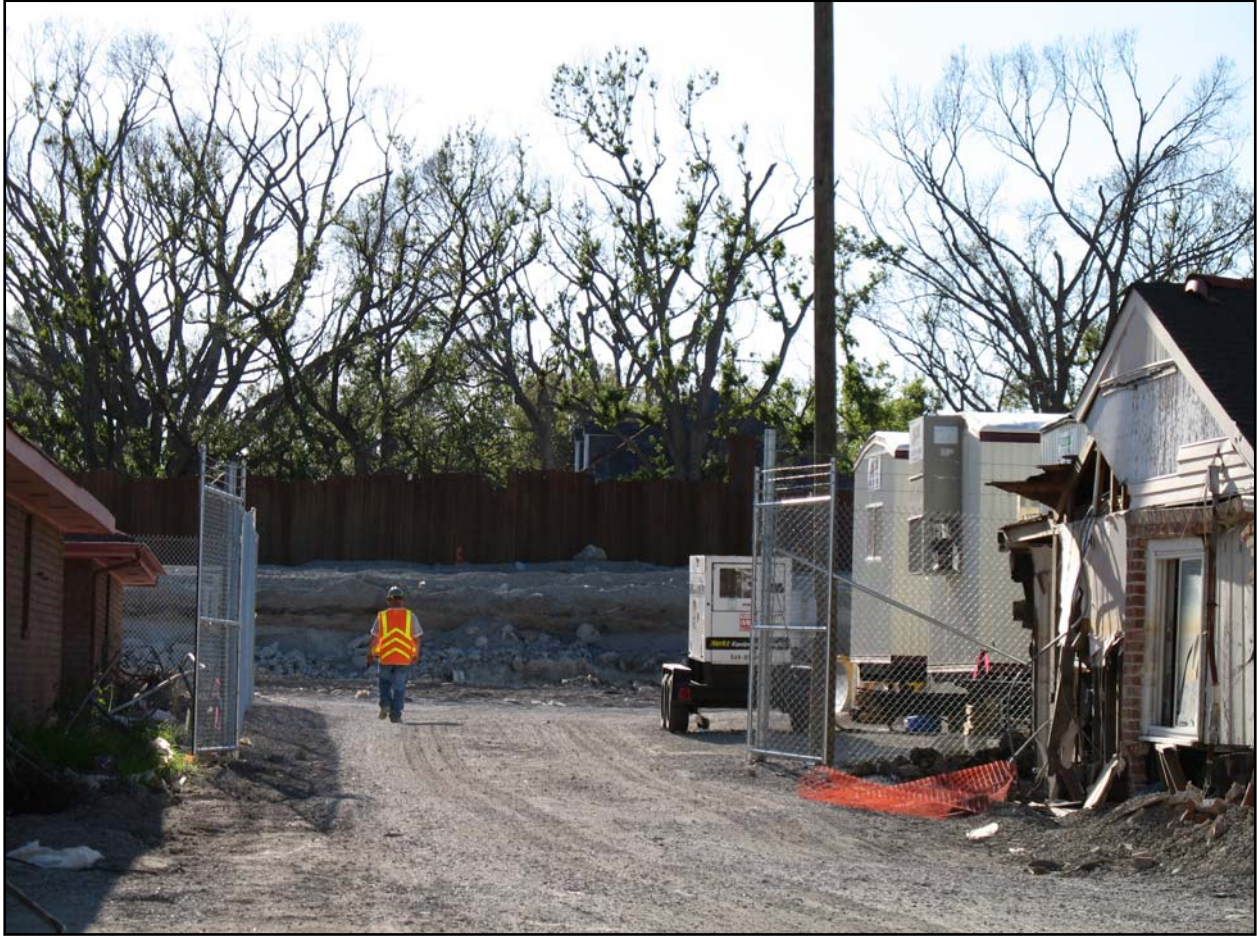
Figure 5. Sheetpile repair along the London Ave Canal – East Side Failure
