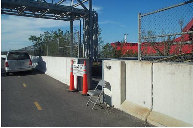
Typical closure gate (vehicle and pedestrian) along MRL
