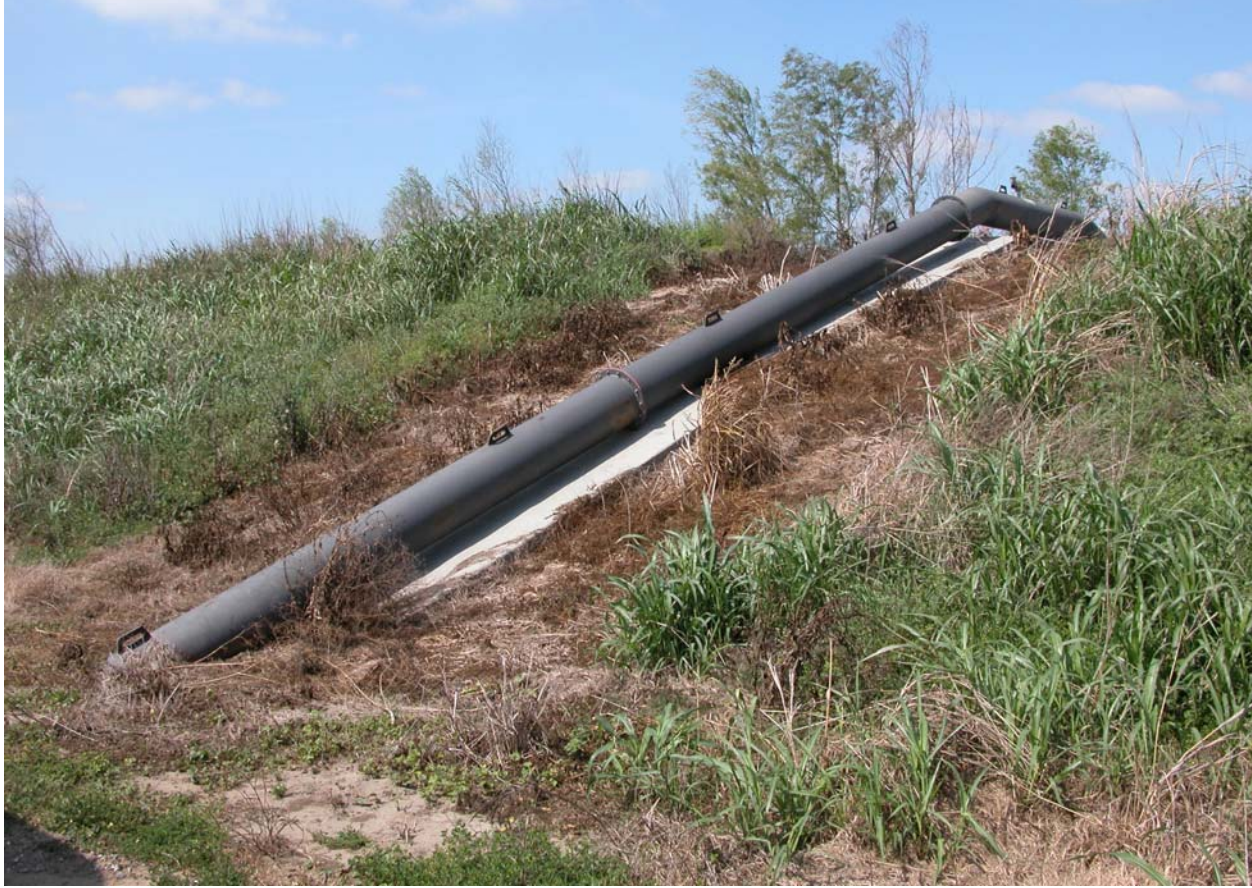
Pipe crossing over the GIWW levee
