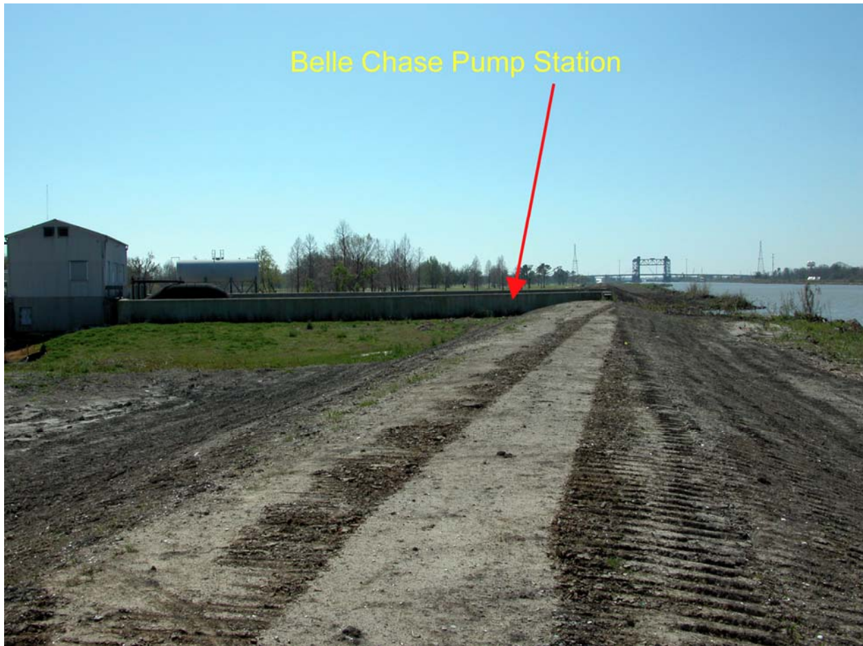
Going south along the GIWW to the Belle Chase Pump Station.
