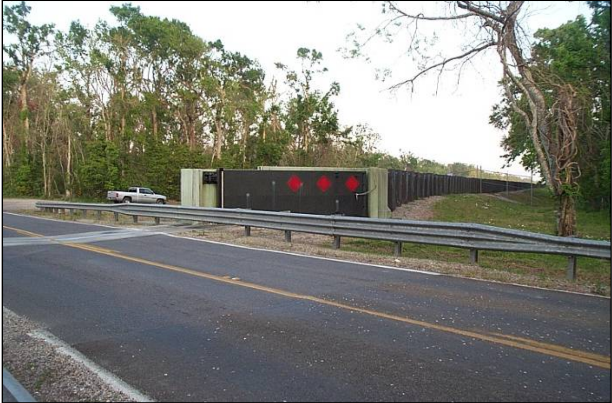
Double Swing gate at the LA Hwy 45 closure in the V-Line levee
