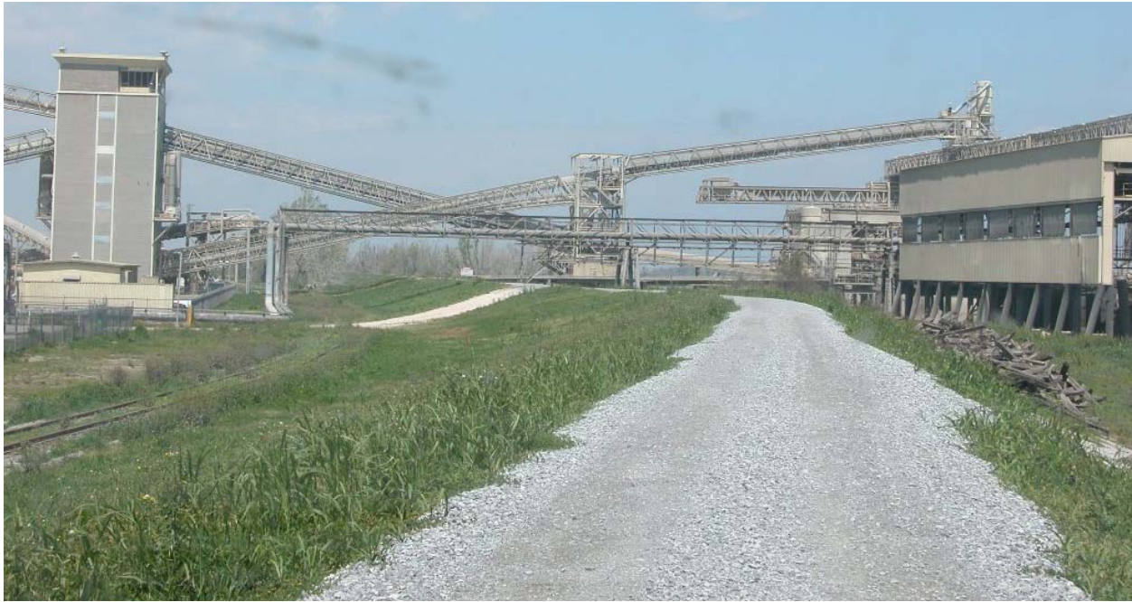
A number of off-load facilities are located along this portion of the MRL, similar to this grain loading facility
