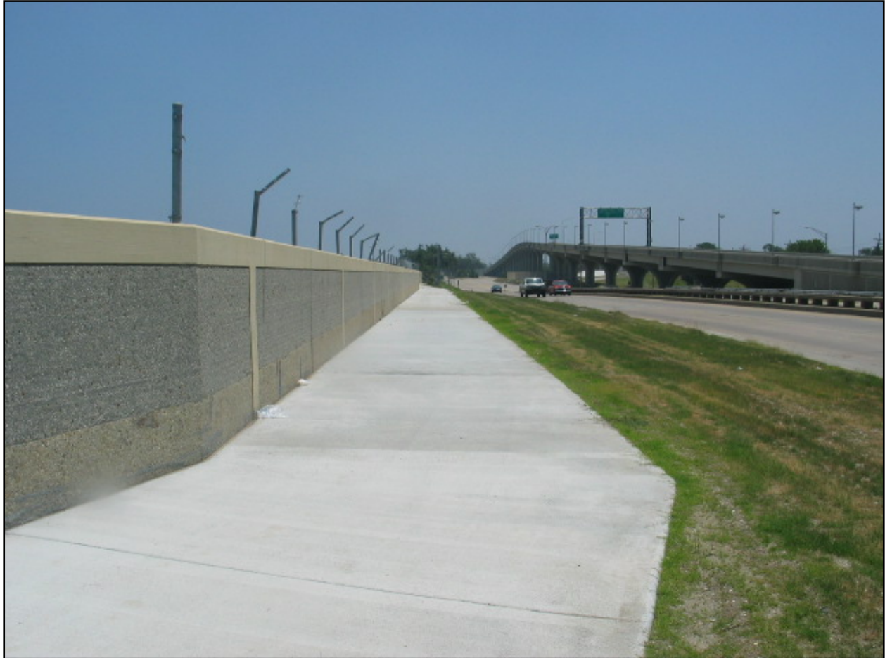
Figure NOE 22. Scour Protection Pad Behind Lakefront Airport FW
