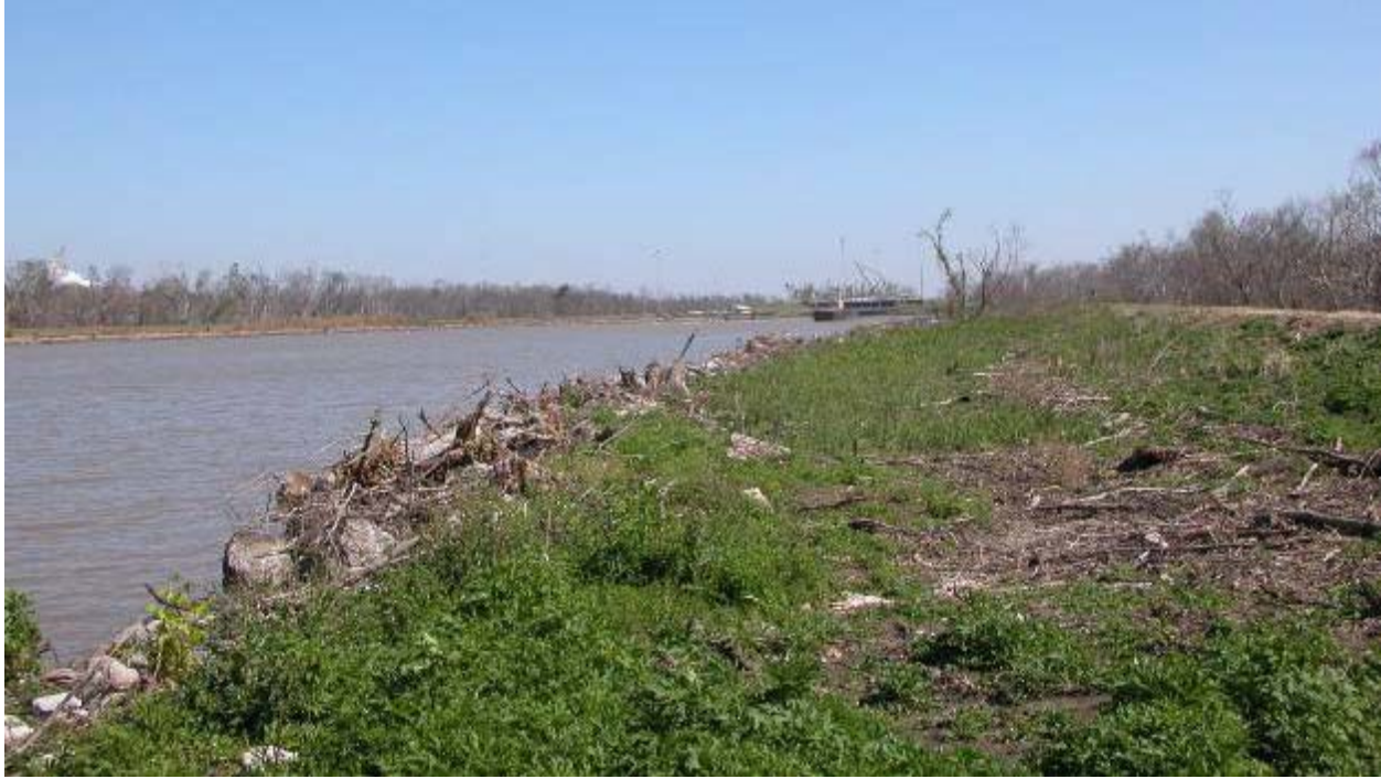
Typical Algiers Canal levee; no armor
