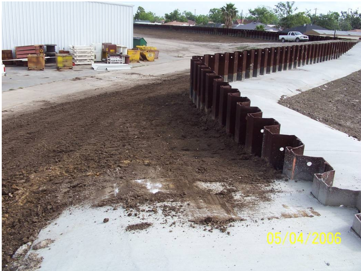
Figure STB 38. Scour repairs to Caernarvon sheetpile I-wall area (Note: compare to pre-Katrina condition shown in Figure STB 18)
