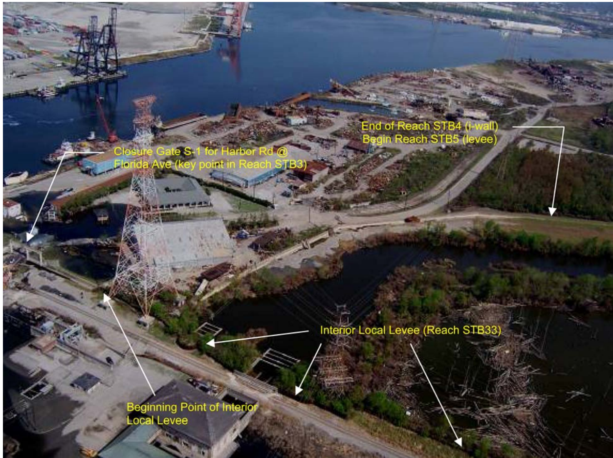
Figure STB 23. Area showing beginning of interior local levee at the IHNC
