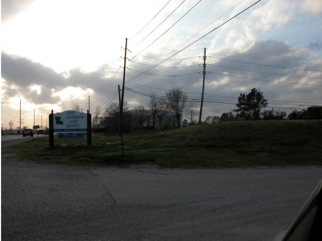
St. Charles – Jefferson Parish Boundary Levee ends North of US 61 Highway – gap at this crossing
