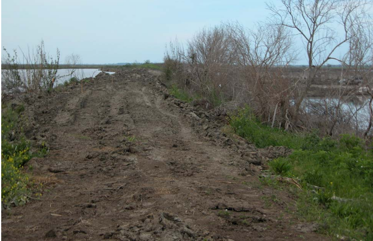
Citrus Lands Back Levee repairs to breach
