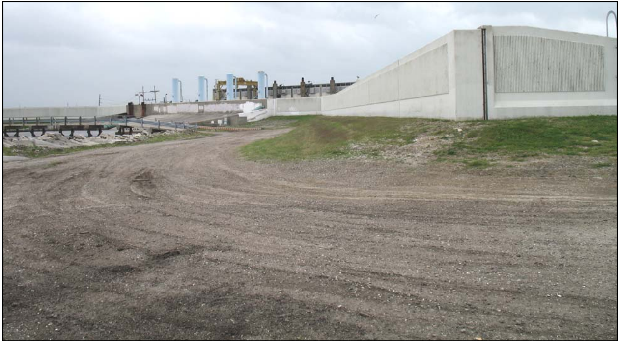
Duncan Canal Pump Station
