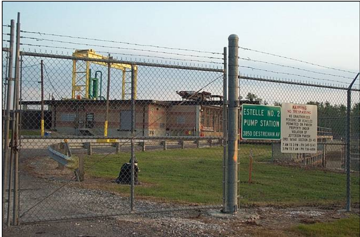
New Estelle Pump Station
