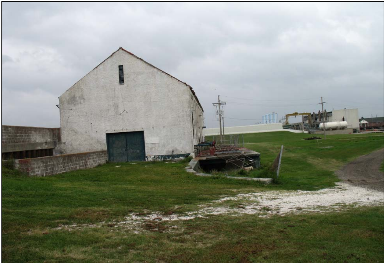
Foreground: Original Pump Station and old masonry wall (not in Service) Background: Duncan Pump Station with new T-walls
