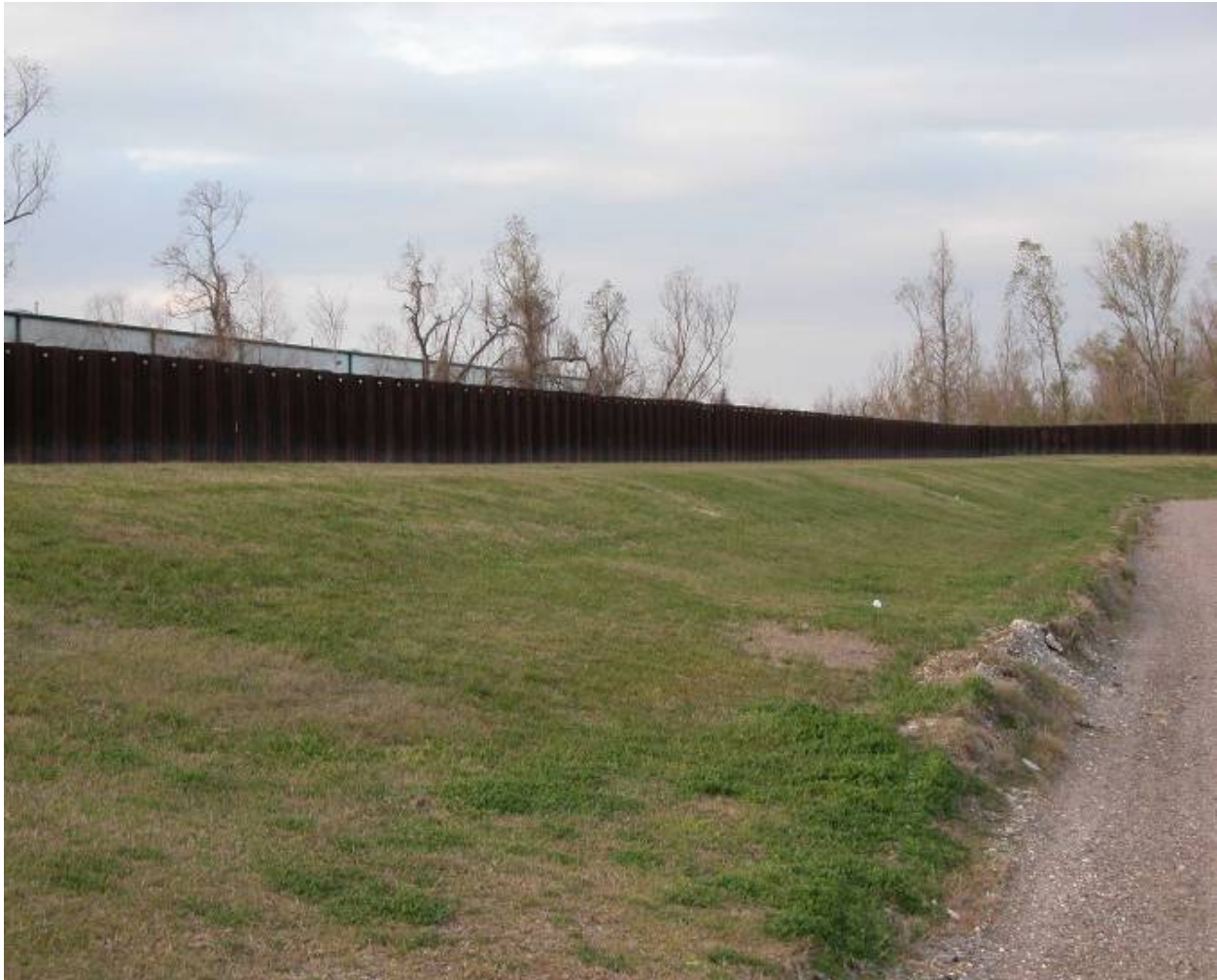
Floodwall as it turns east by the Airport runway extension
