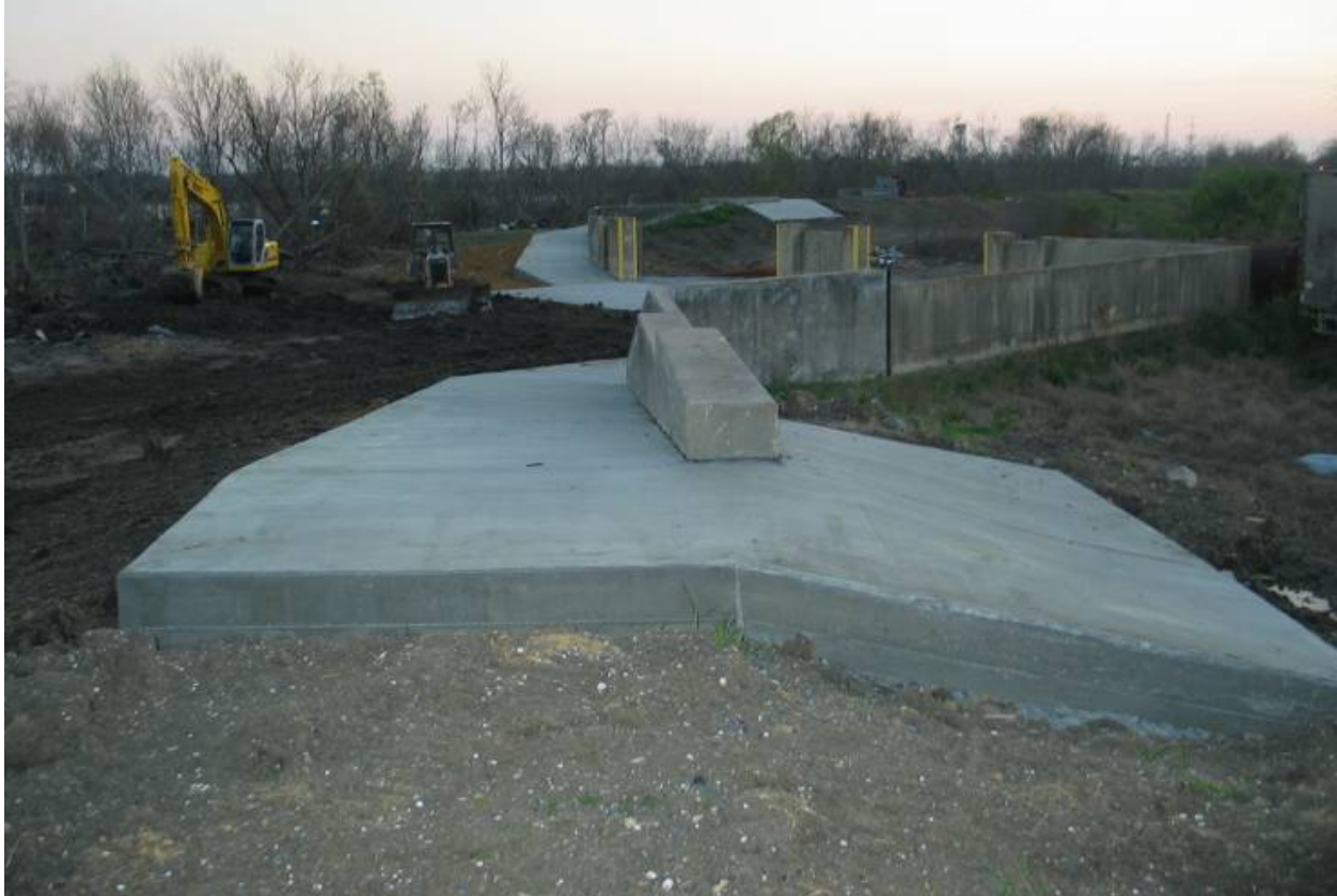
Figure STB 31. New scour protection around Reach STB6
