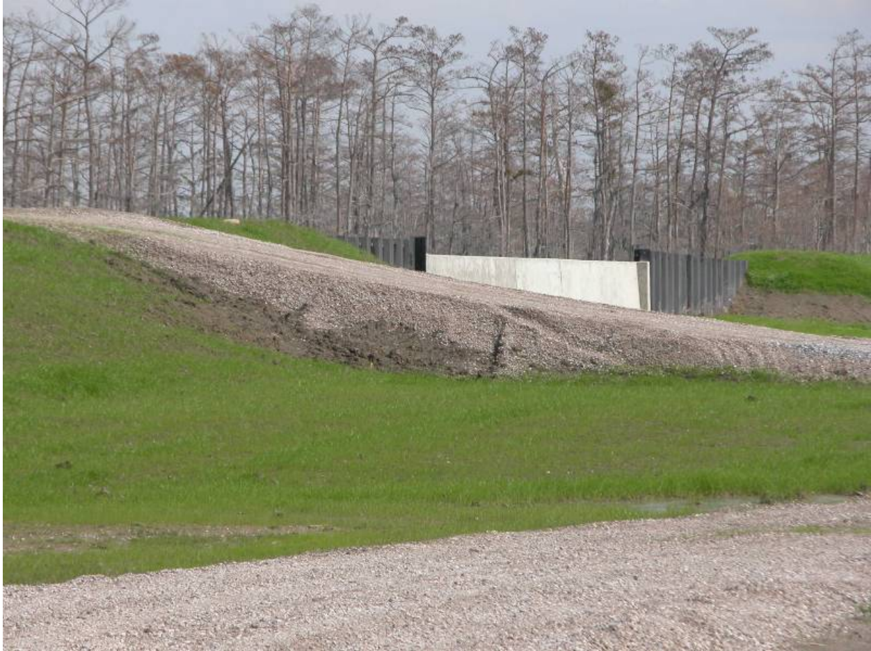
Pipeline Crossing with sheetpile transition to levee
