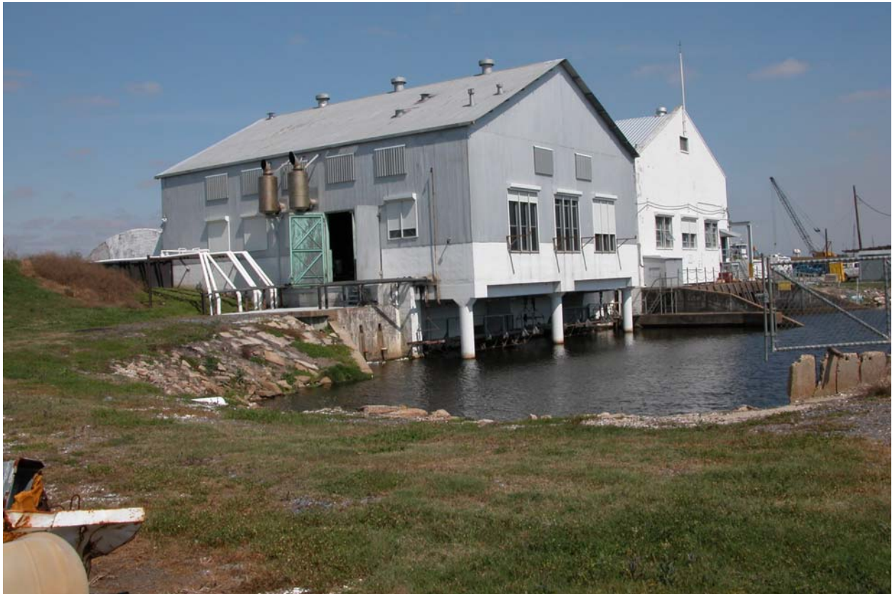
Plaquemines Pump Stations 1 and 2
