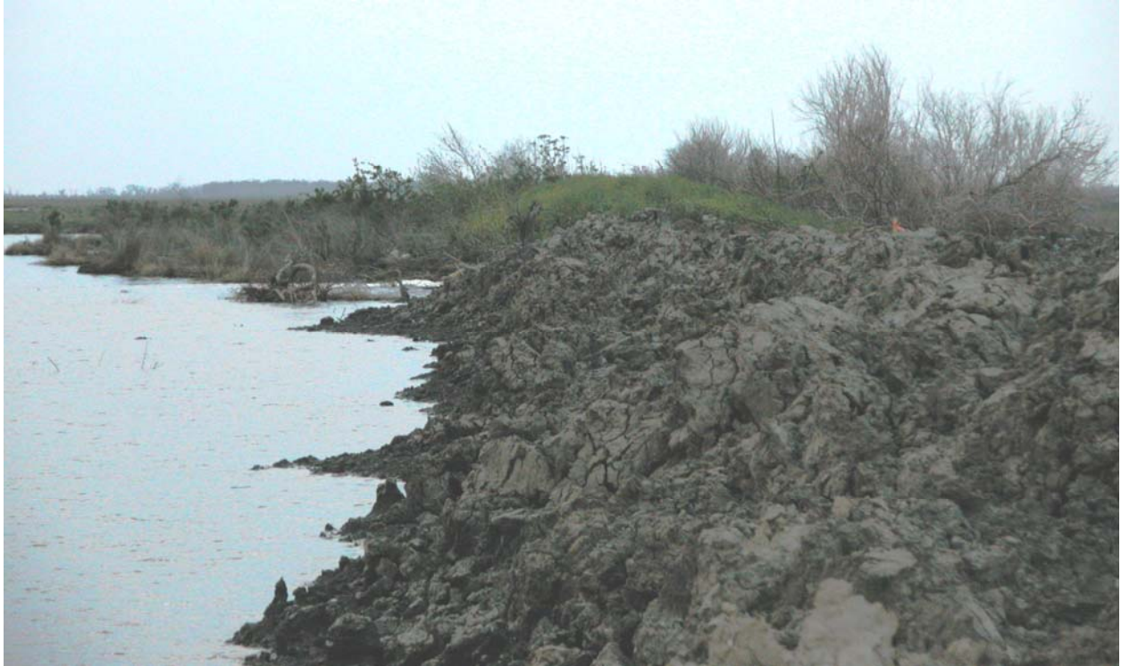
Citrus Lands Back Levee repairs to breach
