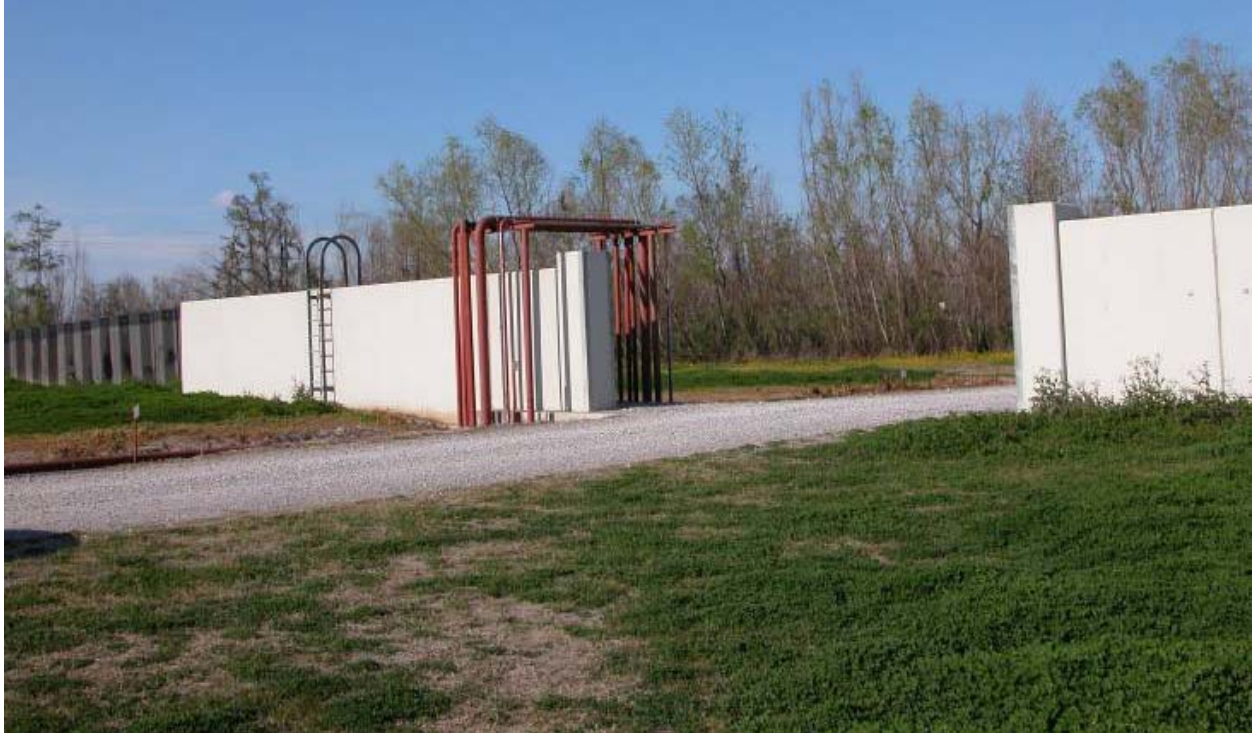
Industrial access road closure gate
