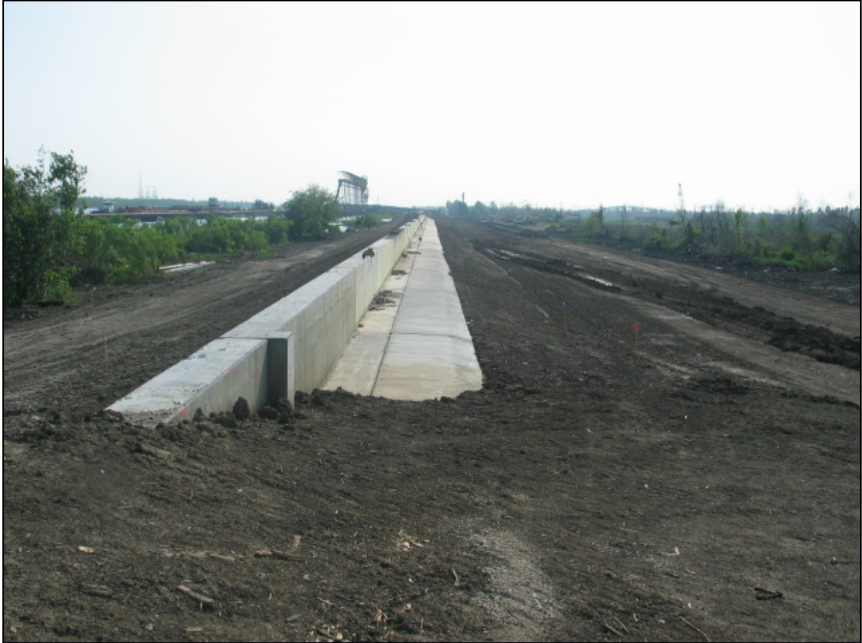
Figure NOE 35. New L-Wall at Bulk Loading Facility
