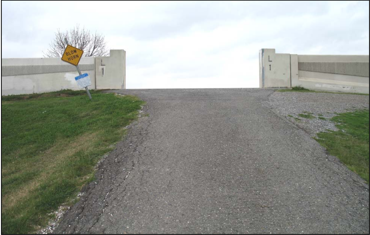
Gate L1 – Lakefront Levee
