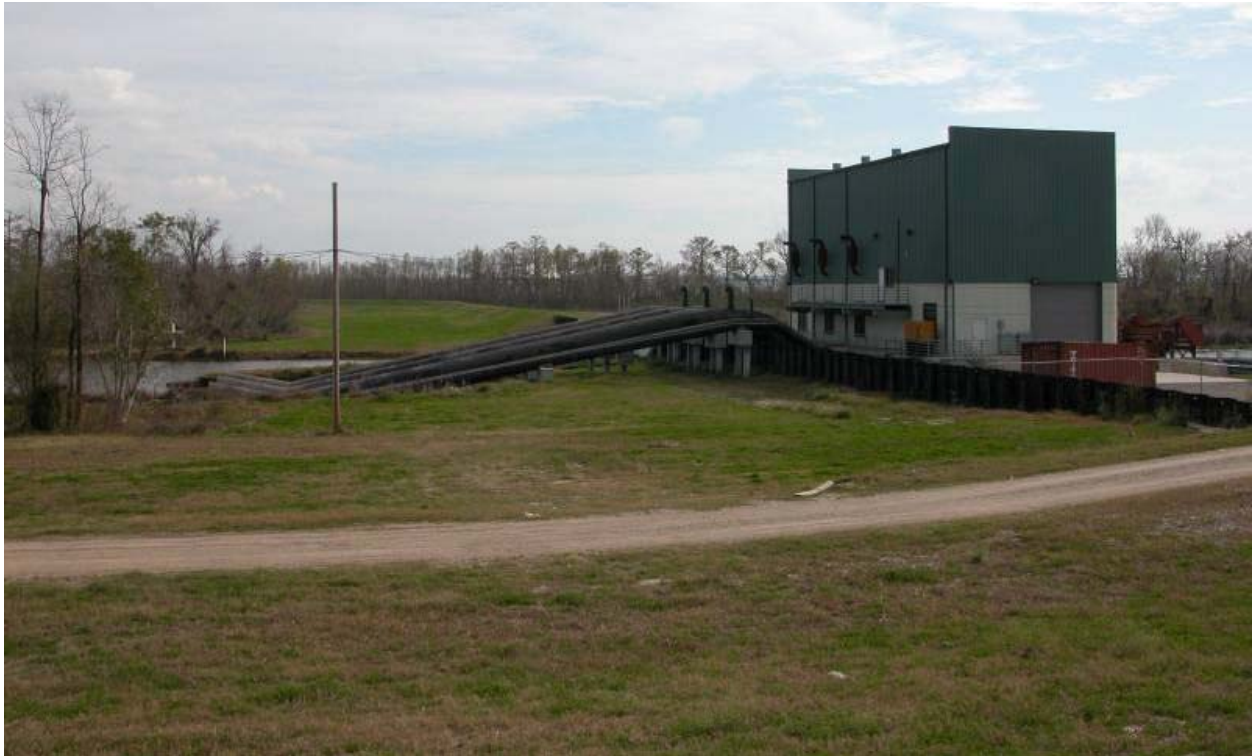
Trepagnier Pump Station
