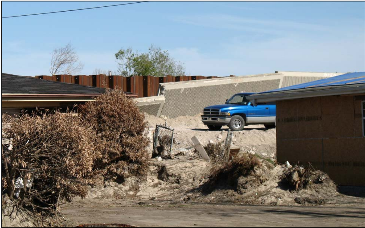
Figure 6. Sheetpile repair along the London Ave Canal – West Side Failure
