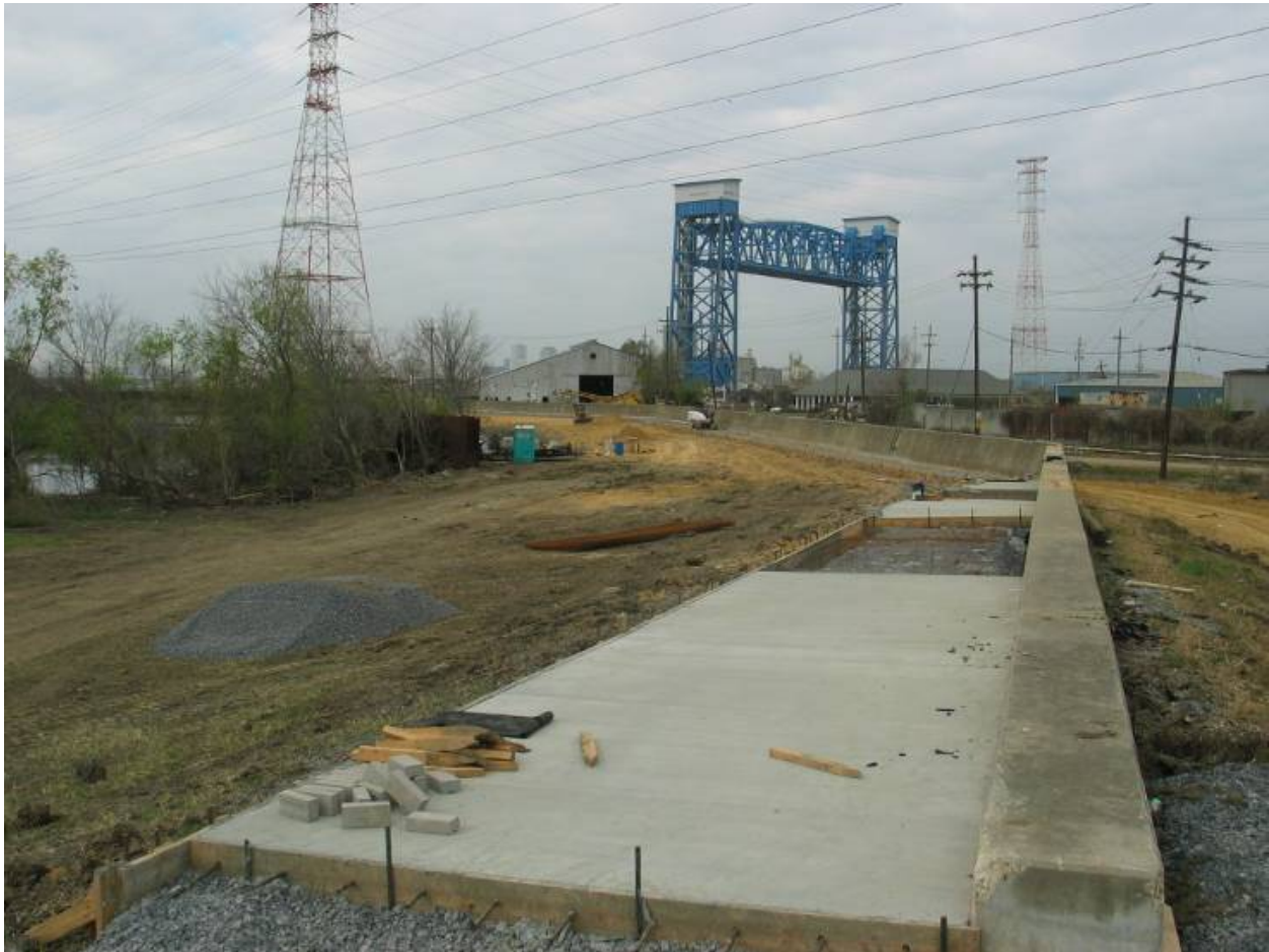
Figure STB 30. New scour protection pad (typical) (photo taken at end of Reach STB4 looking back toward IHNC)
