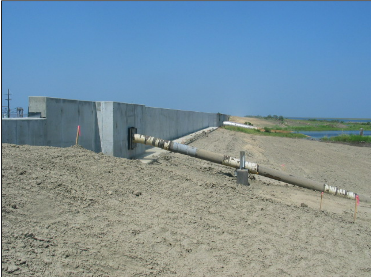
Figure NOE 30. Repaired Floodwalls Around Pump Station #15
