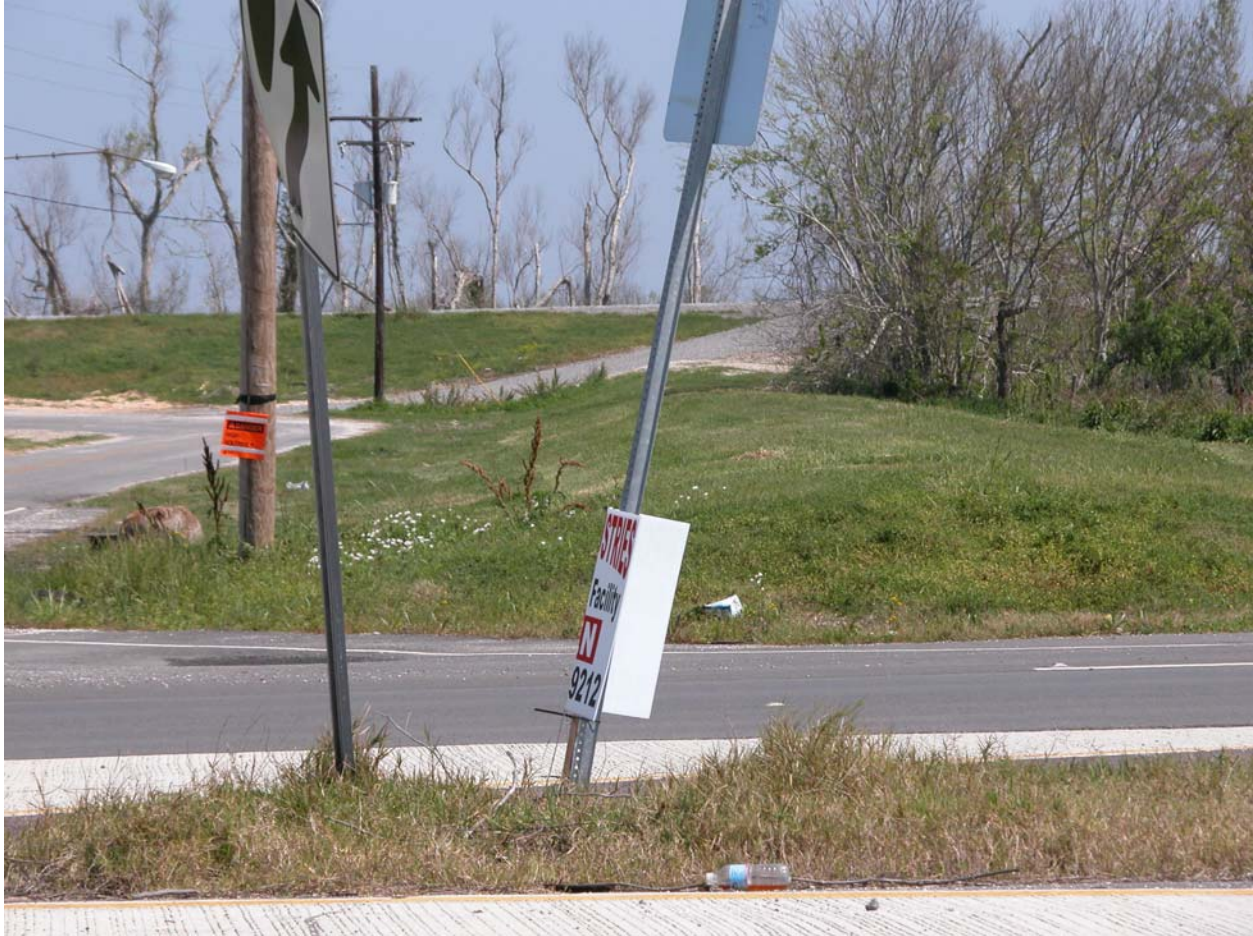
PL 11 Back levee intersects Hwy 23 north of Jesuit Bend
