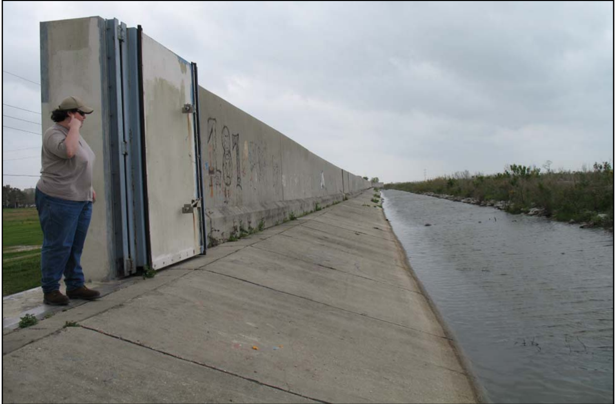
Typical T-wall and slope protection on floodside in Reach 3
