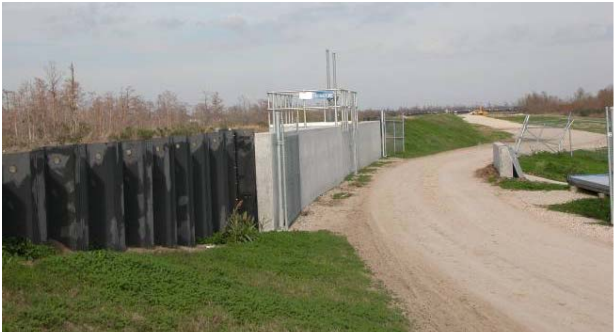
Walker Drainage Structure with sheetpile transition
