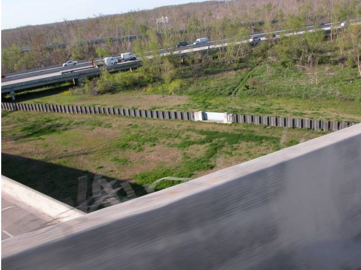
I-310 Floodwall access closure gate (normally closed) with 24-ft closure gate
