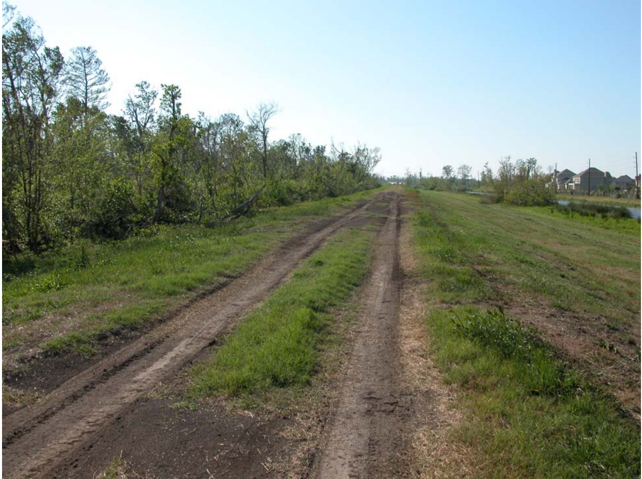
Back levee continues outside U.S. Coast Guard toward GIWW Station
