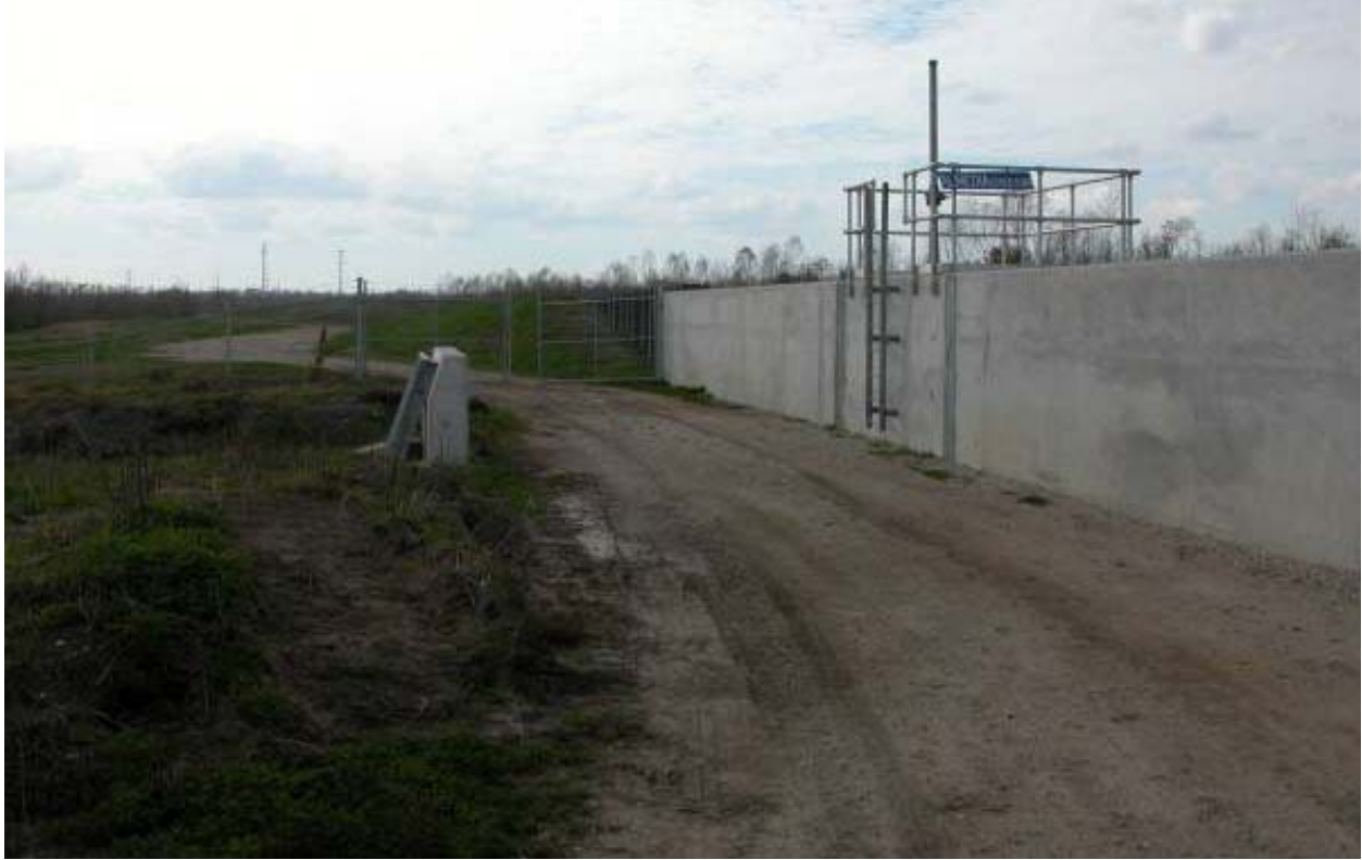
Alemedia Drainage Structure
