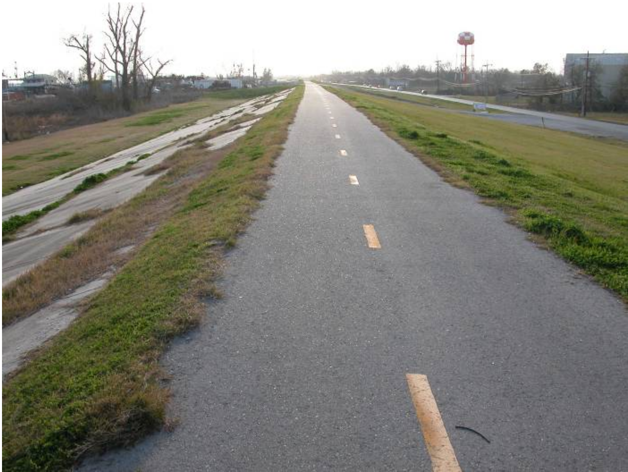
Top of Mississippi River Levee at the St. Charles-Jefferson boundary
