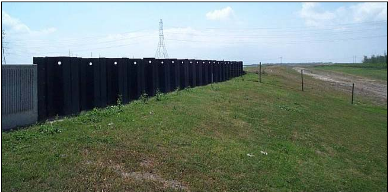
Figure 19. I-wall transition to concrete structure and levee.
