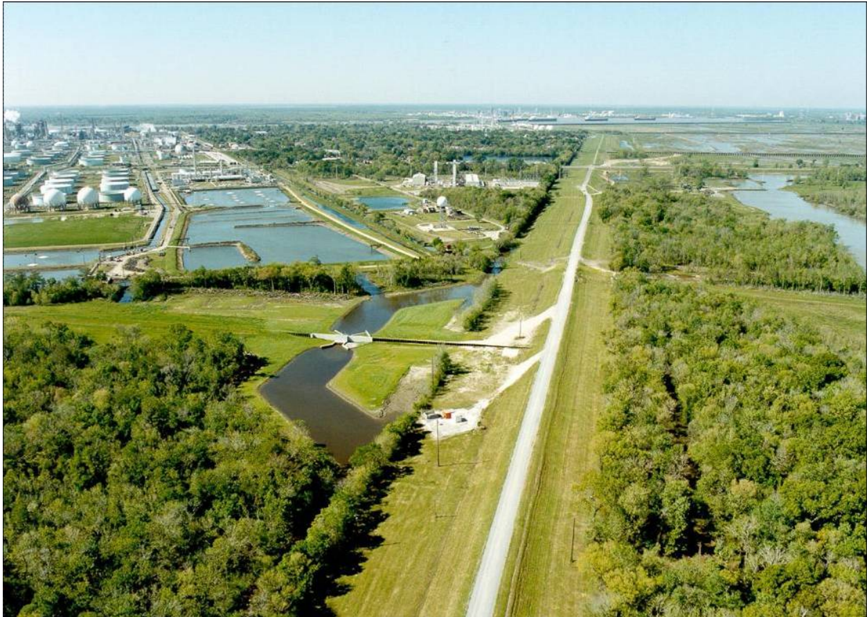
Figure 5. Typical New Orleans levee.
