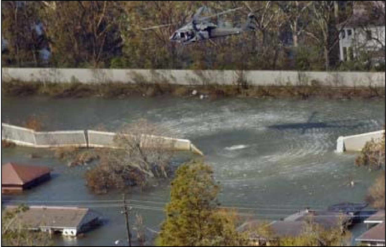
Figure 12. Katrina damage to concrete capped I-wall.
