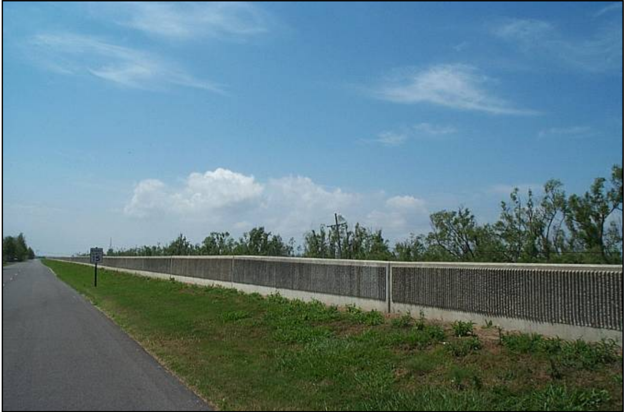
Figure 9. Concrete capped I-wall.
