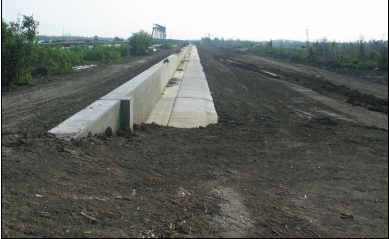
Figure 15. Typical L-wall.
