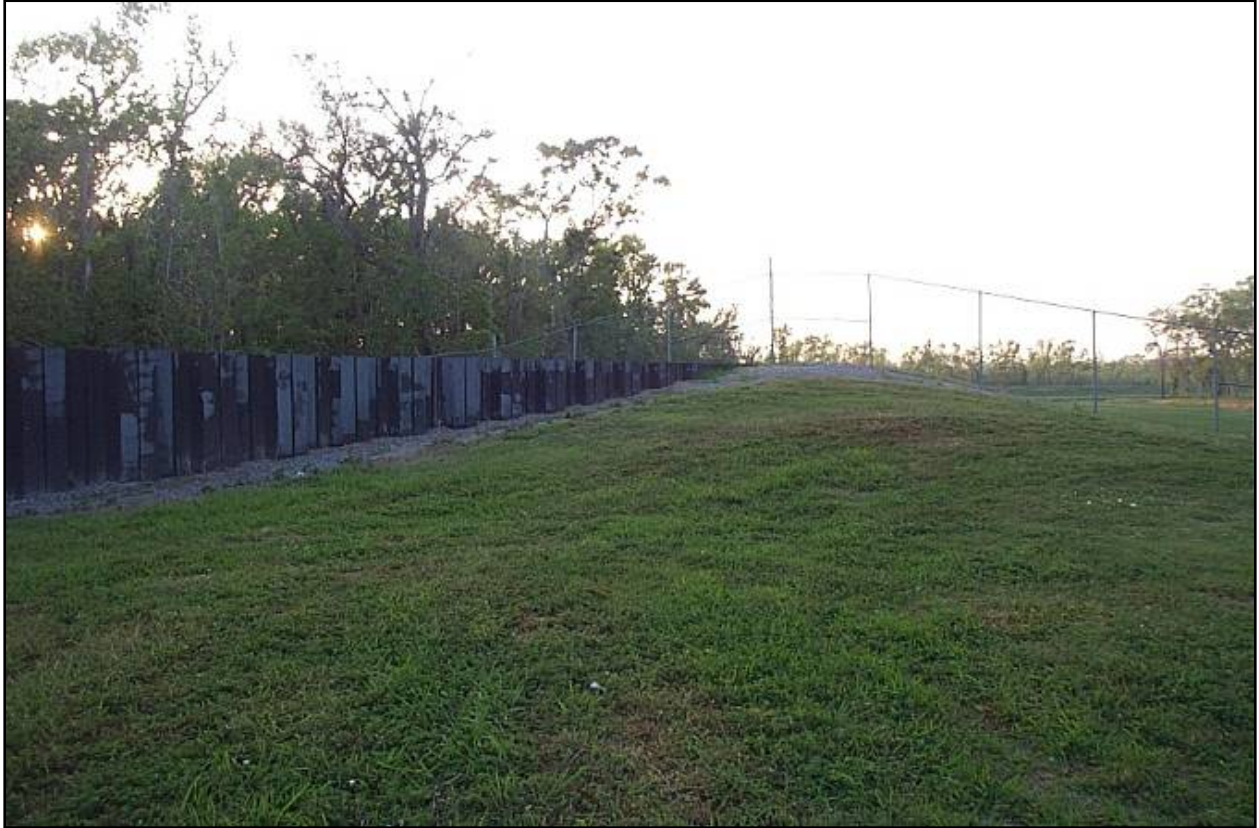
Sheet pile transition at the LA Hwy 45
