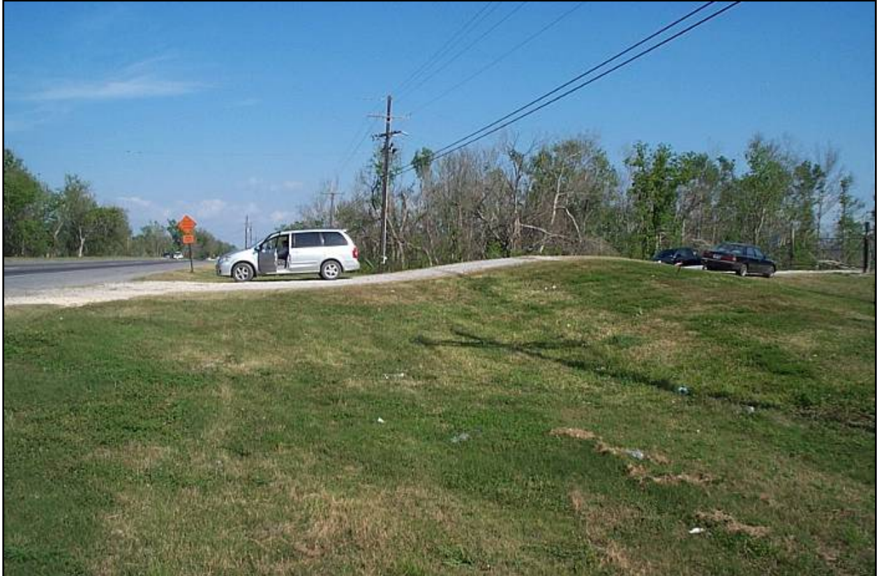
Levee begins at Hwy 90
