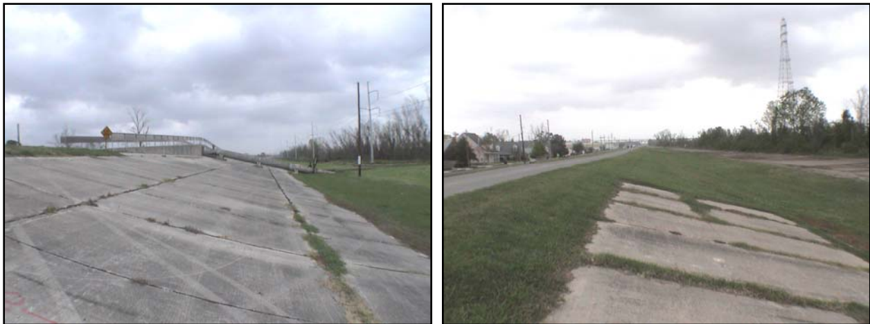
Flood side of MRT in East Jefferson Parish (Note: Concrete scour protection and asphalt roadway on crown)
