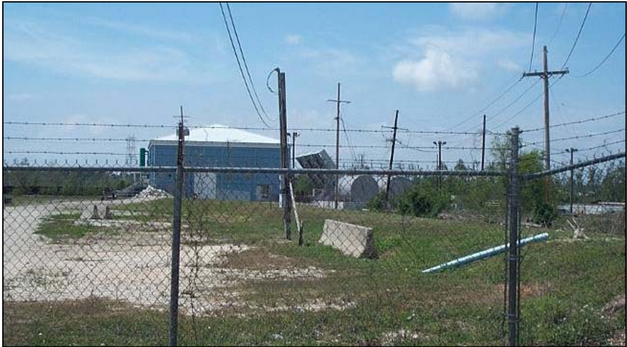
Cataouatche Pump Station
