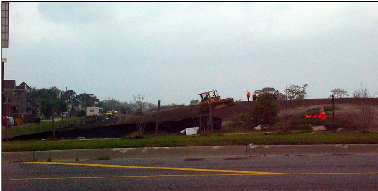
Reconstruction of a Portion of Reach 7 Lakefront Levee
