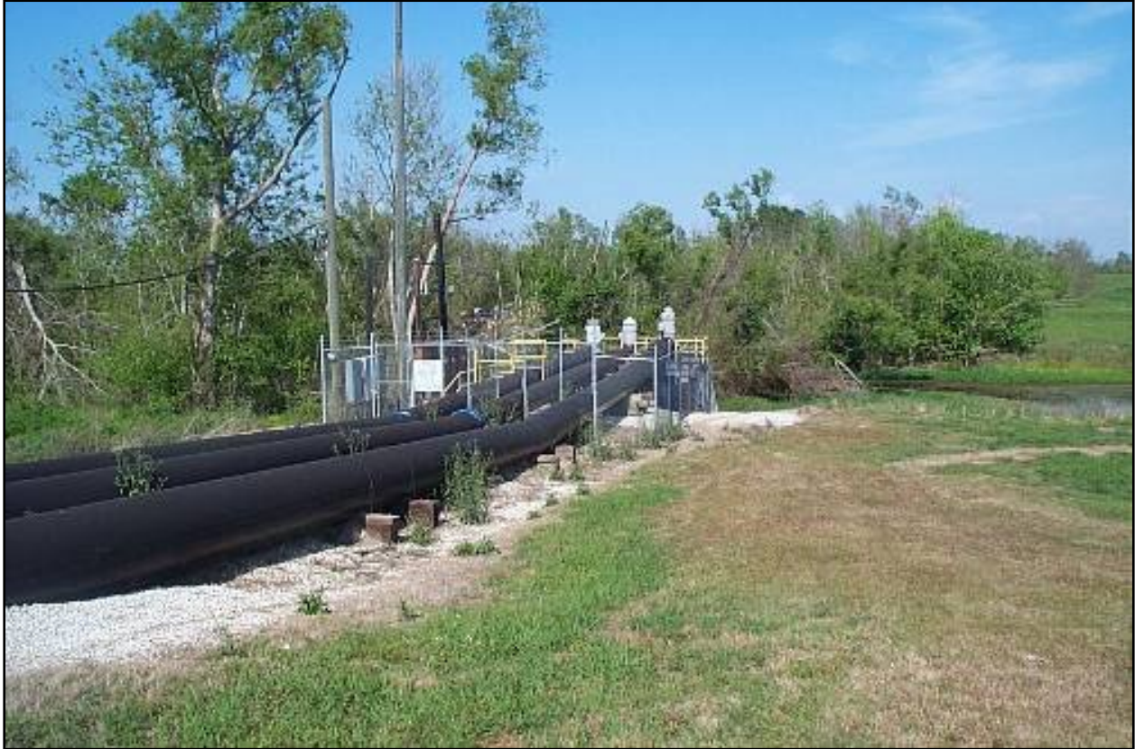
Pump station near Hwy 90 with pipe crossing over levee
