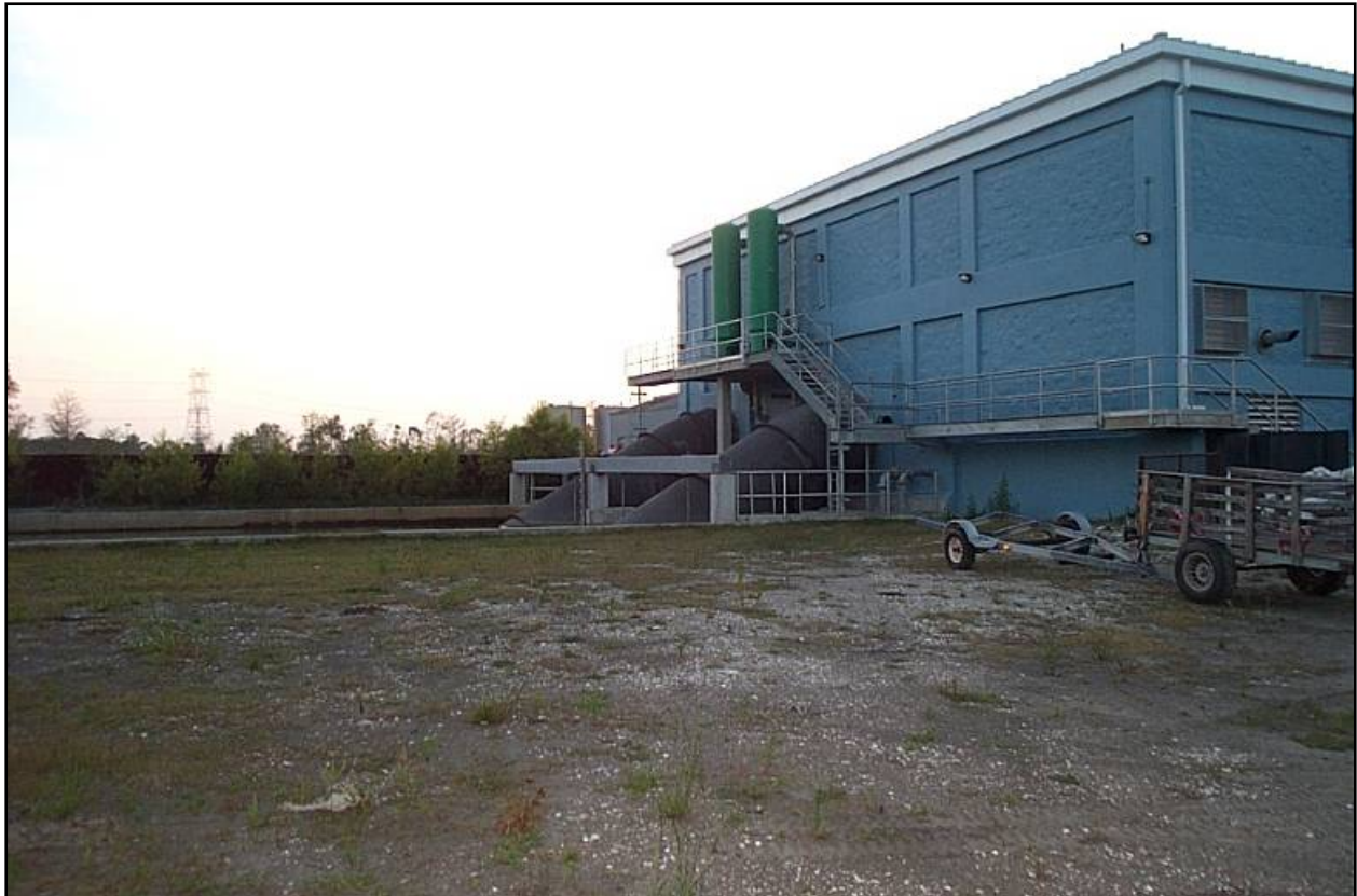
Segnette Pump Station
