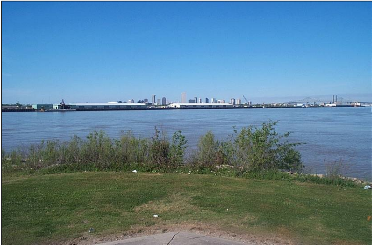
MS River Levee at exit of Harvey Canal
