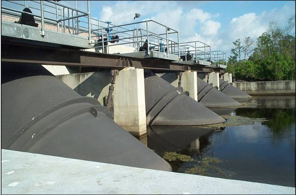
New Westminster Pump Station
