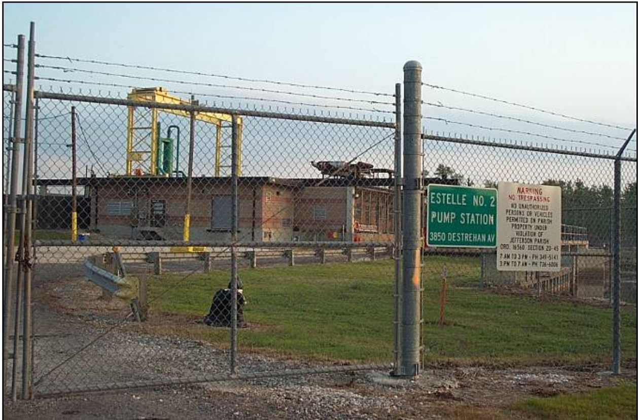
New Estelle Pump Station
