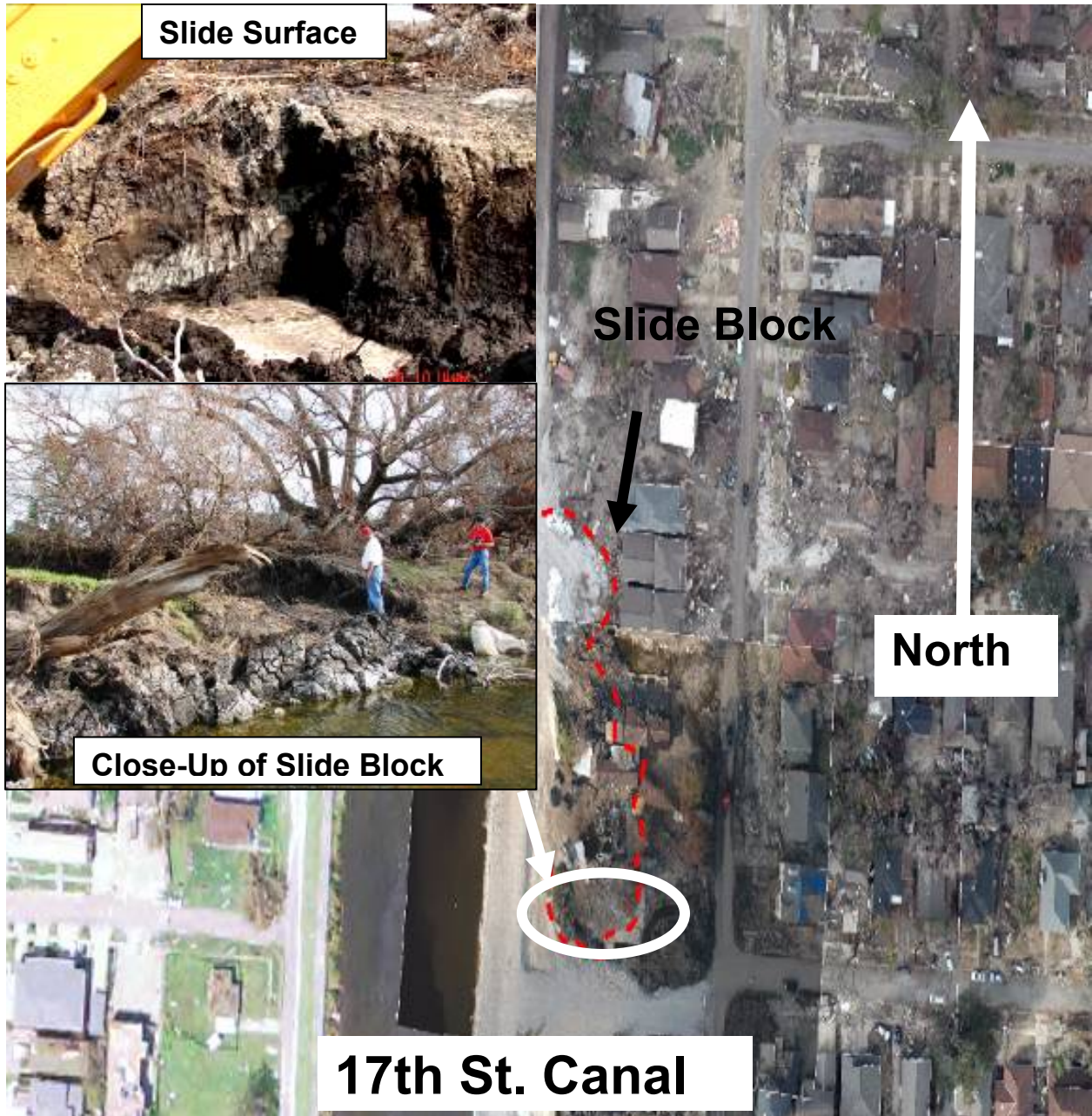
Figure 16. Photographs taken at the 17th Street Canal breach after the failure.
