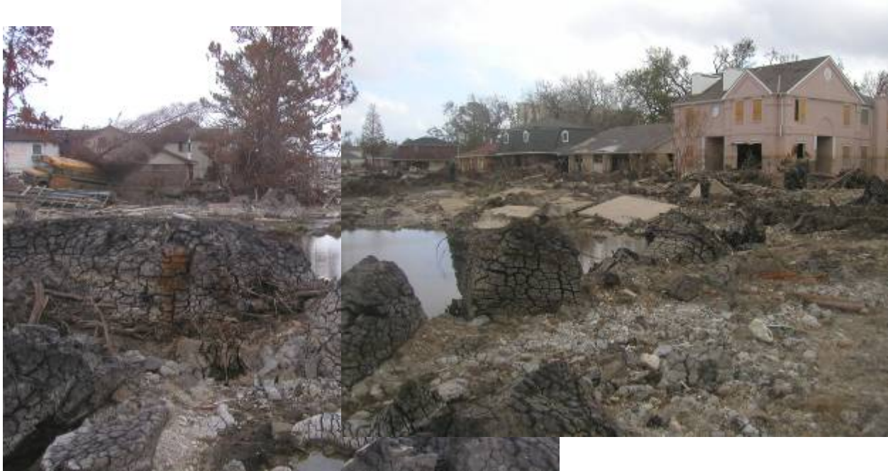
Figure 14. Marsh blocks from the levee embankment at the 17th Street Canal breach.
