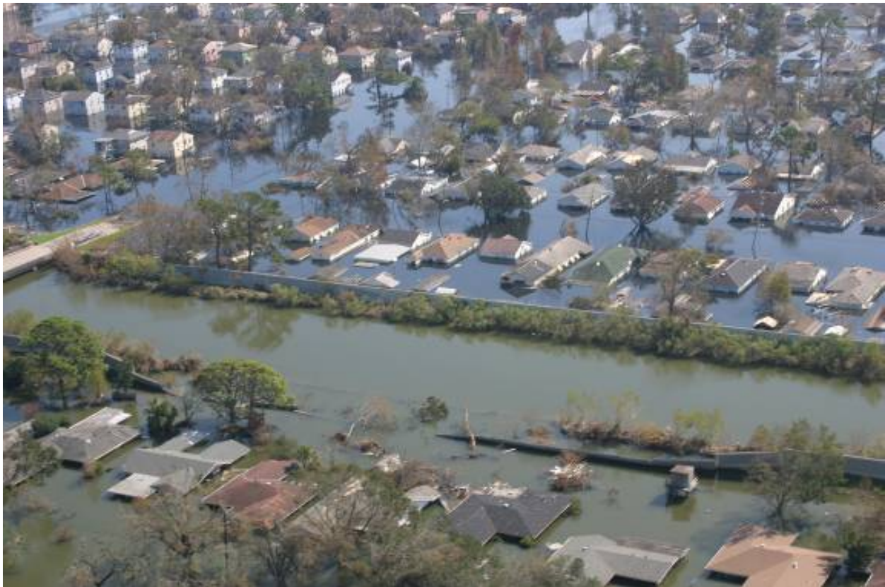
Figure 36. North breach, London Avenue Canal.
