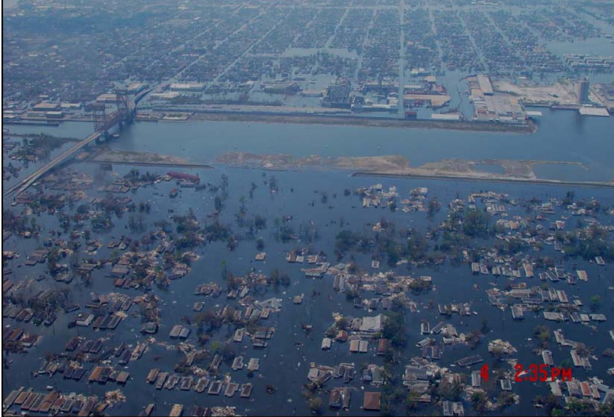
Figure 80. Aerial photo of the breached floodwall along the eastern side of IHNC adjacent to the Lower Ninth Ward.
