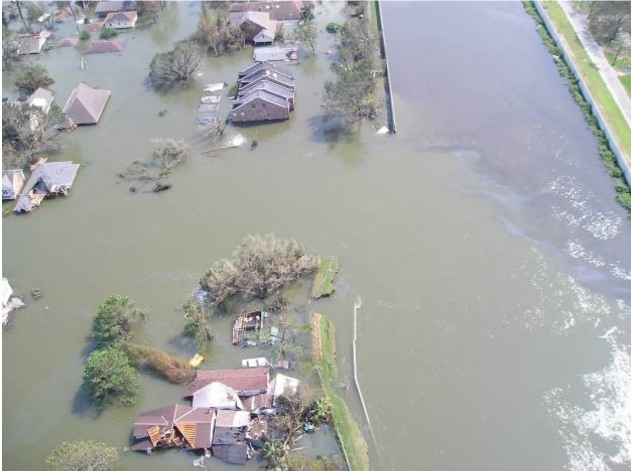
Figure 10. Aerial photograph of the 17th Street Canal breach showing I-wall and embankment translation.
