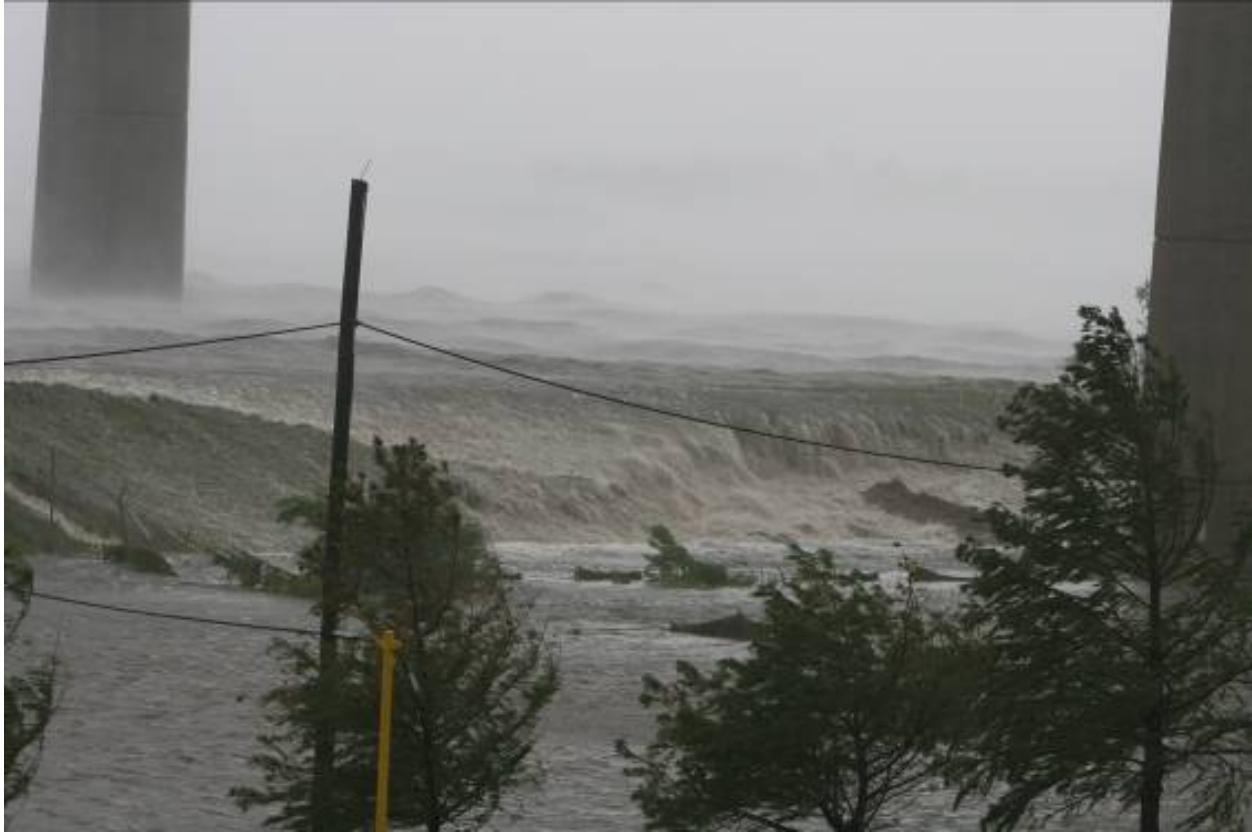
Figure 95. Overtopped levee under the Paris Road Bridge adjacent to the Entergy power plant in New Orleans East, during Hurricane Katrina.
