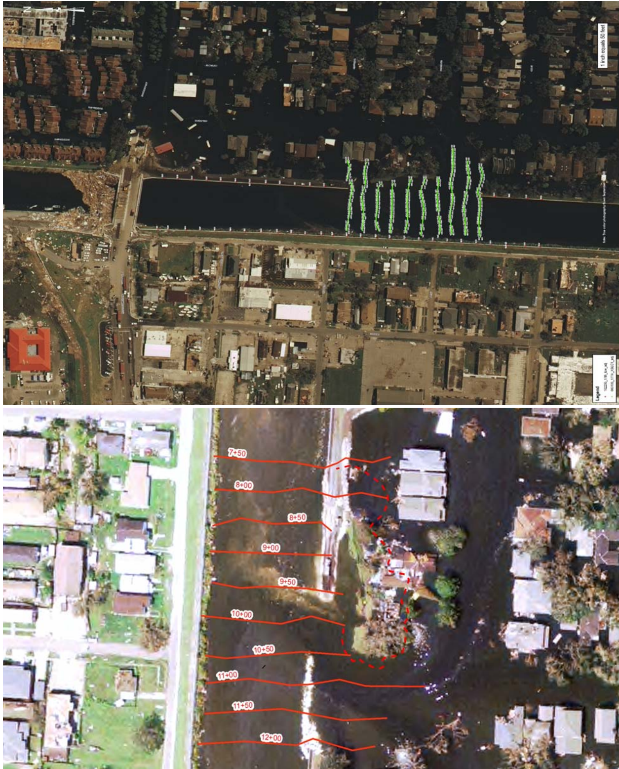
Figure 11. Location of multi-beam sonar survey cross sections at the 17th Street Canal breach.
