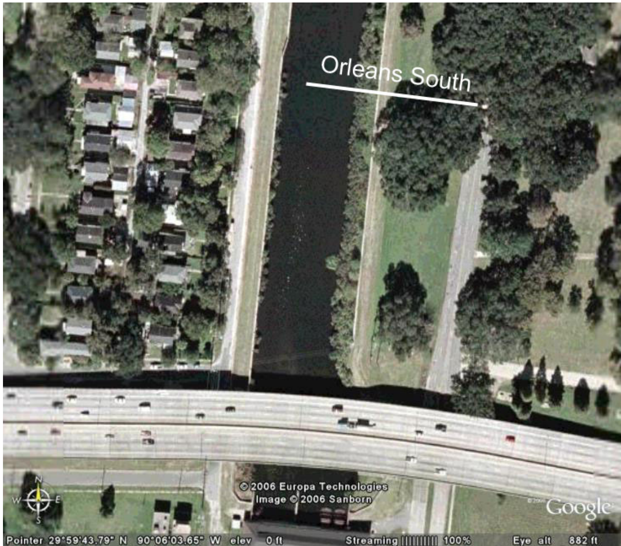
Figure 10-1. Aerial View of Orleans Avenue Canal – South (Station 8+61)
