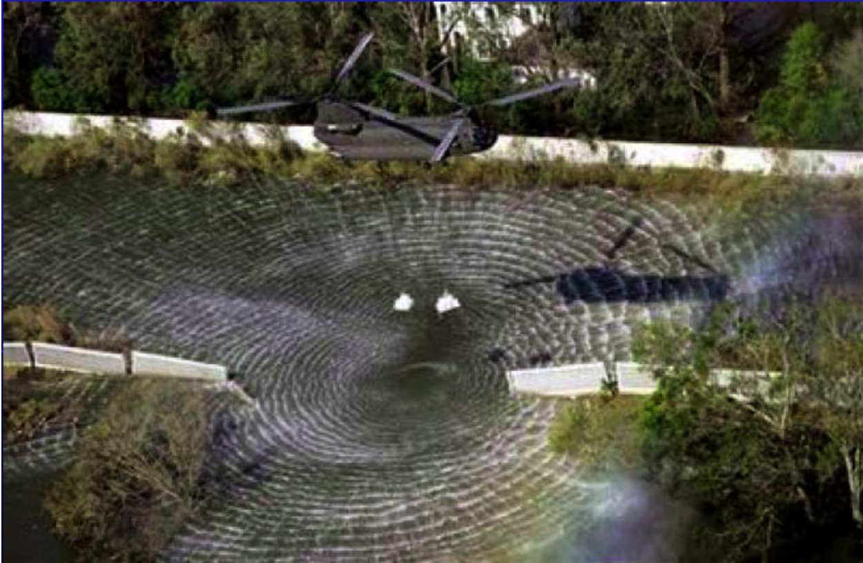
Figure 8-1. The South Breach at the London Avenue Canal Occurred at 6:00 AM to 7:00 AM on August 29, 2005. The breach, on the east side of the canal, was approximately 60 feet wide.
