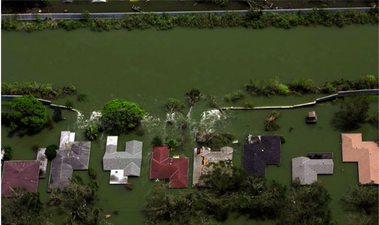
Figure 8-2. The North Breach at the London Avenue Canal Occurred at 7:00 AM to 8:00 AM on August 29, 2005. The breach, on the west side of the canal, is approximately 410 feet wide.
