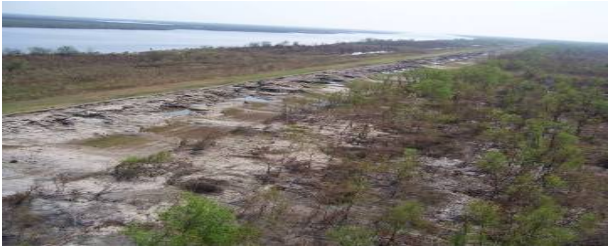
Figure 18. Example of levee breach along MRGO from overtopping and scour of erodible materials.
