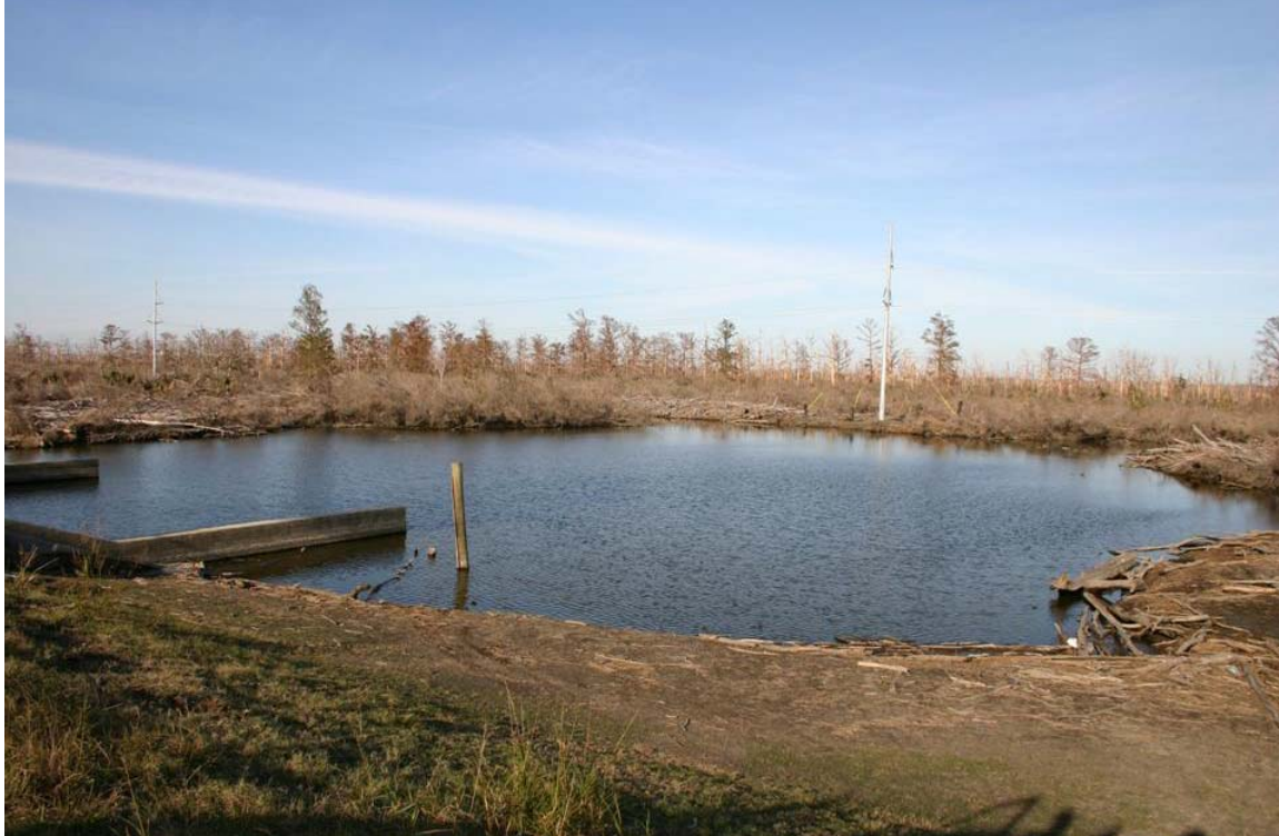
Figure 2. Pump Station Meraux #4 sampling station (pumped).
