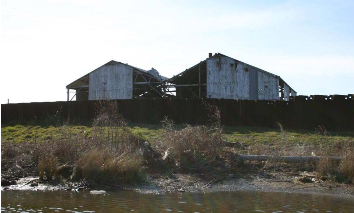
Figure 4. Pump Station Guichard #2 sampling station (did not pump).
