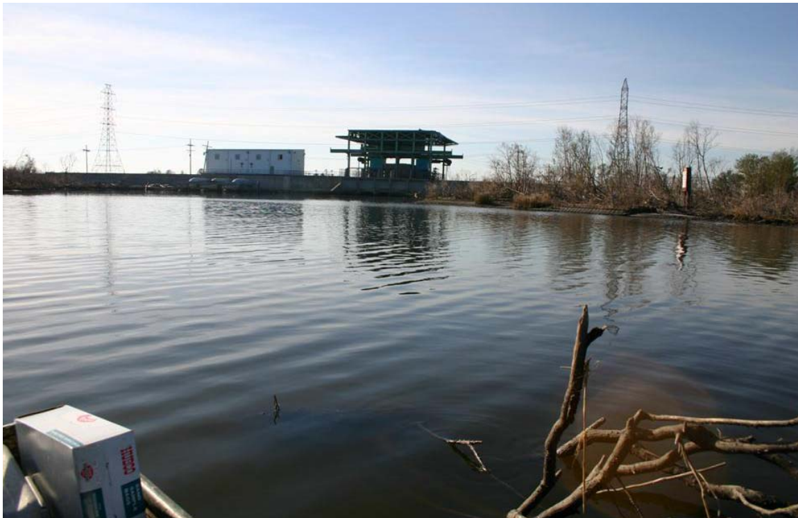
Figure 3. Pump Station Jean Lafitte #6 sampling station (pumped).
