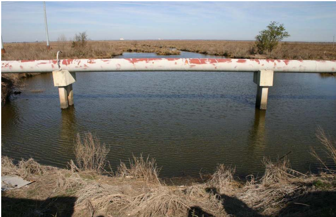
Figure 5. Pump Station Bayou Villere #3 sampling station (did not pump).
