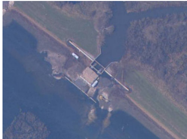
After Hurricane Katrina: Aerial view of the pump station
