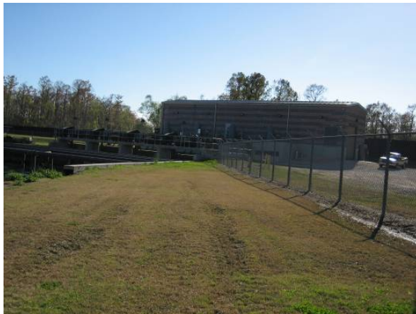
After Hurricane Katrina: View from the side
