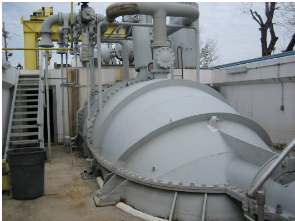
After Hurricane Katrina: View towards the discharge
