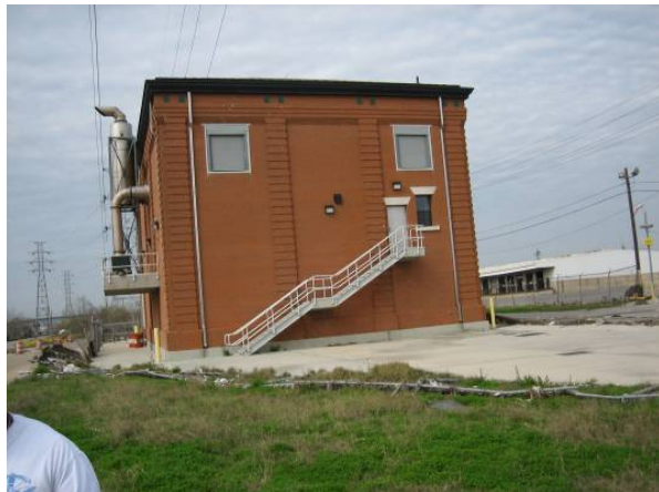
After Hurricane Katrina: View of the station
