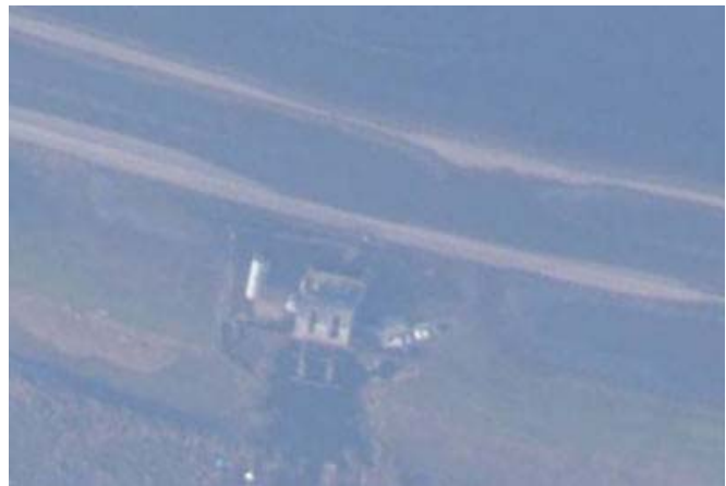
After Hurricane Katrina: Aerial view of the pump station
