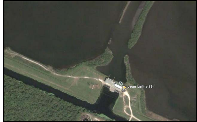
Before Hurricane Katrina: Aerial view of the pump station
