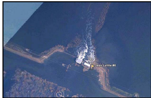
After Hurricane Katrina: Aerial view of the pump station
