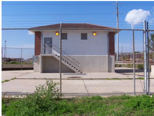
After Hurricane Katrina: View of the station
