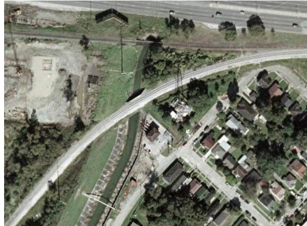
Before Hurricane Katrina: Aerial view of the pump station
