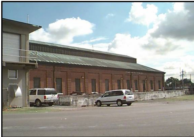
After Hurricane Katrina: View from the inlet canal
