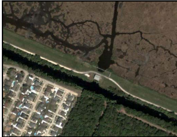
Before Hurricane Katrina: Aerial view of the pump station
