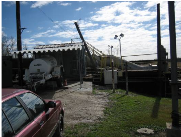
After Hurricane Katrina: View from the side
