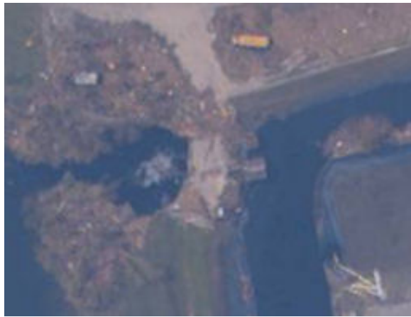
After Hurricane Katrina: Arial view of the pump station
