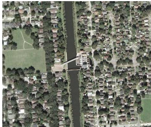
Before Hurricane Katrina: Aerial view of the pump station
