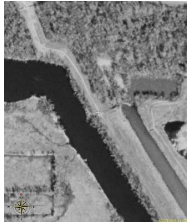
Before Hurricane Katrina: Aerial view of the pump station
