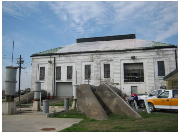
After Hurricane Katrina: View from the discharge
