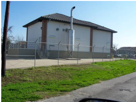
After Hurricane Katrina: View of the station
