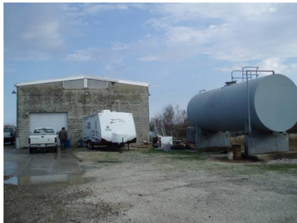
After Hurricane Katrina: View from the side
