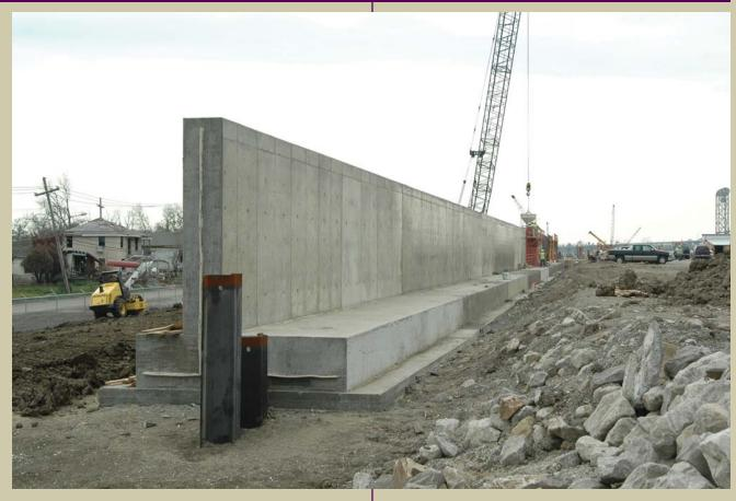
Katrina caused 50 major breaches in the hurricane protection system; 46 were due to overtopping and erosion. Four breaches occurred before water levels reached the top of the floodwalls and have been attributed to foundation failure.
