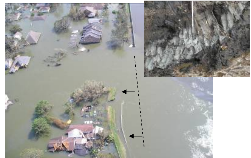
Displacement of wall and part of levee
