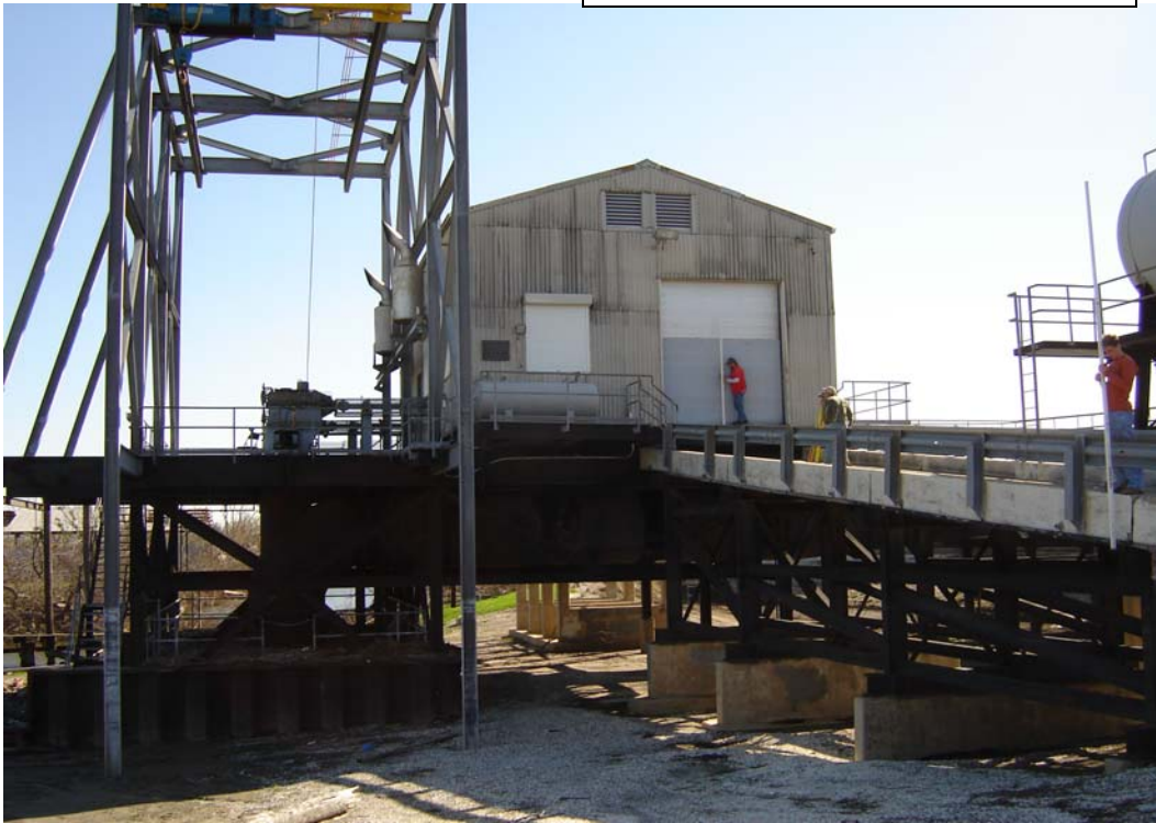
DUVIC(VENICE) PUMP STATION
