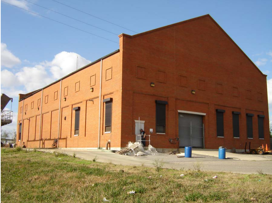
OP 11 PUMP STATION
