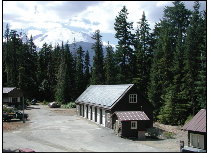
Mount Rainier National Park's solar-powered White River facility is similar to the one proposed at Ohana.
