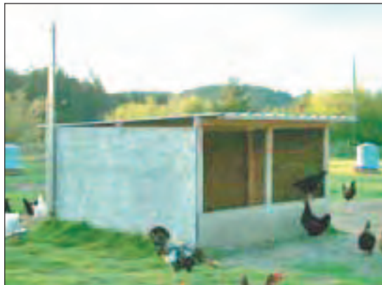
An electrified house. There are insulators near ground level. Chickens hop up to the top of the low front to get inside; predators have to climb. The mast at the back of the house allows the hot wire to come from overhead.
