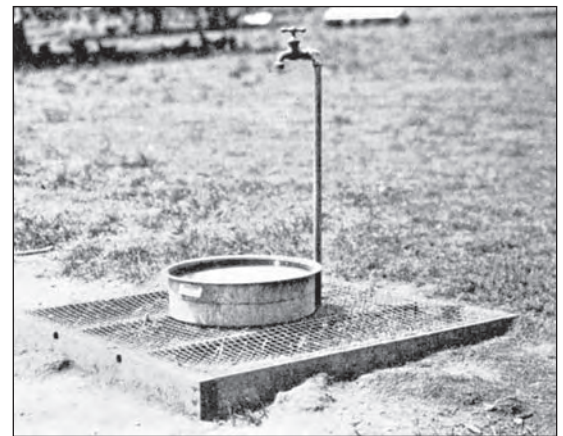
This installation from the 1930s uses a simple wire-covered platform to prevent wet spots.
